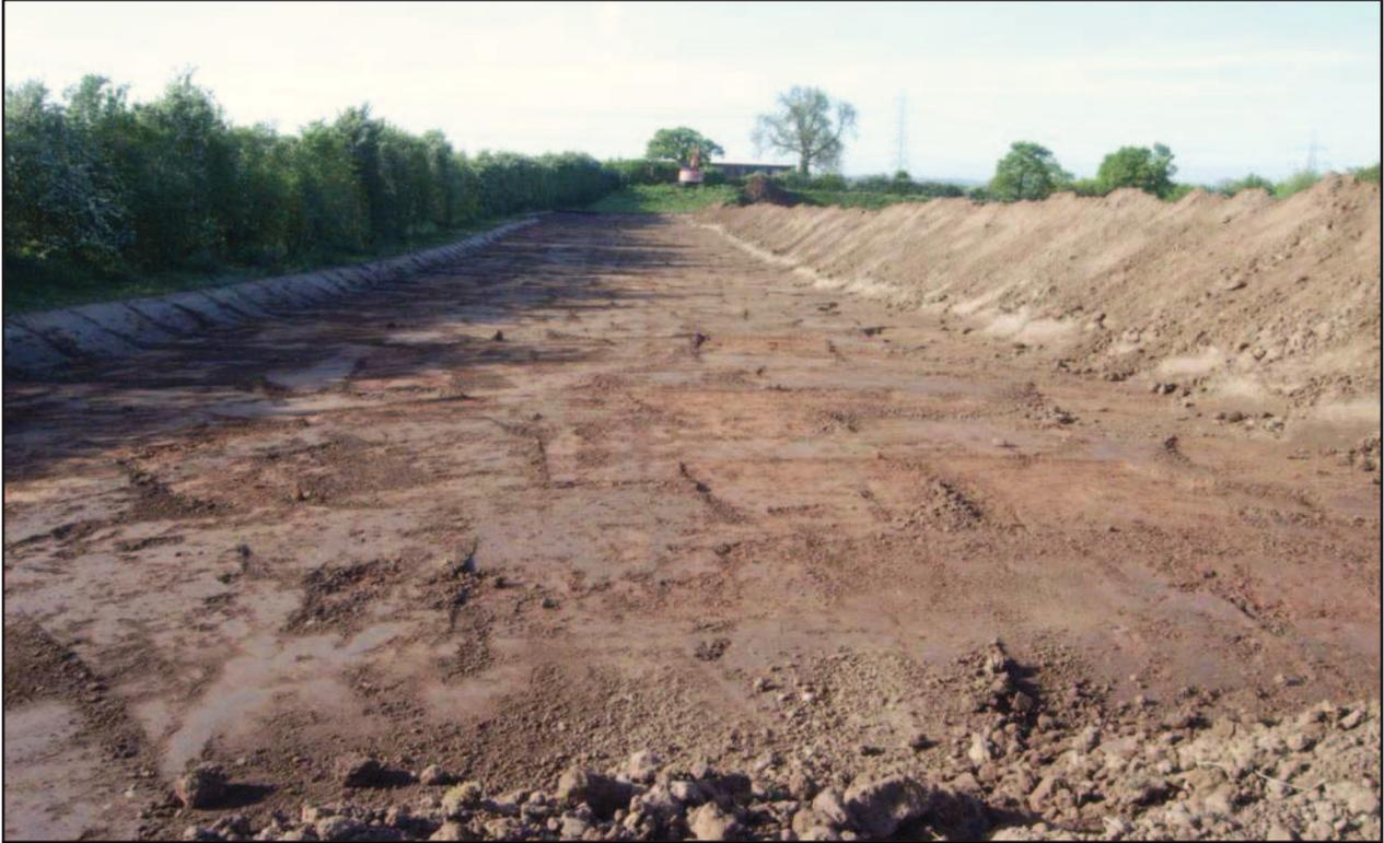
Plate 1: Topsoil strip for bund (looking south)
