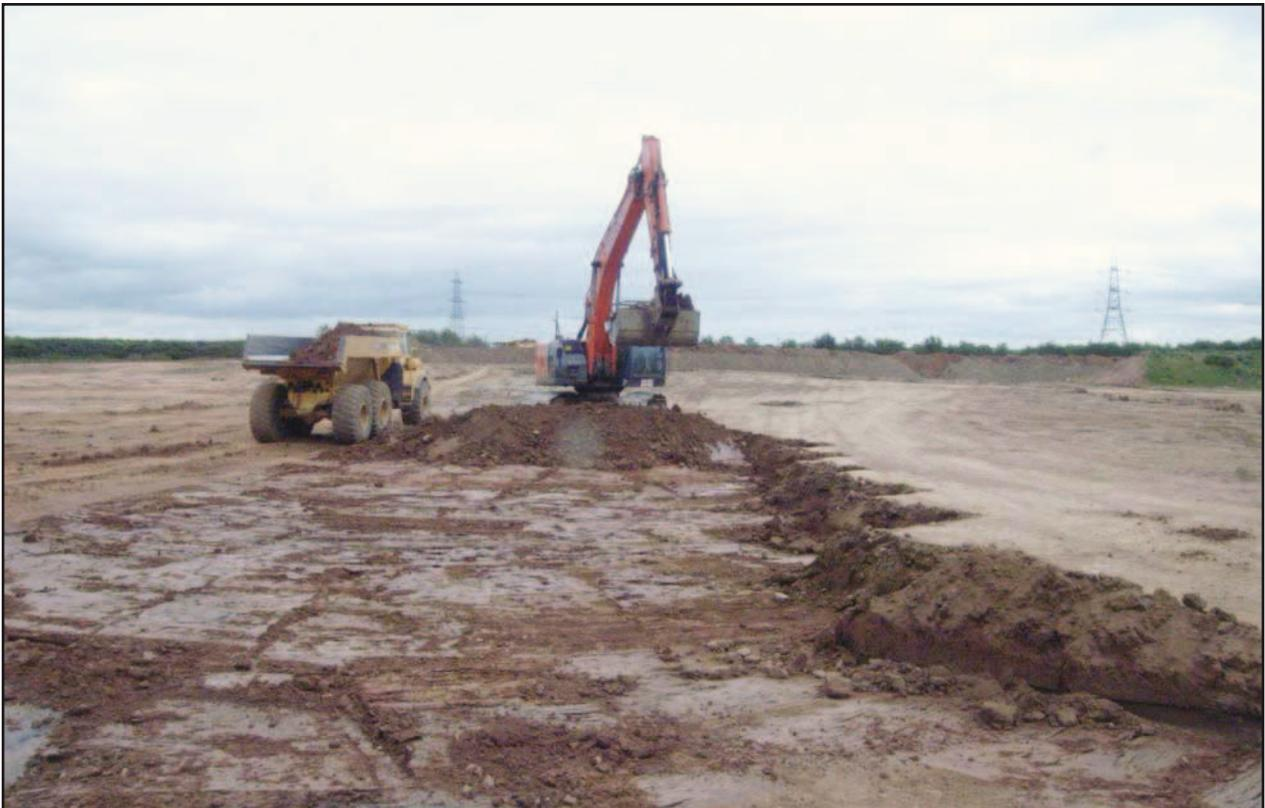
Plate 2: Subsoil strip for new building in progress (looking east)
