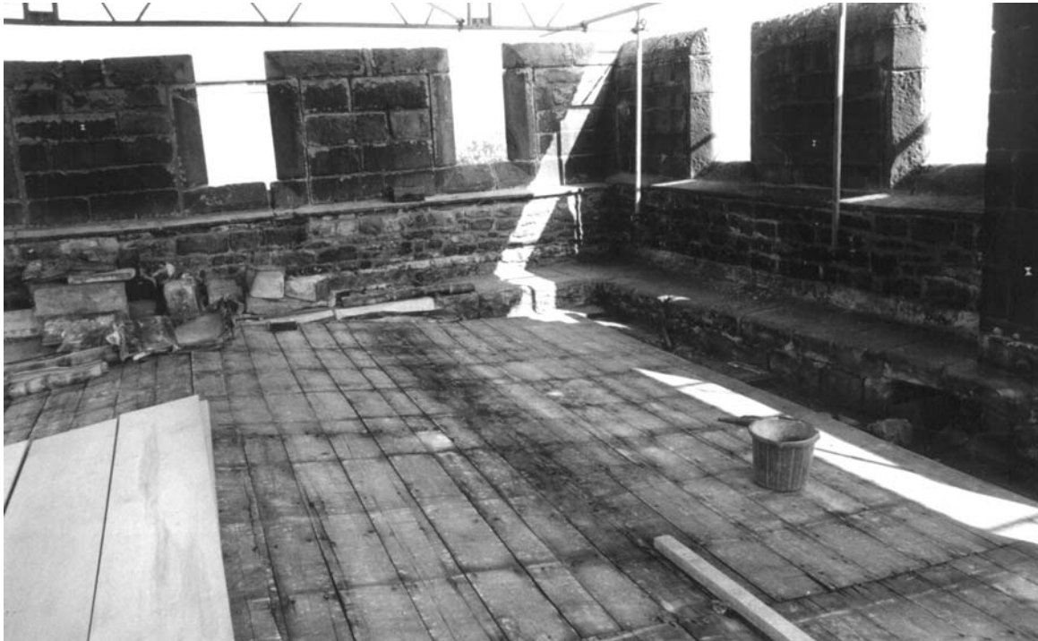
Plate 3 Roof of the Witches' Tower following stripping of the lead
