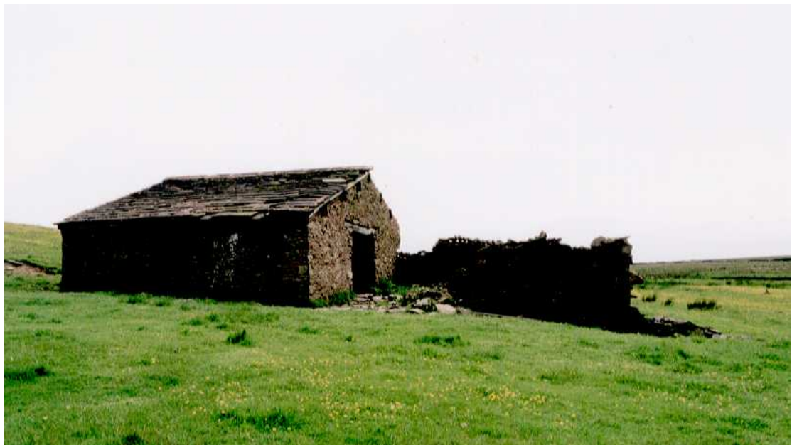
Fig 6 Photograph of field barn – Site 28
