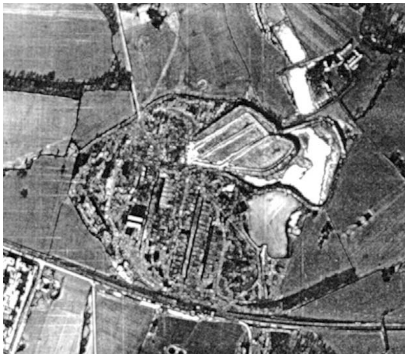
Plate 2: Vertical air photograph of the Plumley site, taken in 1946
