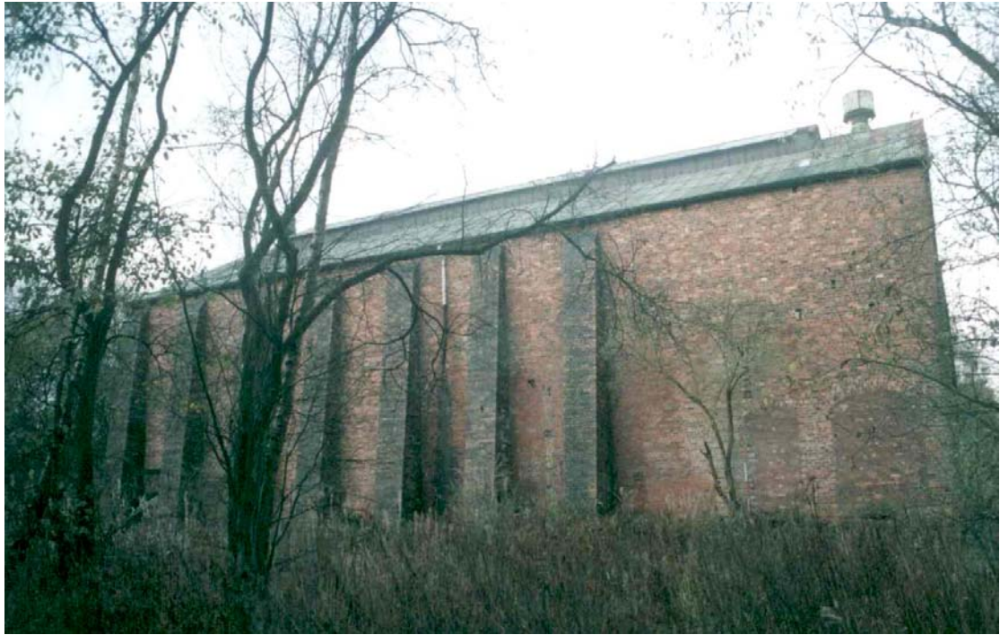
Plate 5: South external elevation of warehouse, showing blocked doorways and roof scars in the south-east corner
