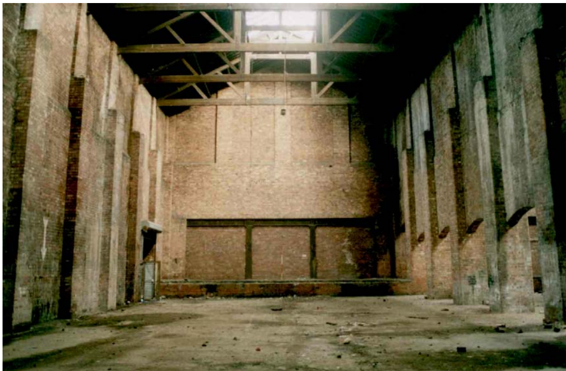
Plate 4: North-cell of the warehouse, showing bricked-up loading bays, looking east
