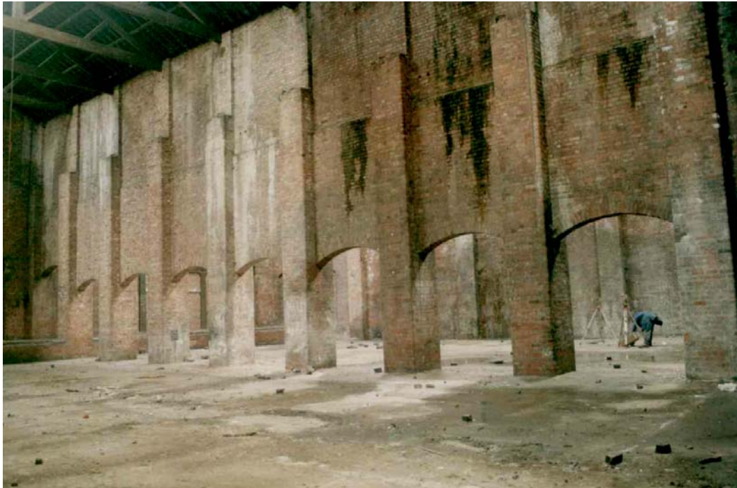
Plate 3: Central arched wall in the interior of the warehouse, looking south-east
