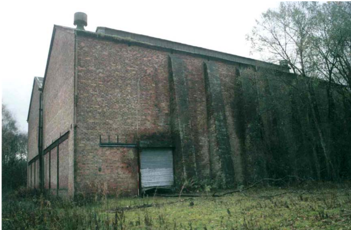
Plate 6: North and east elevations of the warehouse, showing shuttered door and bricked-up loading bays
