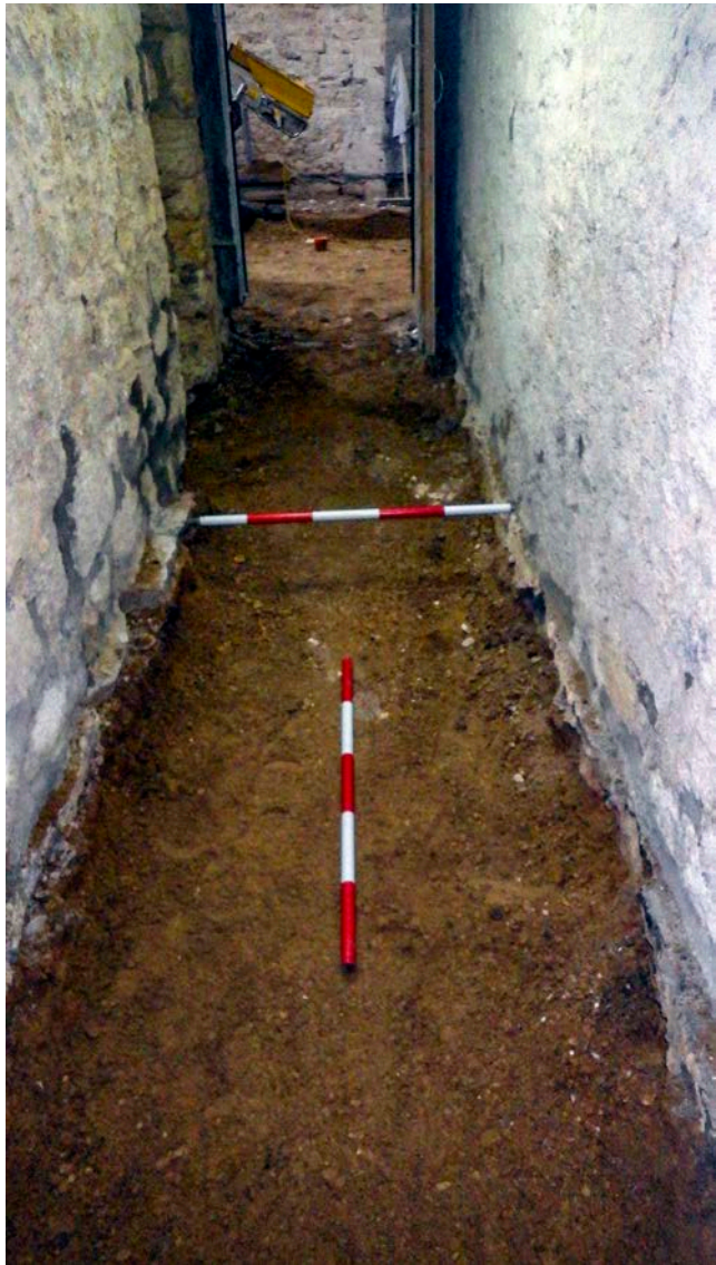
Plate 2: General shot of basement works
