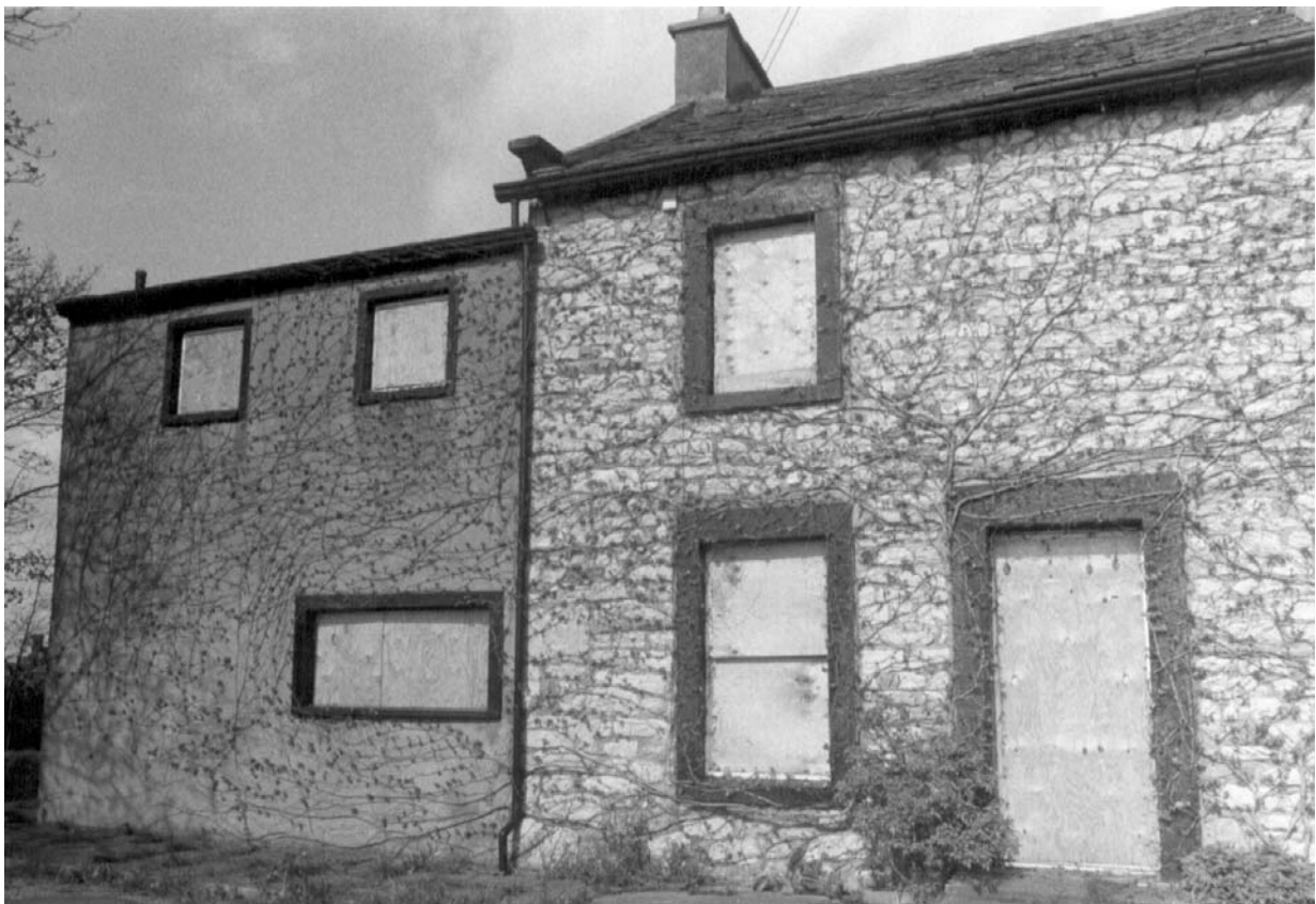
Plate 2: eastern elevation showing outbuilding extension
