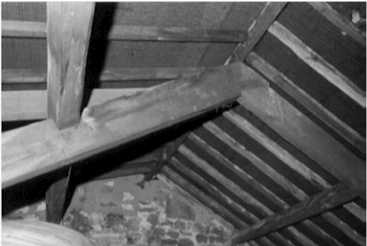
Plate 4: tie-beam pine roof truss in the attic
