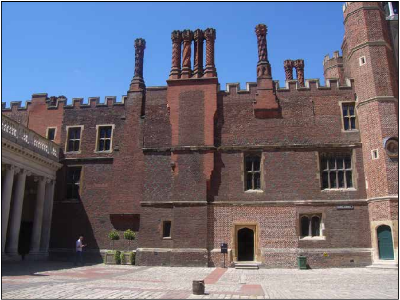
Plate 13: General view of east facing elevations of Clock Court, looking west
