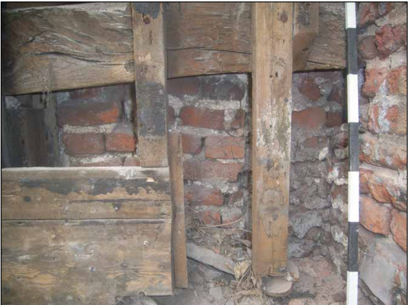
Plate 48: Earlier structure under east side of Roof 1, looking north
