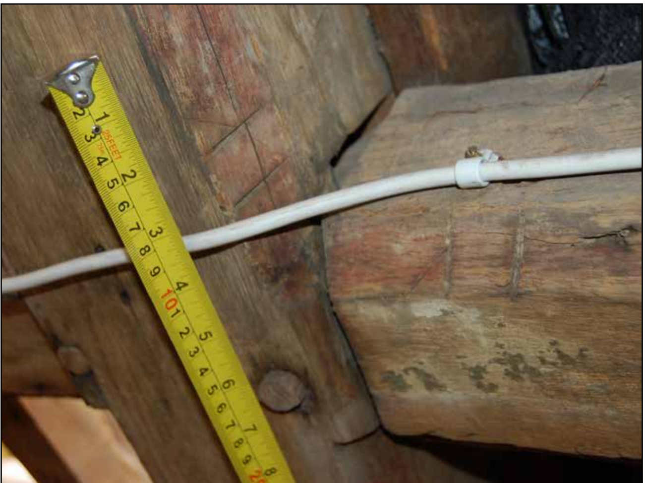
Plate 68: Detail of carpenter's marks on the east principal rafter and purlin of Truss 2, Roof 2
