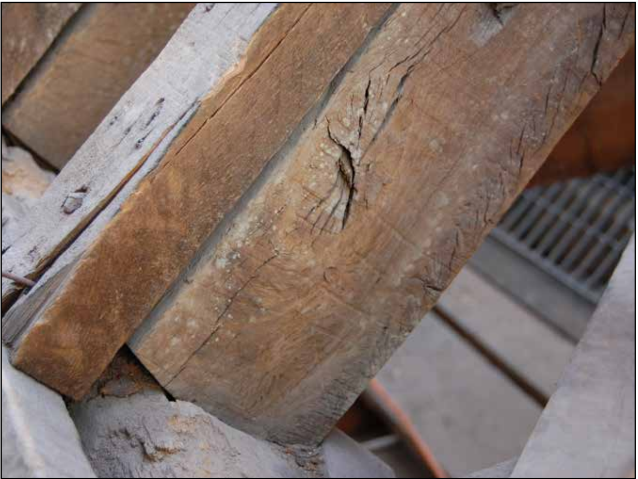
Plate 61: Detail of common rafter in Bay 3, Roof 2, looking north
