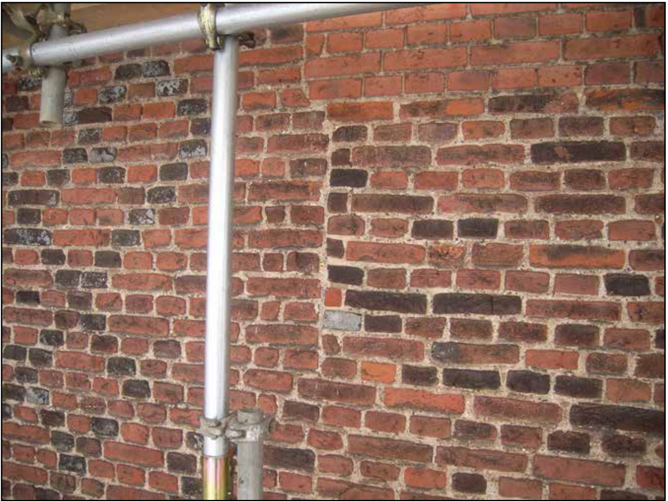
Plate 5: Base Court - West facing Elevation Part 1, upper parapet, looking north east
