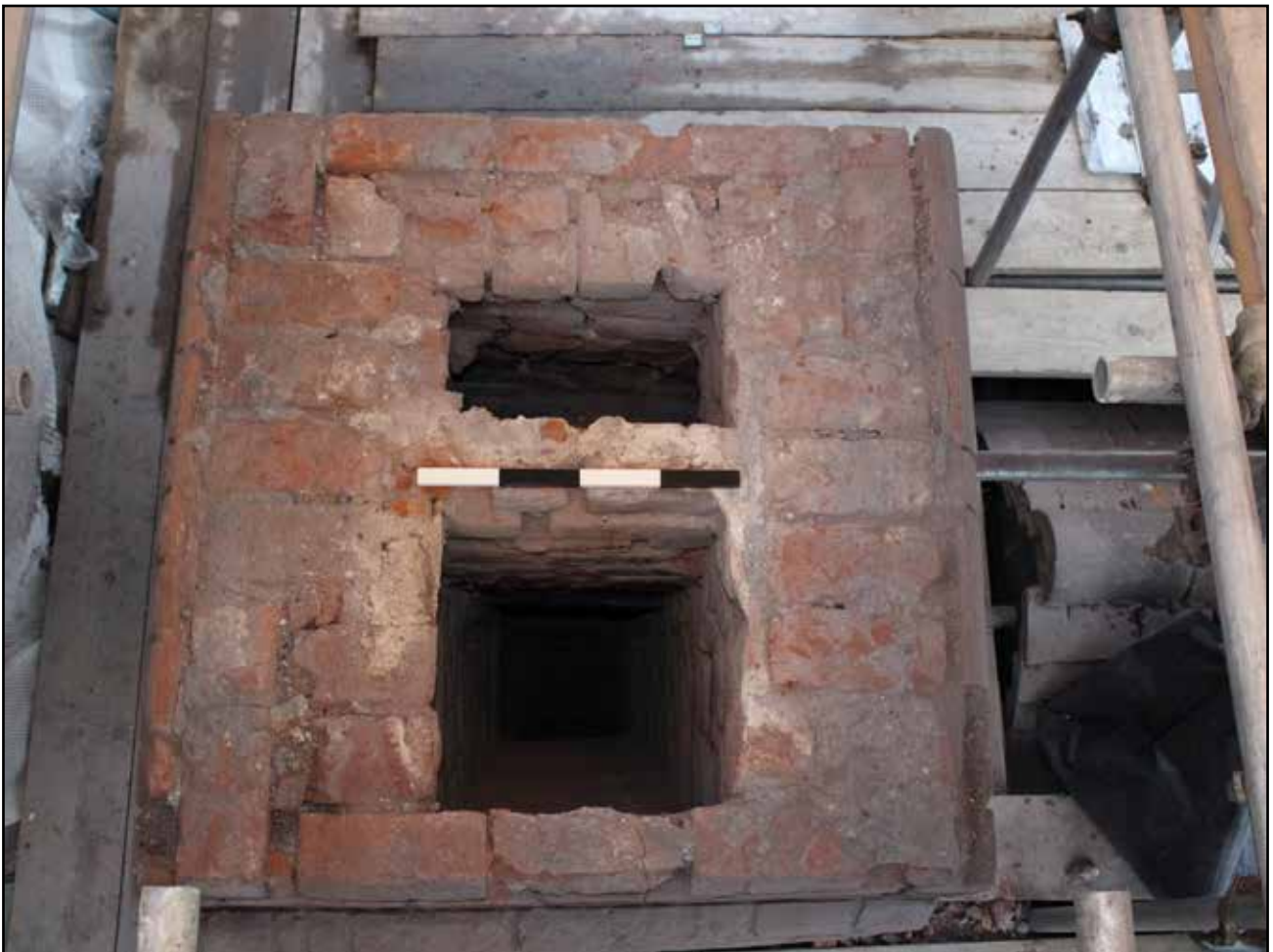
Plate 32: Chimney E243, Interior during deconstruction
