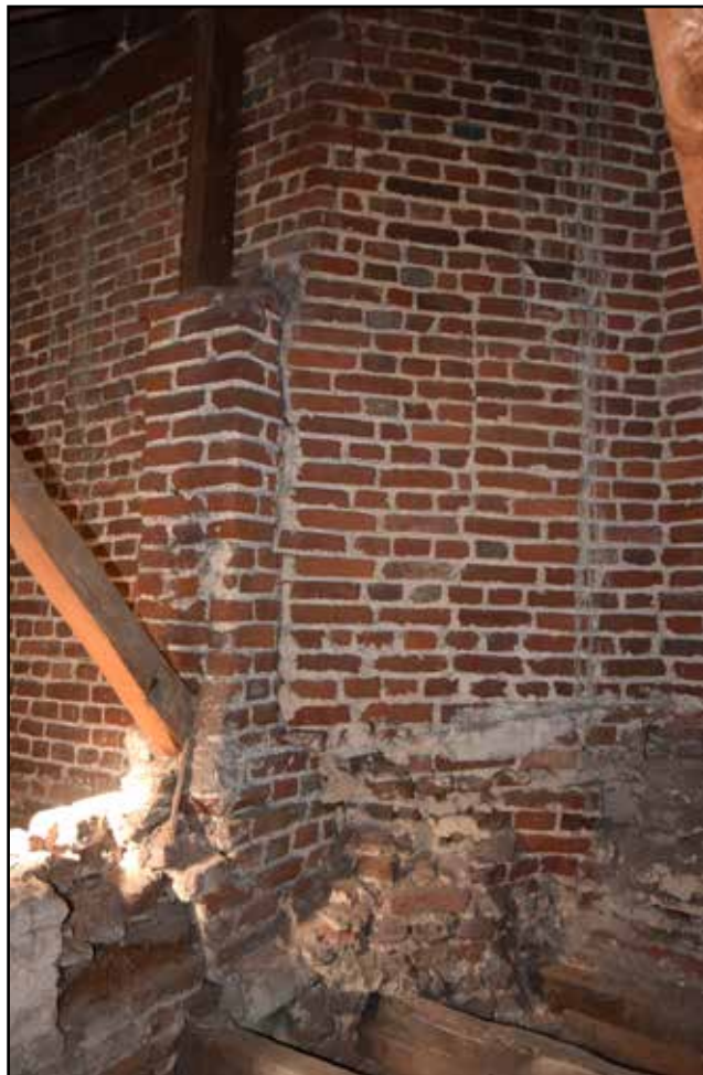
Plate 34: Roof 4 north west elevation, east space, looking north west
