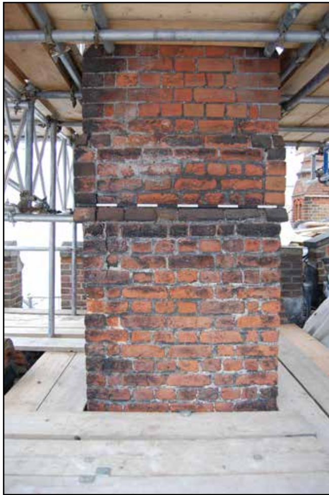
Plate 31: Chimney E243, Looking west
