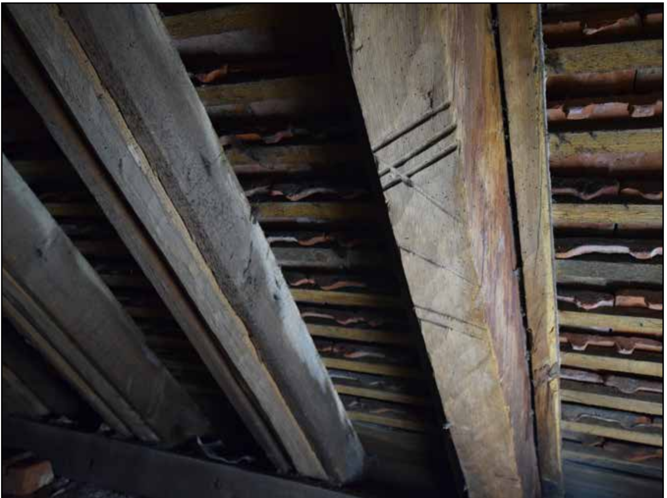
Plate 74: Baltic mark on lower rafter,Lean-to roof structure of Roof 4, looking south
