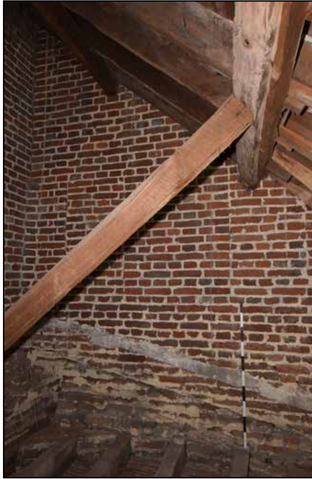
Plate 37: Roof 4 east elevation, east space, looking east
