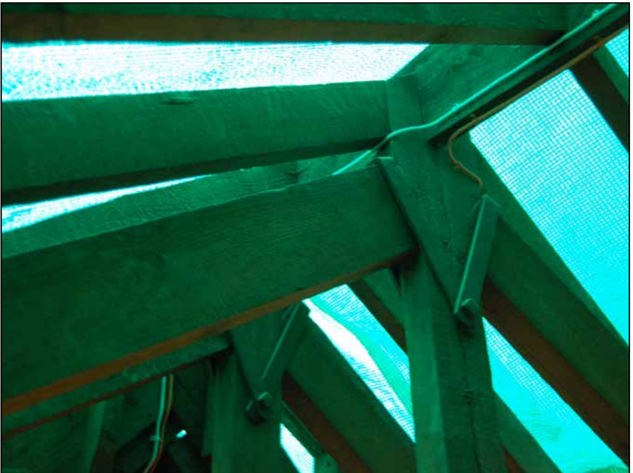
Plate 46: Details of Trusses 1 and 2, Roof 1, looking south west
