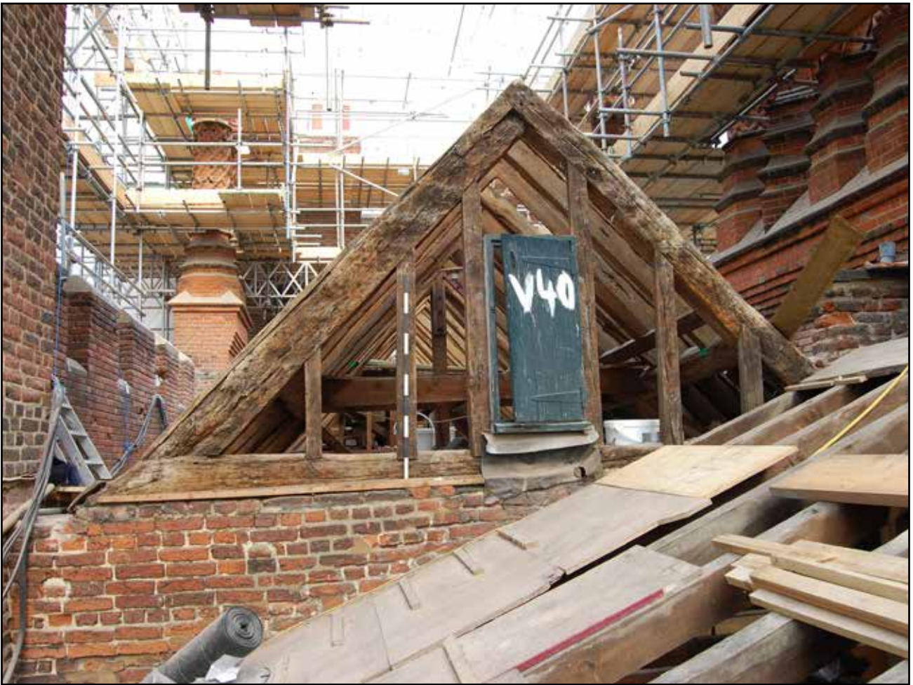
Plate 51: Roof 2, looking north
