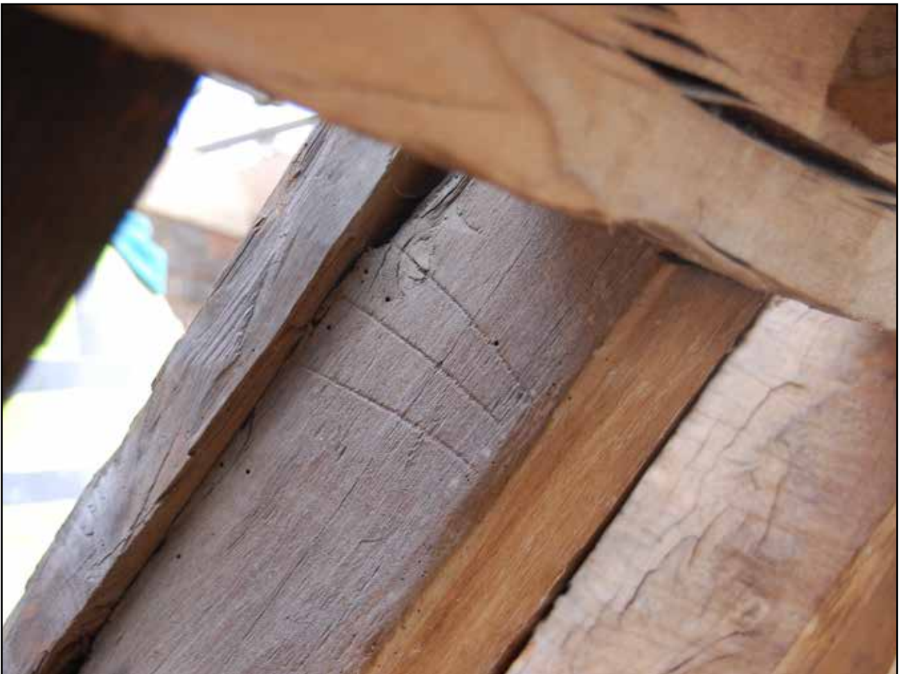
Plate 64: Detail of common rafter in Bay 2, Roof 2, looking south east
