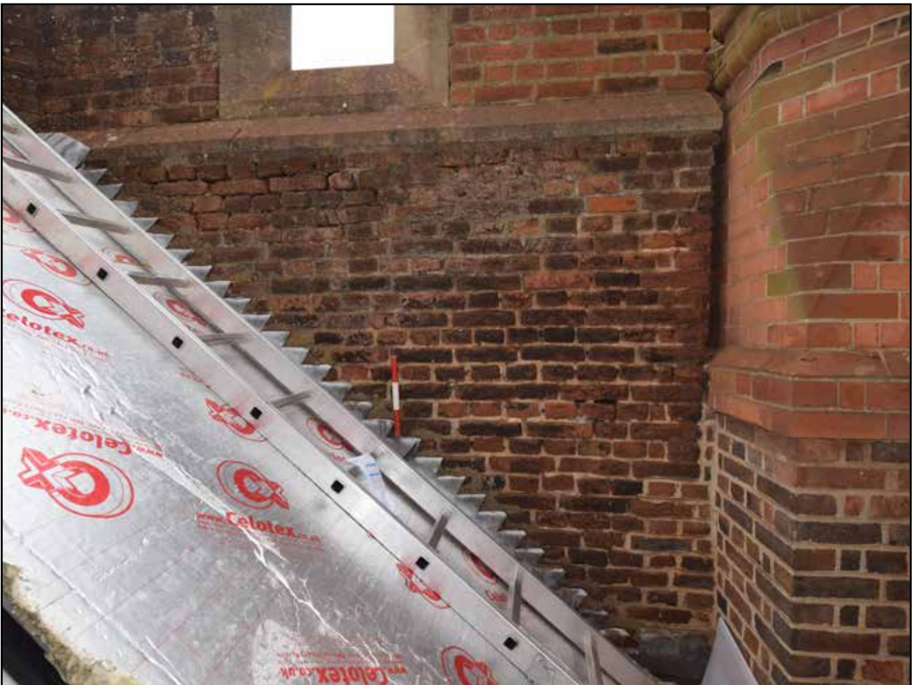
Plate 38: Exterior parapet level of Roof 4 east elevation, east space, looking east
