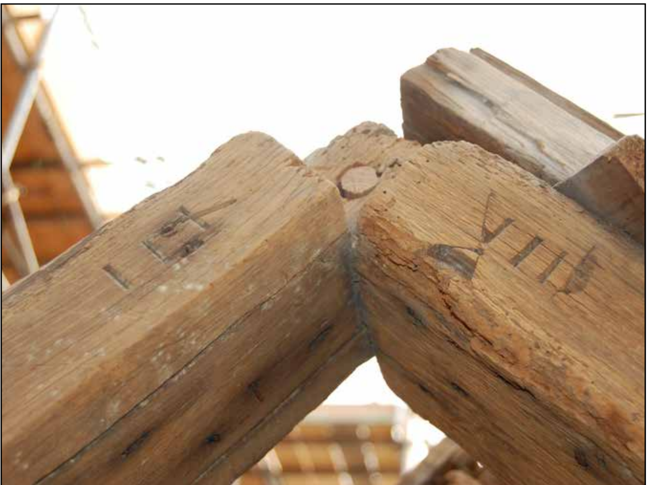
Plate 66: Detail of carpenter's marks in south face of common rafters, Bay 2, Roof 2
