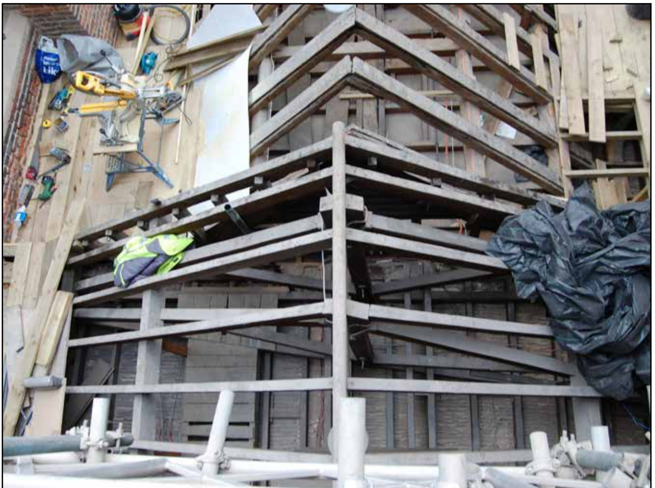
Plate 44: Roof 1 from above
