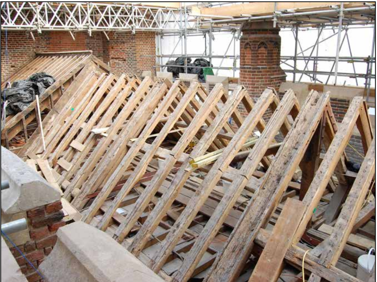
Plate 50: Roof 2, looking north east
