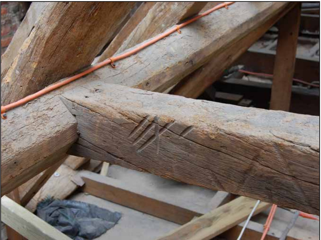
Plate 70: Baltic mark on north face of intermediary collar in Bay 1, Roof 2
