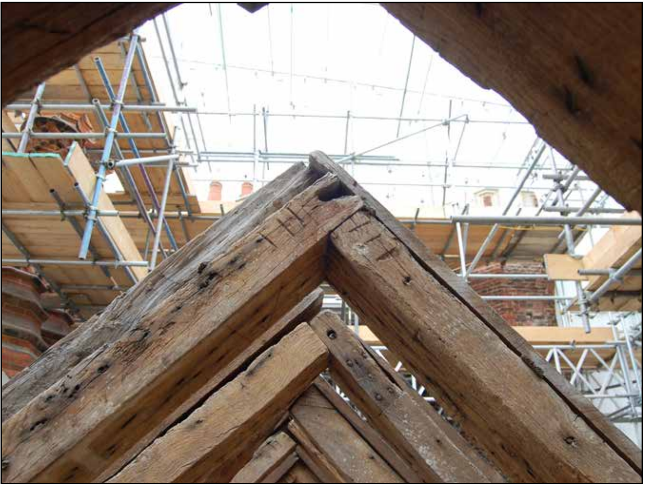
Plate 65: Detail of carpenter's marks in south face of common rafters, Bay 2, Roof 2
