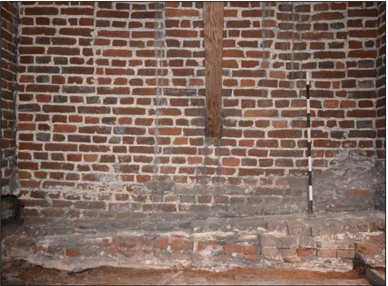
Plate 43: Roof 4 north elevation, west space, looking north
