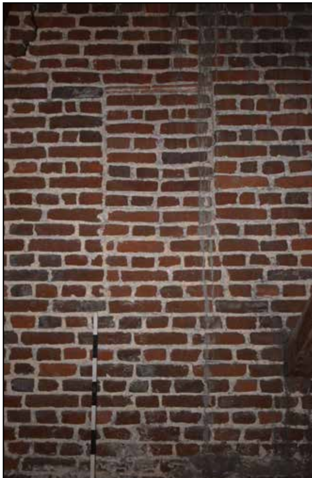
Plate 36: Detail of Roof 4 north elevation, west space, looking north
