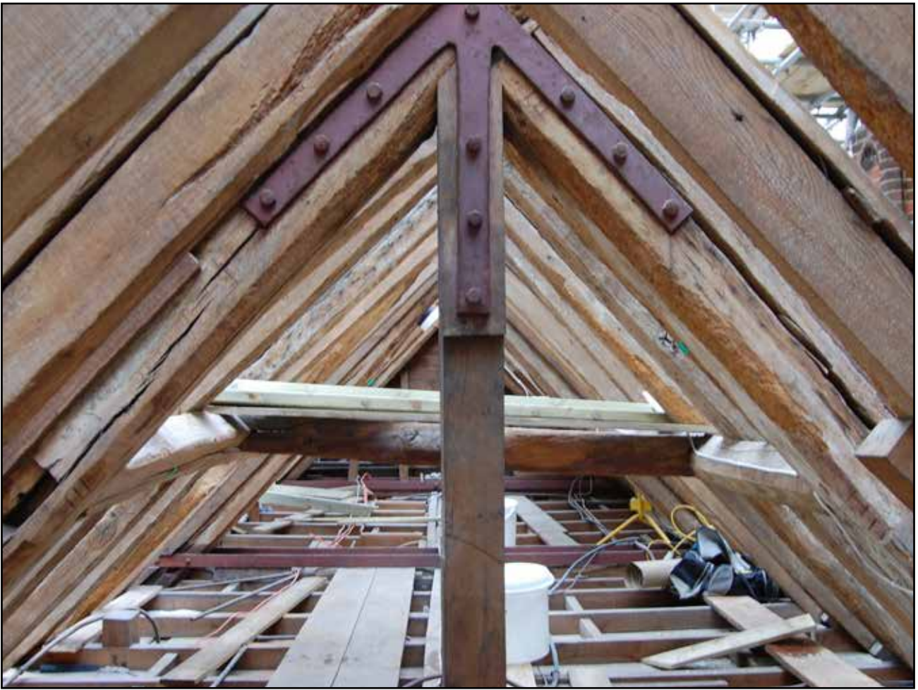
Plate 71: 20th century modification to Truss 3, Roof 2, looking north
