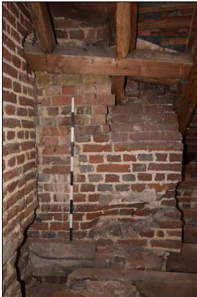
Plate 42: Roof 4, Chimney E242, looking south
