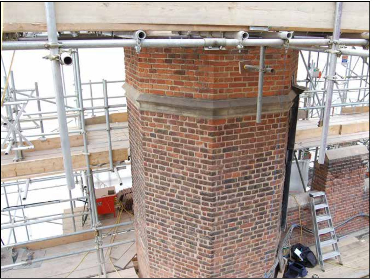
Plate 11: Upper section of Base Court Turret, looking north west
