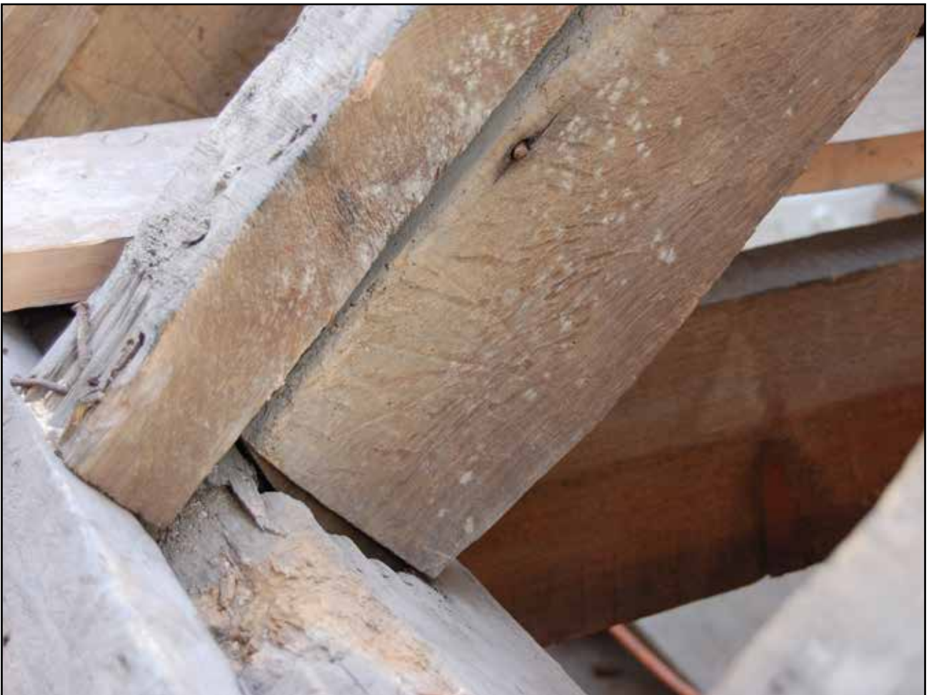
Plate 62: Detail of common rafter in Bay 3, Roof 2, looking north
