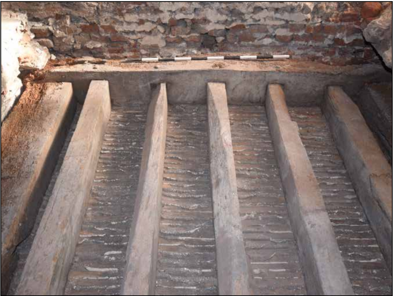
Plate 75 : Lower roof structure in west space, Roof 4, looking east
