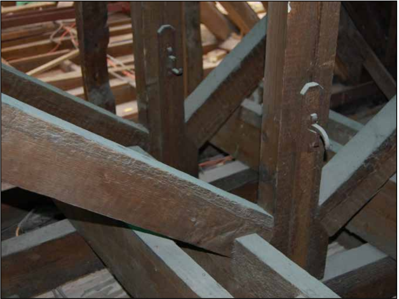
Plate 45: Details of Trusses 1 and 2, Roof 1, looking south west
