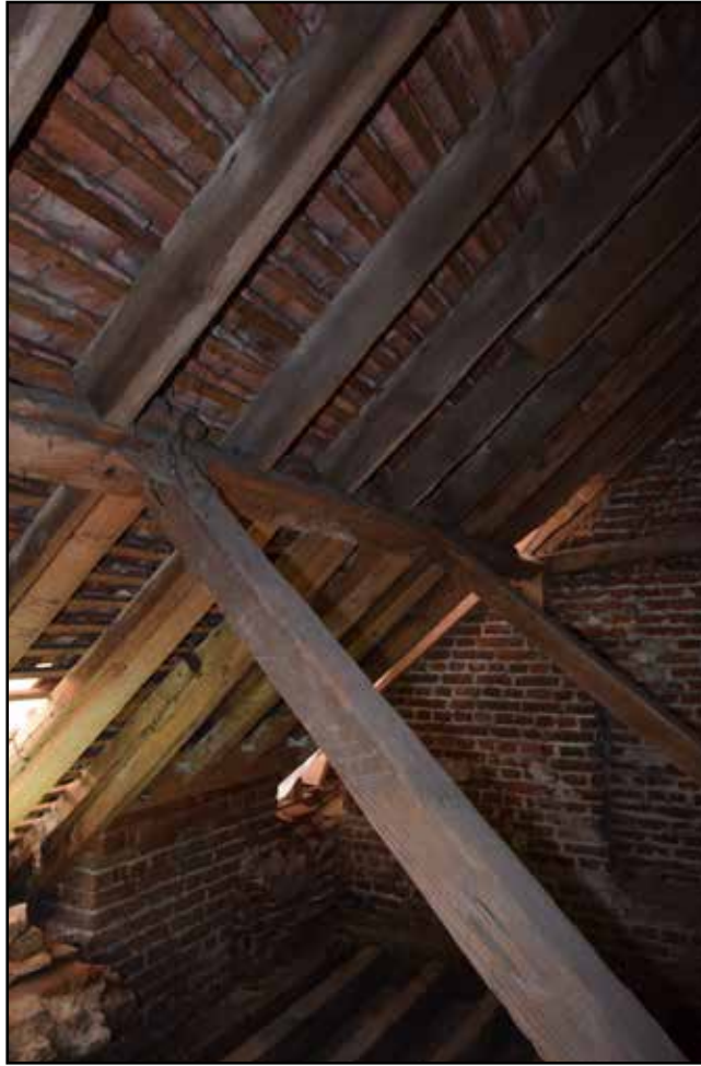
Plate 73 : Lean-to roof structure of Roof 4, looking south west
