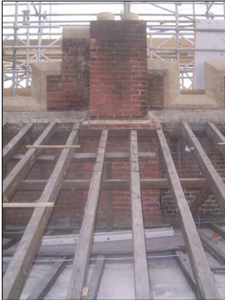
Plate 17: General view of Clock Court - East Facing Elevation Part 1, inner parapet
