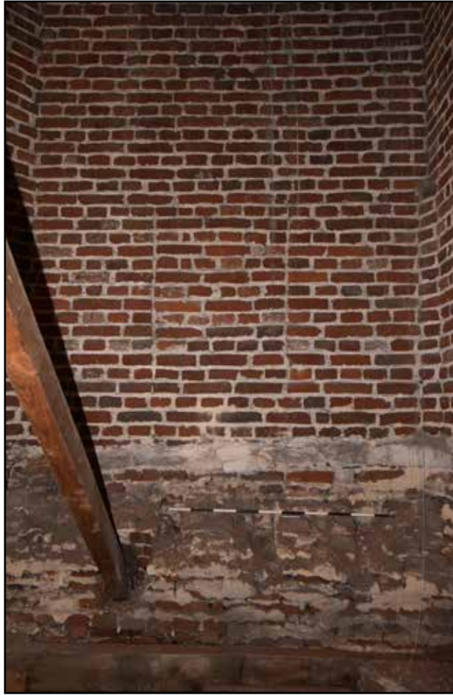
Plate 35: Roof 4 north elevation, east space, looking north
