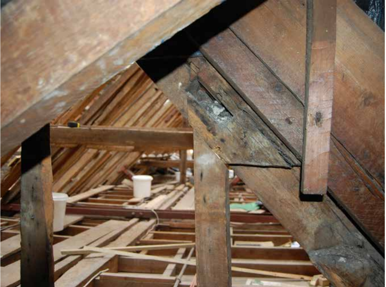
Plate 56: Detail of west principal rafter in Truss 1, Roof 2, looking south west
