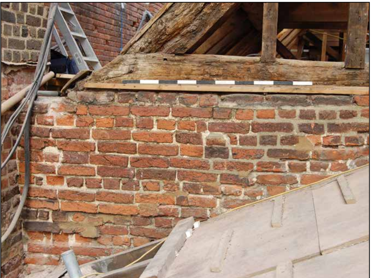
Plate 52: Wall plate of south end of Roof 2, looking north
