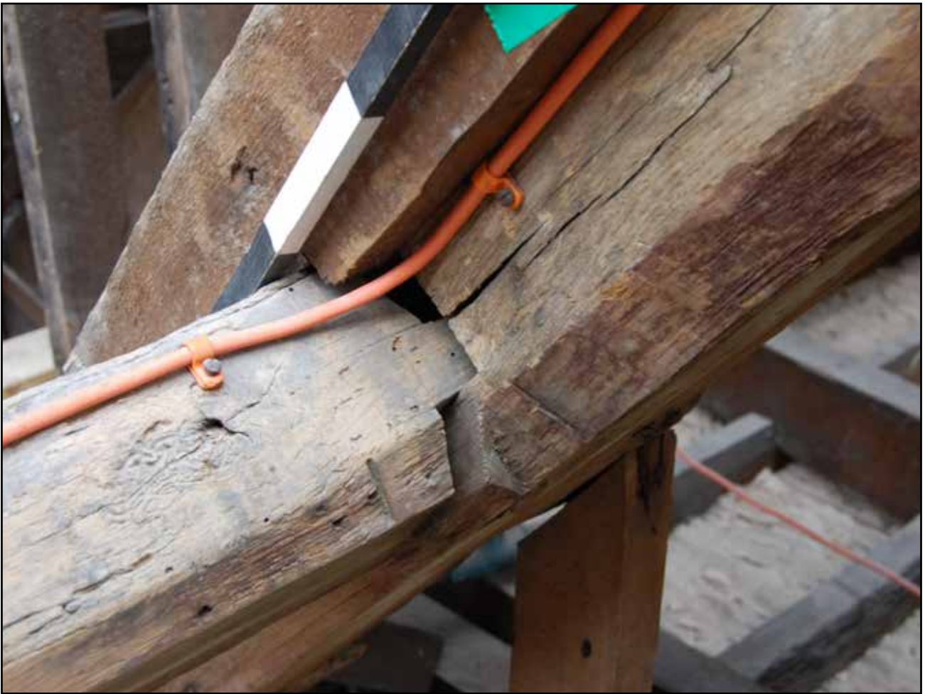
Plate 53: Purlin and west principal rafter of Truss 1, Roof 2, looking north west
