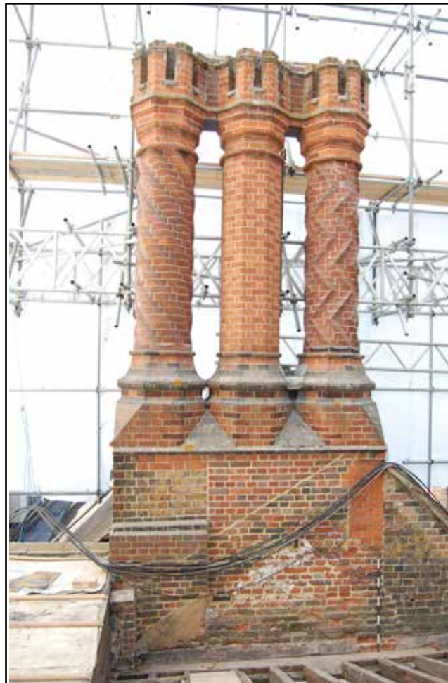
Plate 10: Chimney breast that supports chimneys E251, E252 and E253, looking west
