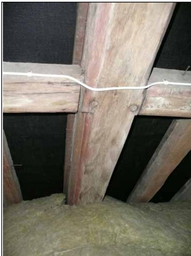
Plate 54: Painted principal rafter, Roof 2, looking east
