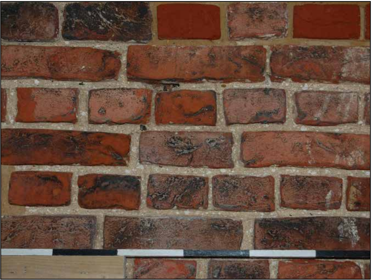
Plate 3: Base Court - West facing Elevation Part 1, detail of primary brickwork (A)
