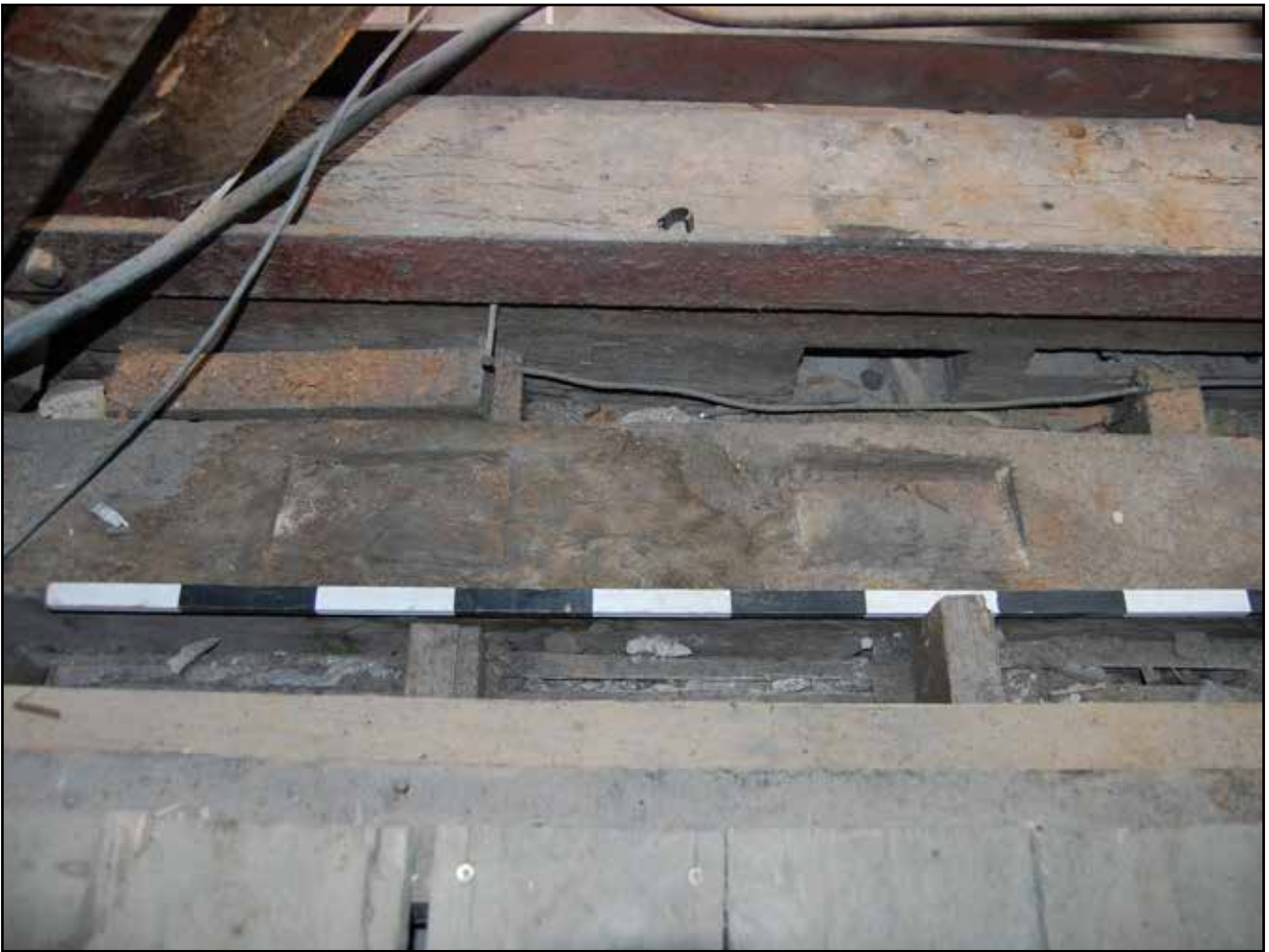
Plate 49: Notches for rafter feet in earlier wall plate under Roof 1
