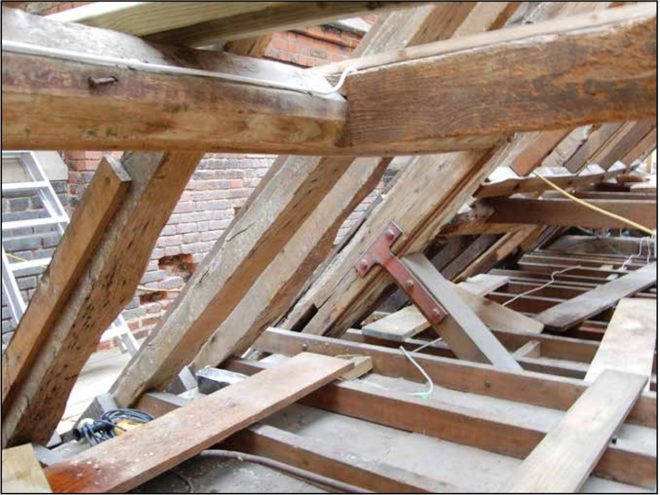
Plate 55: Painted purlin, Roof 2, looking south east
