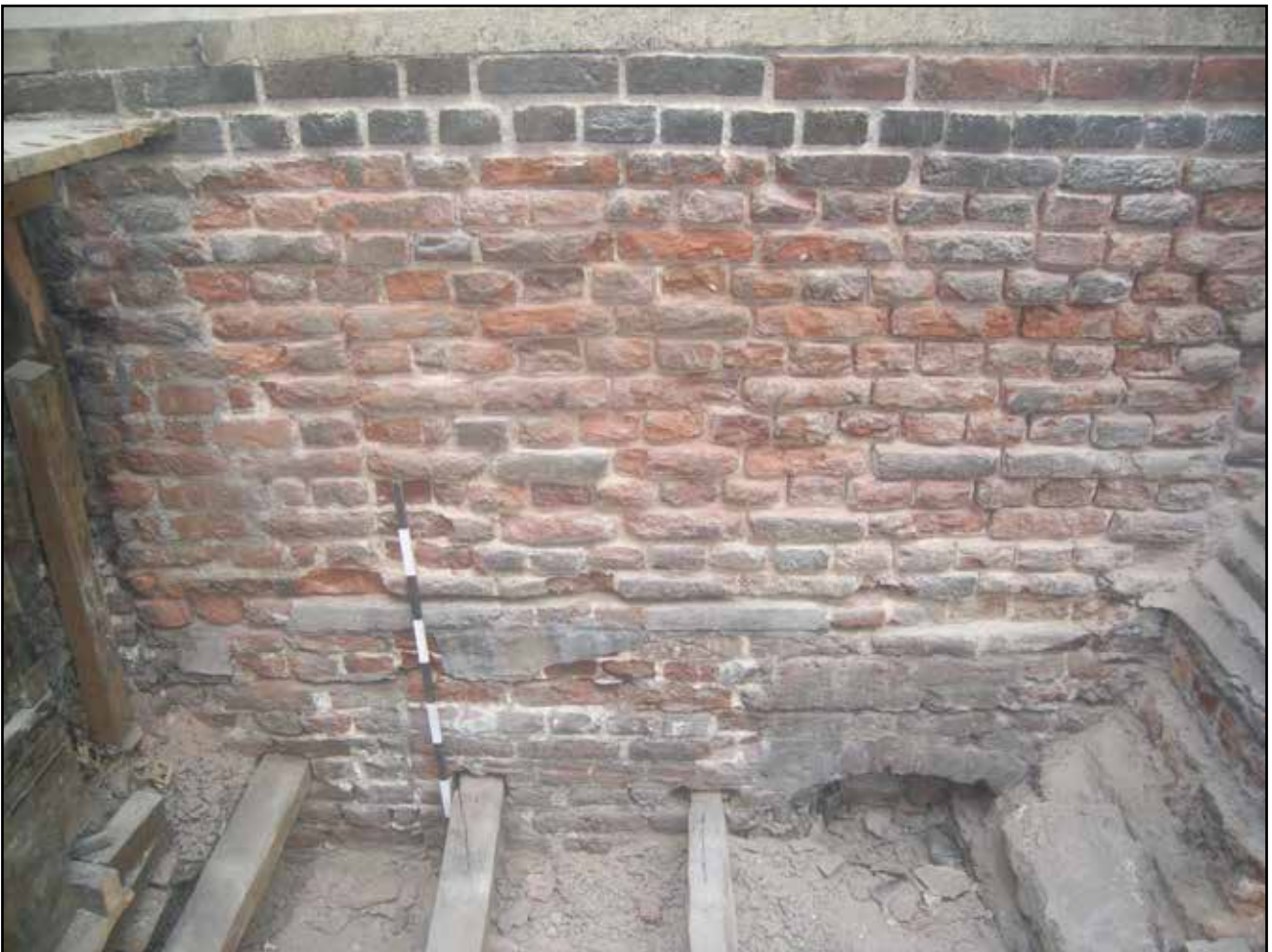
Plate 26: Inner parapet, East Facing Elevation Part 2, Clock Court, looking east
