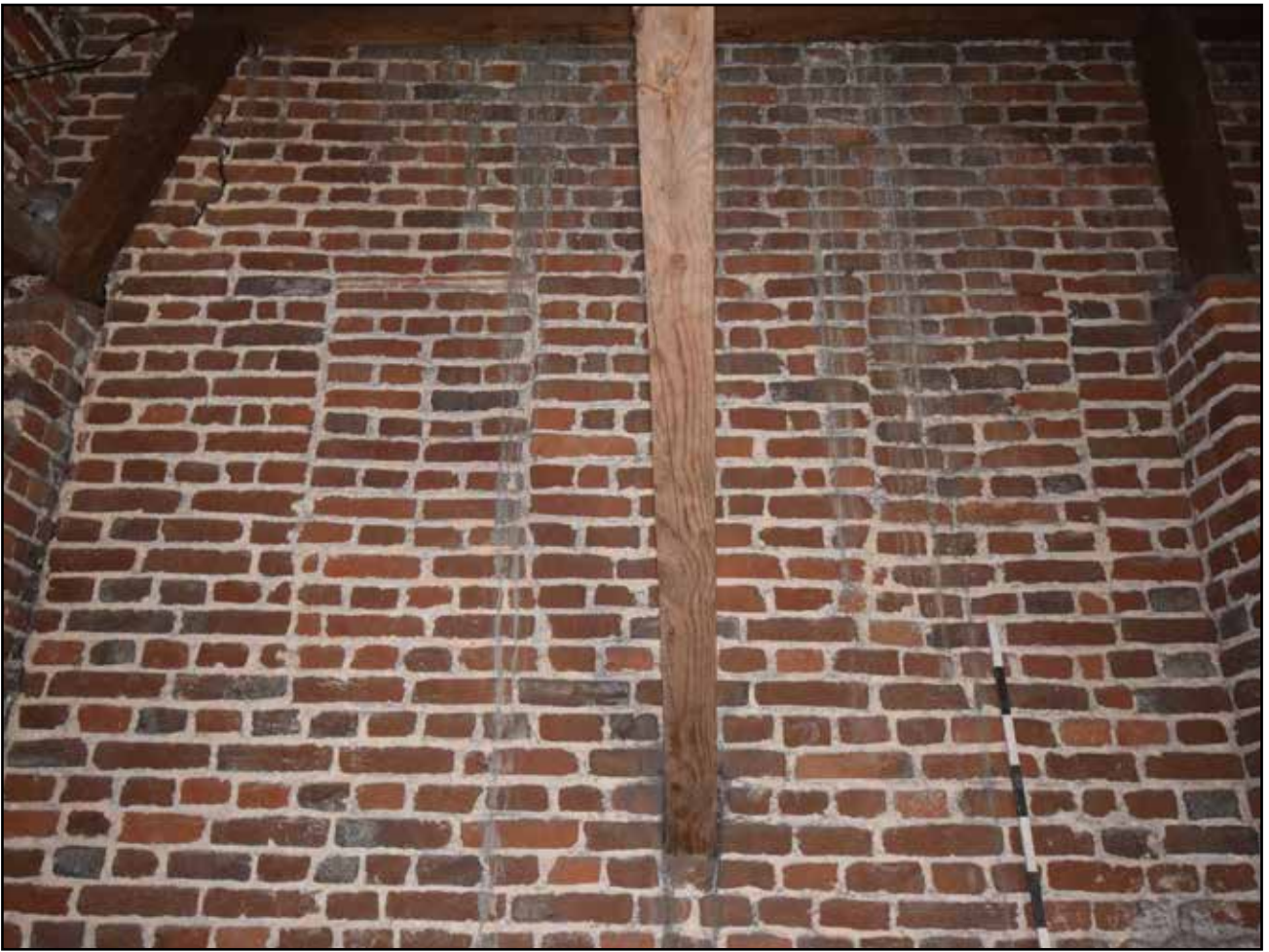
Plate 33: Roof 4 north elevation, west space, looking north
