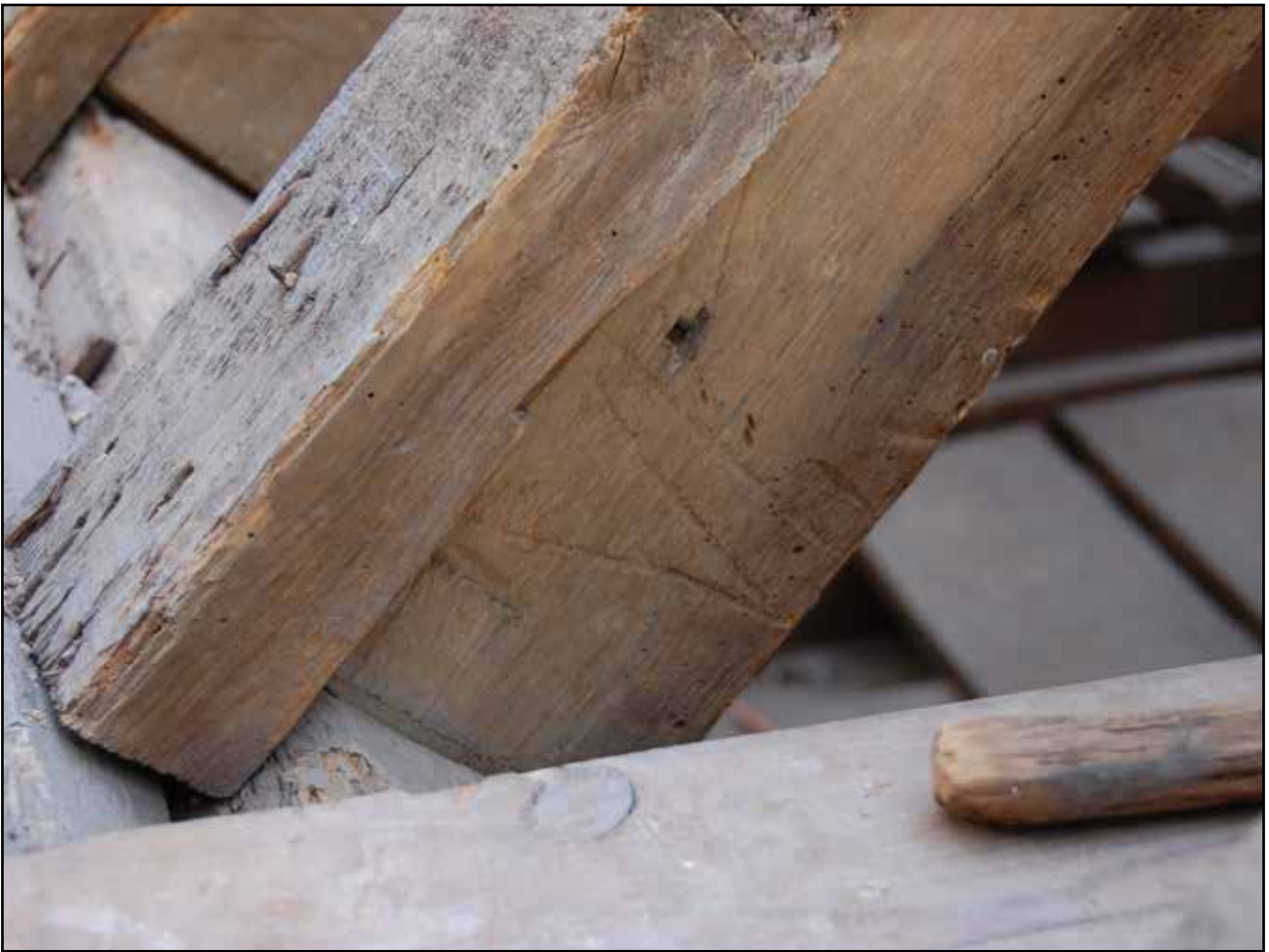
Plate 63: Detail of common rafter in Bay 3, Roof 2, looking north west
