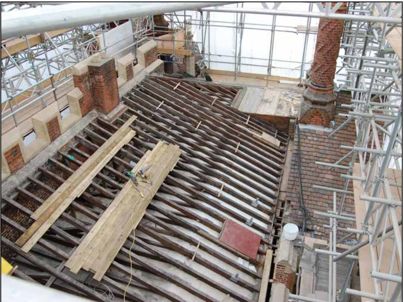
Plate 72: General view of Roof 3, looking south east
