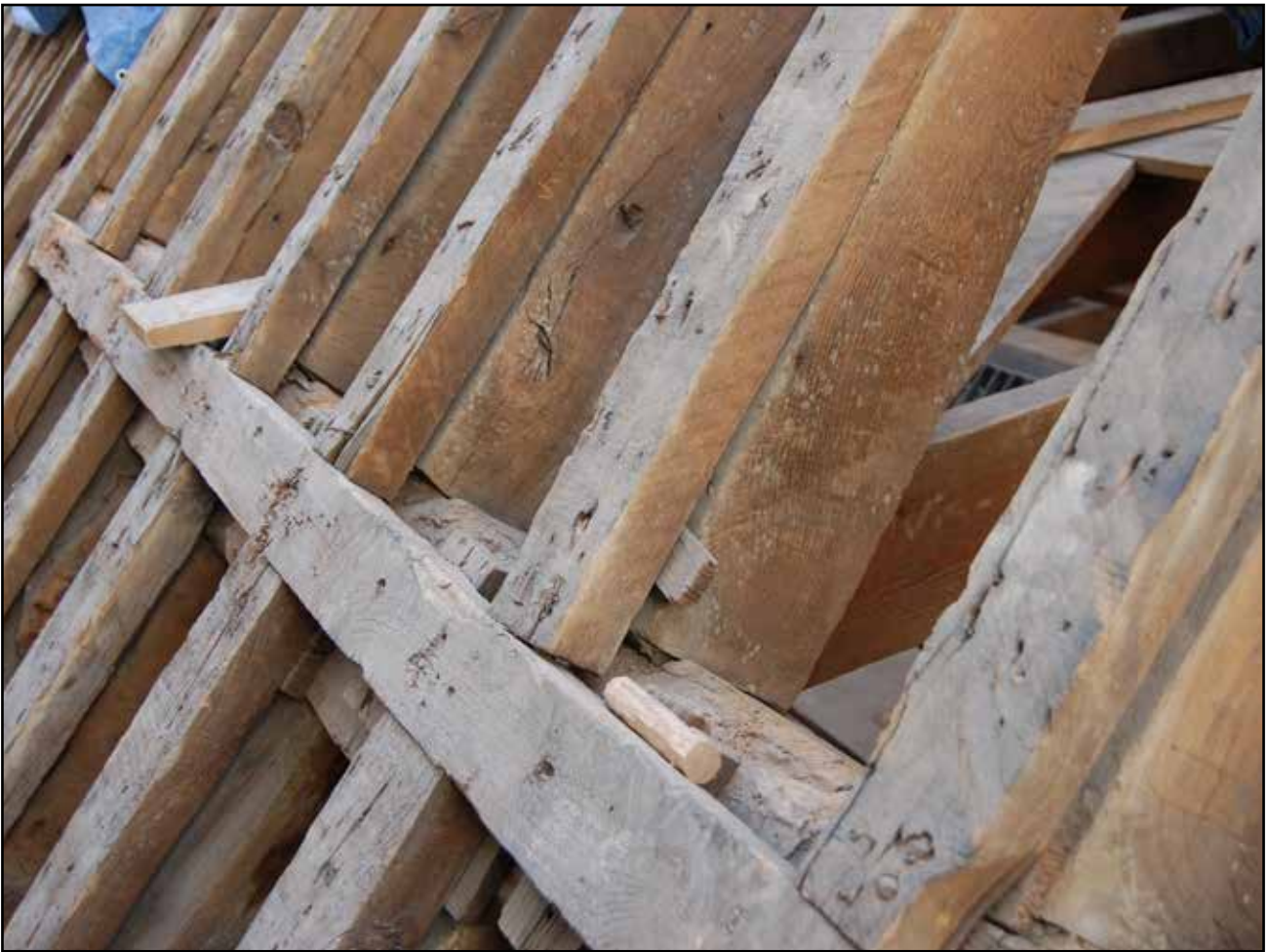
Plate 59 : West common rafters of Bay 3, Roof 2, looking north east
