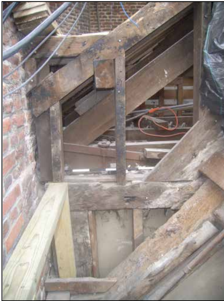
Plate 47: Earlier structure under west side of Roof 1, looking north
