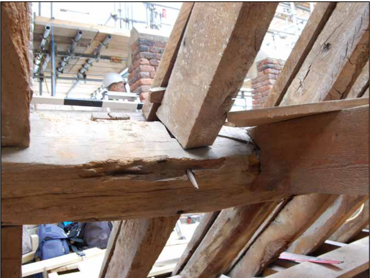
Plate 60: Detail of common rafter in Bay 3, Roof 2, looking north
