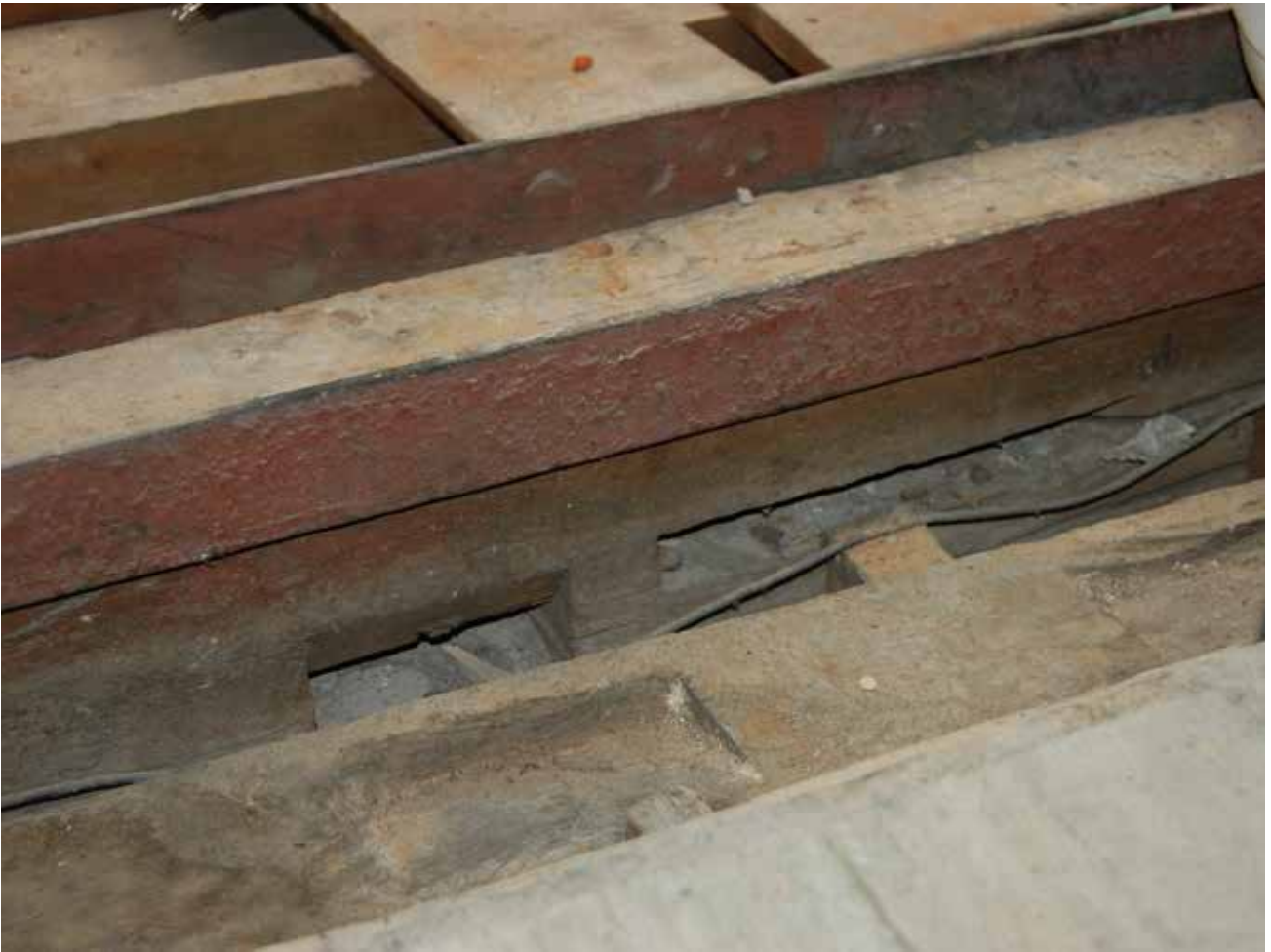
Plate 57: Detail of tie beam in Truss 1, Roof 2, looking north east
