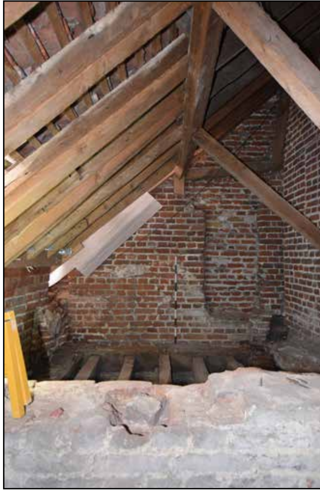
Plate 39: Roof 4 west elevation, west space, looking west
