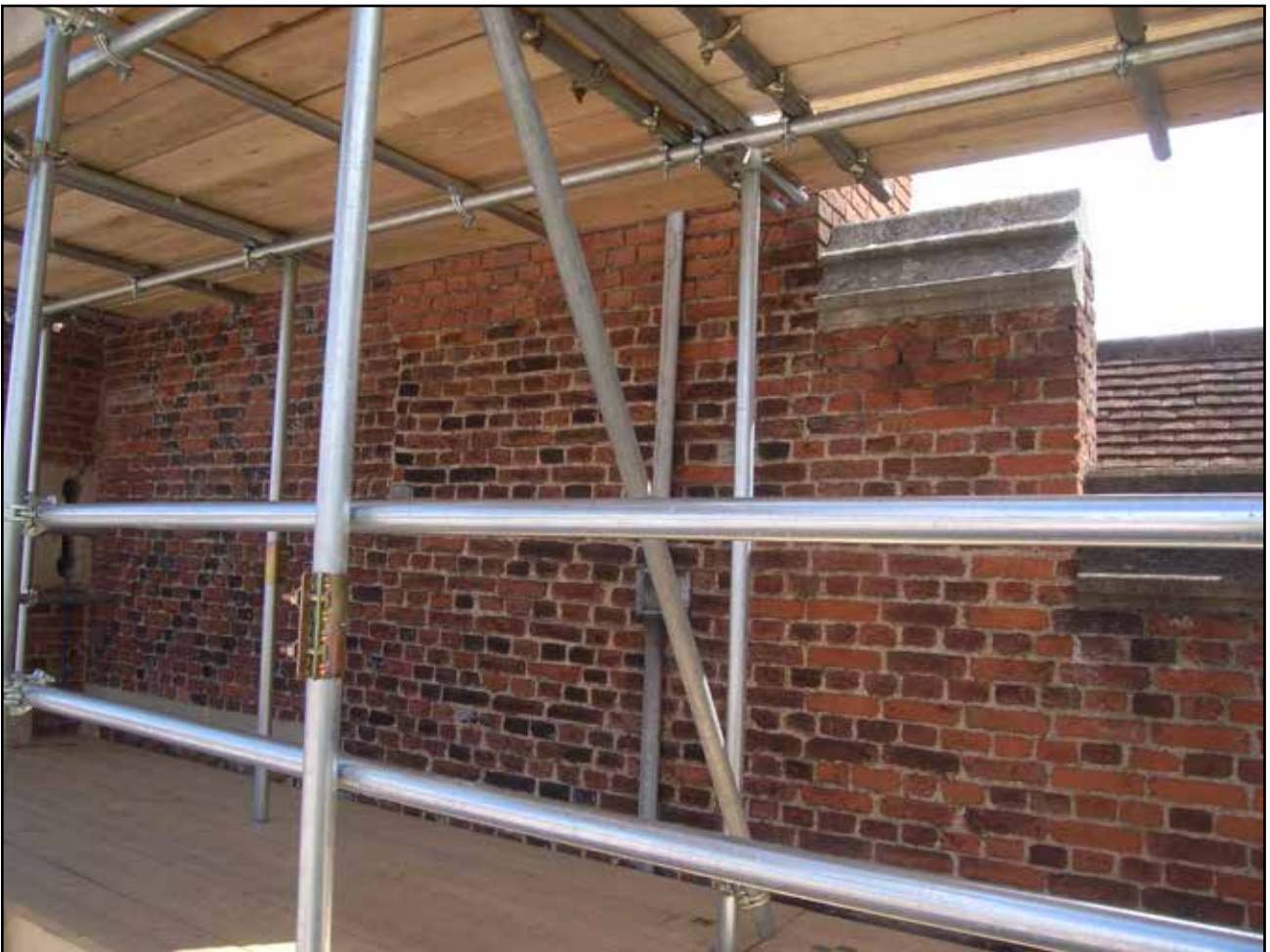
Plate 4: Base Court - West facing Elevation Part 1, upper parapet, looking north east
