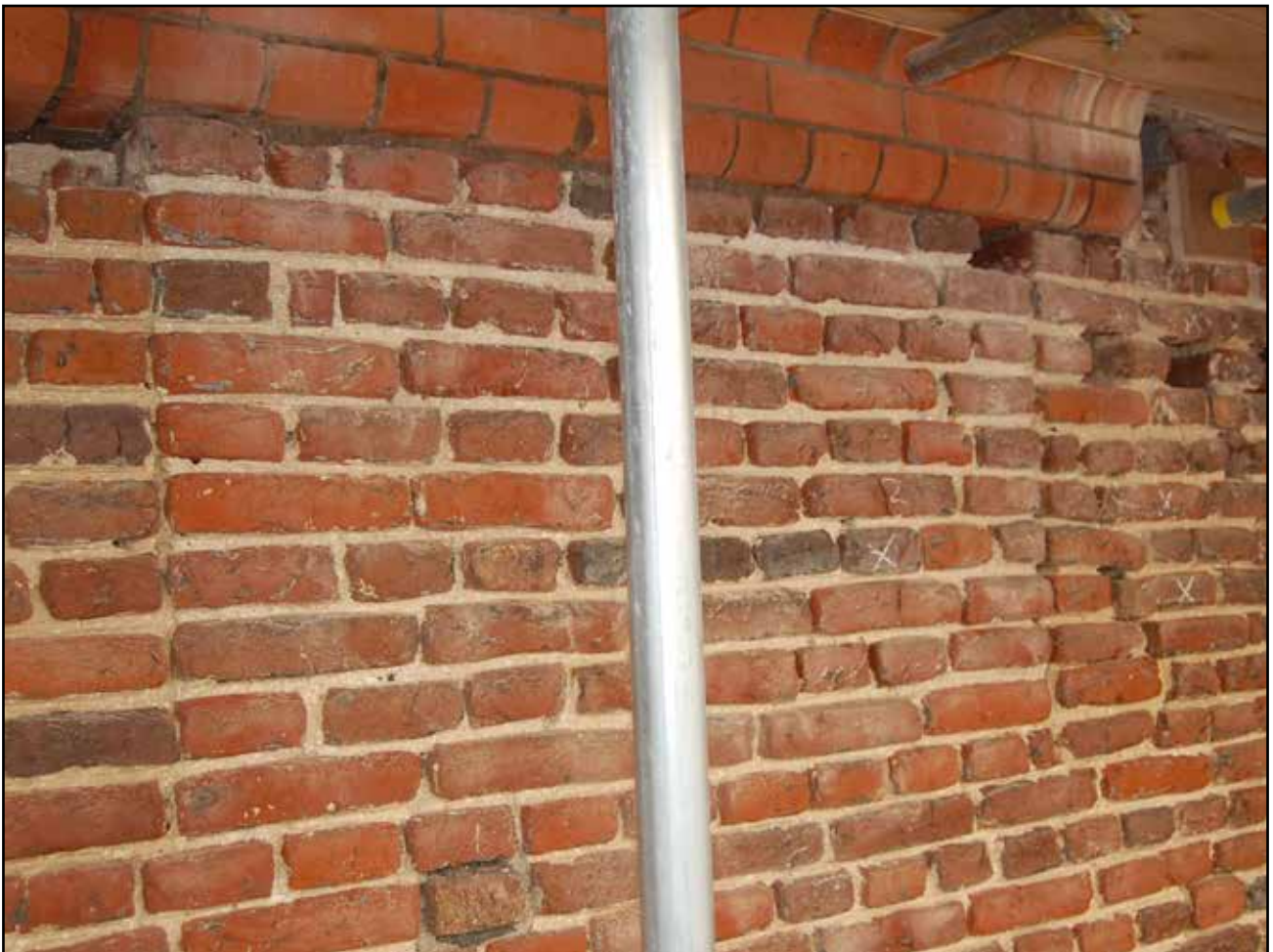
Plate 22: Evidence of crenellations in the Upper East Facing Elevation Part 2, Clock Court
