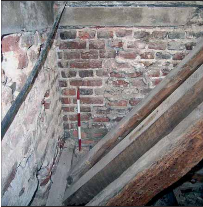
Plate 17: Buttery Return Wall, looking north
