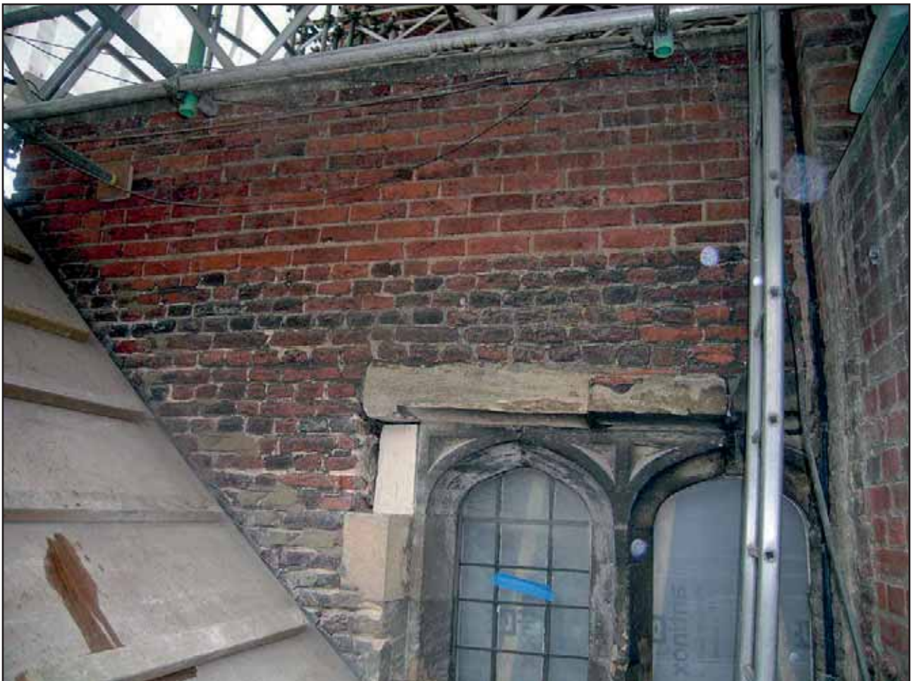
Plate 4: Base Court – West Facing Elevation Part 1, looking north east
