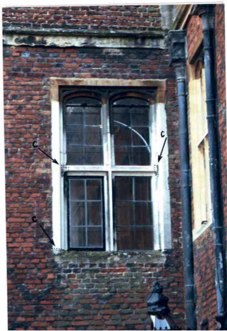
Plate 8. Base Court 1st floor windows at south end of range. Remnants of Caen stone (C) in jambs.
