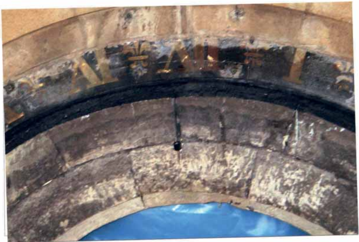
Plate 7. Detail of Plate 6. The yellow outer stone of the surround is a 20th century Clipsham stone restoration.
