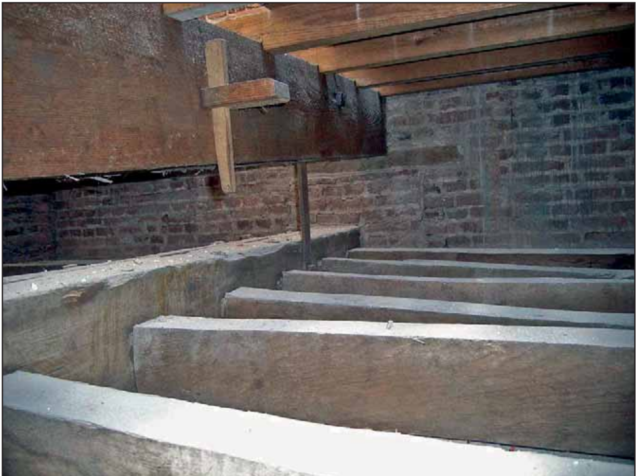
Plate 32: The Upper and Lower structures of the Flat Roof, looking east
