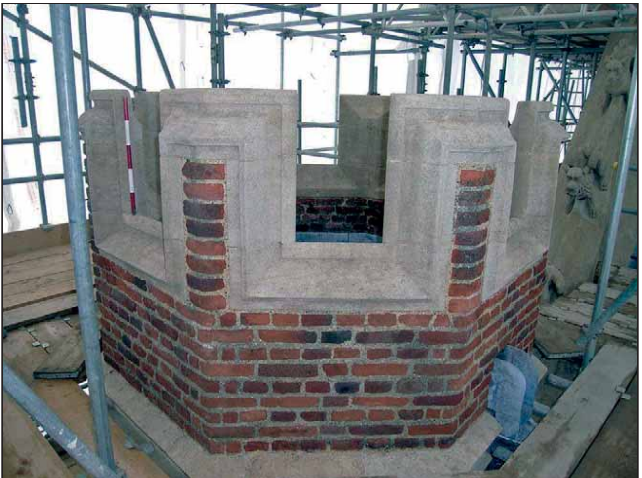
Plate 12: Parapet of Turret 16, looking north west
