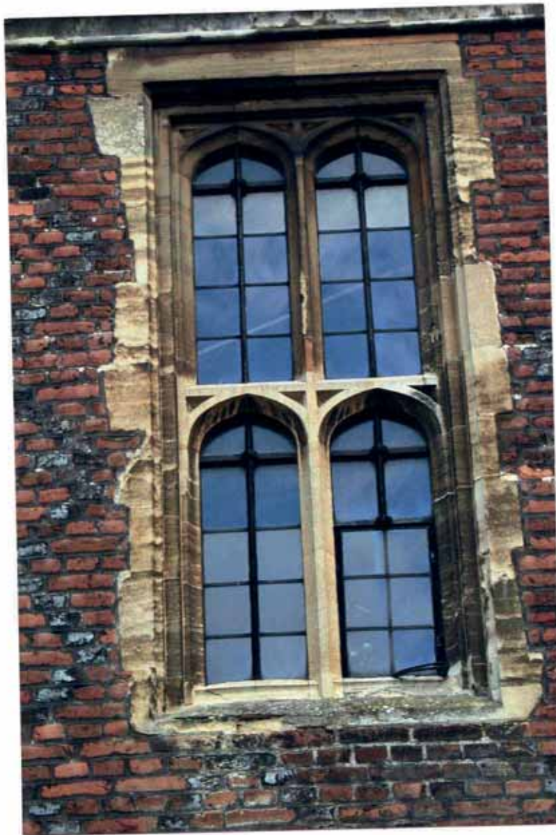
Plate 12. Base Court, south range. 1st floor window of Wheatley Limestone.
