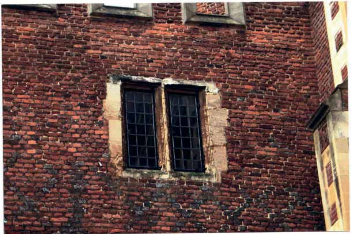
Plate 4. Clock Court, north-west corner 2nd floor window with Beer stone lintel & Bath stone jambs and sill.
