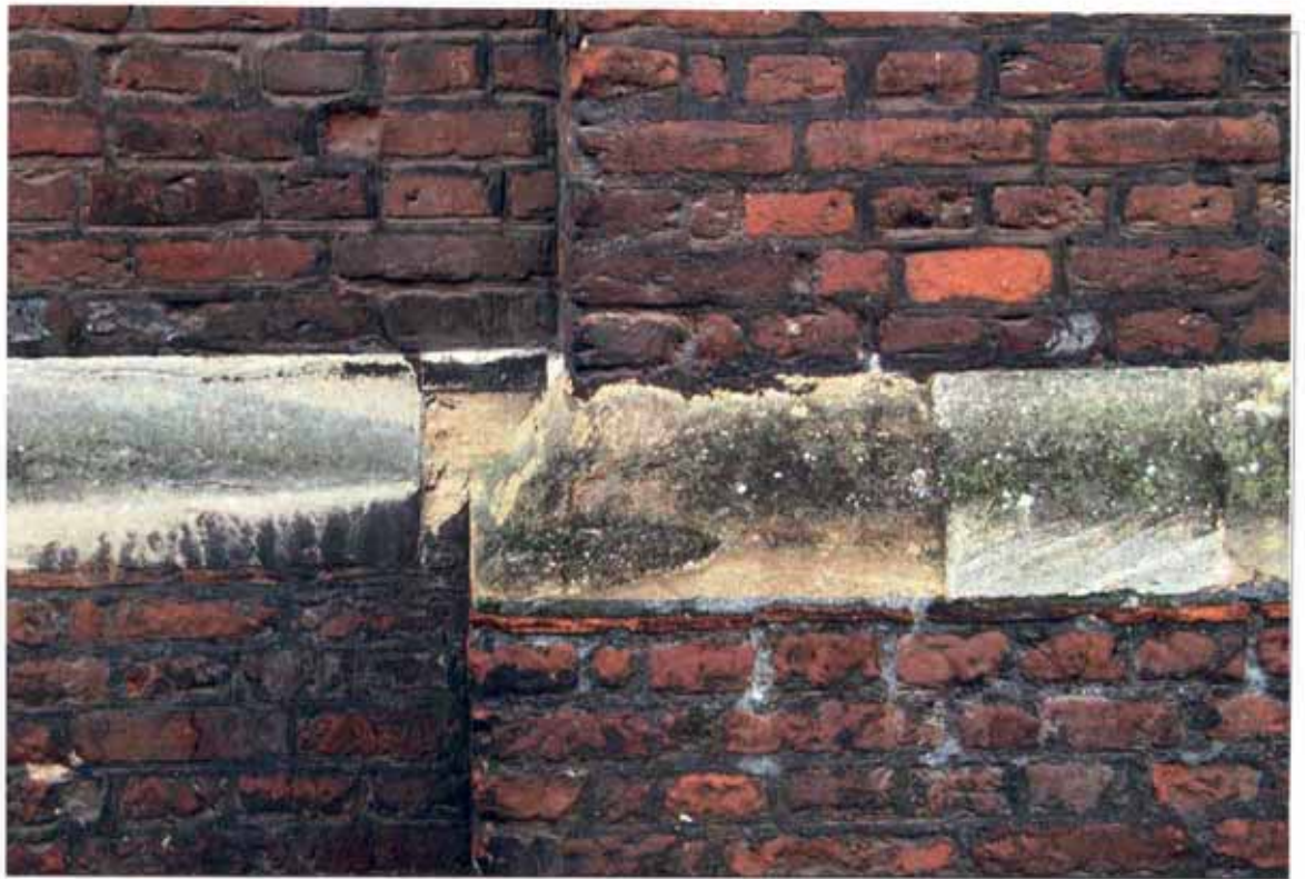
Plate 10. Clock court, 4-flue chimney stack plinth. Yellow Guiting stone? replacement in Bath stone offset course.
