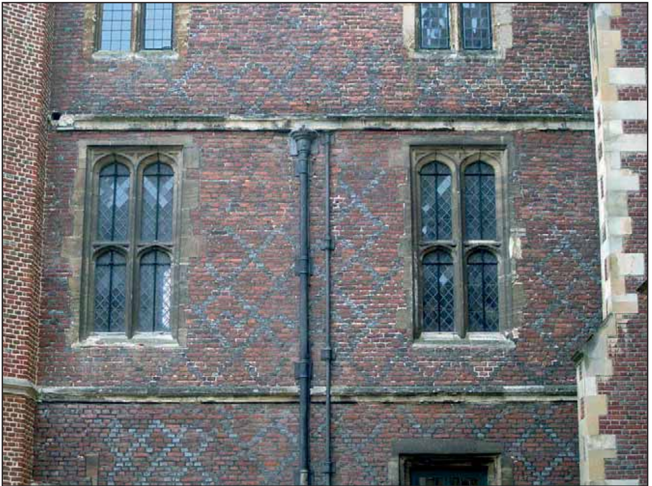
Plate 11: Detail of brickwork on East Facing Elevation of Clock Court
