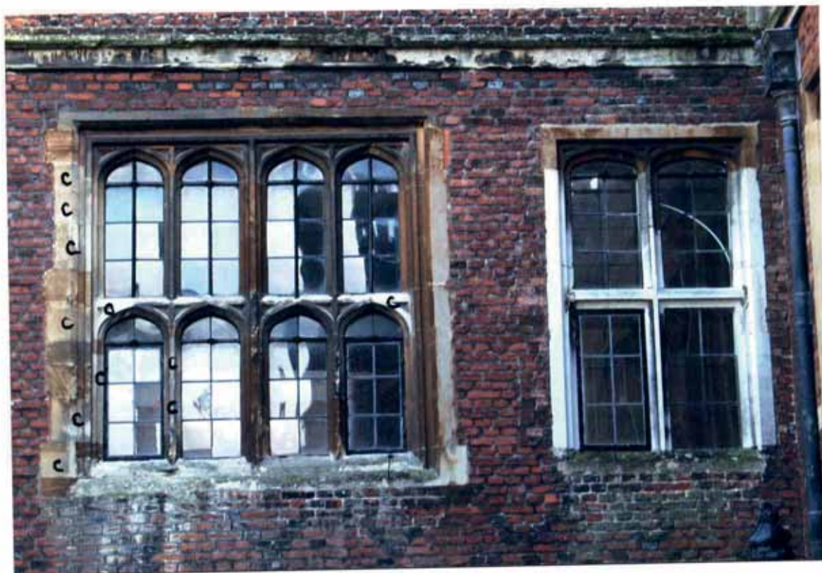
Plate 8. Base Court 1st floor windows at south end of range. Remnants of Caen stone (C) in jambs.
