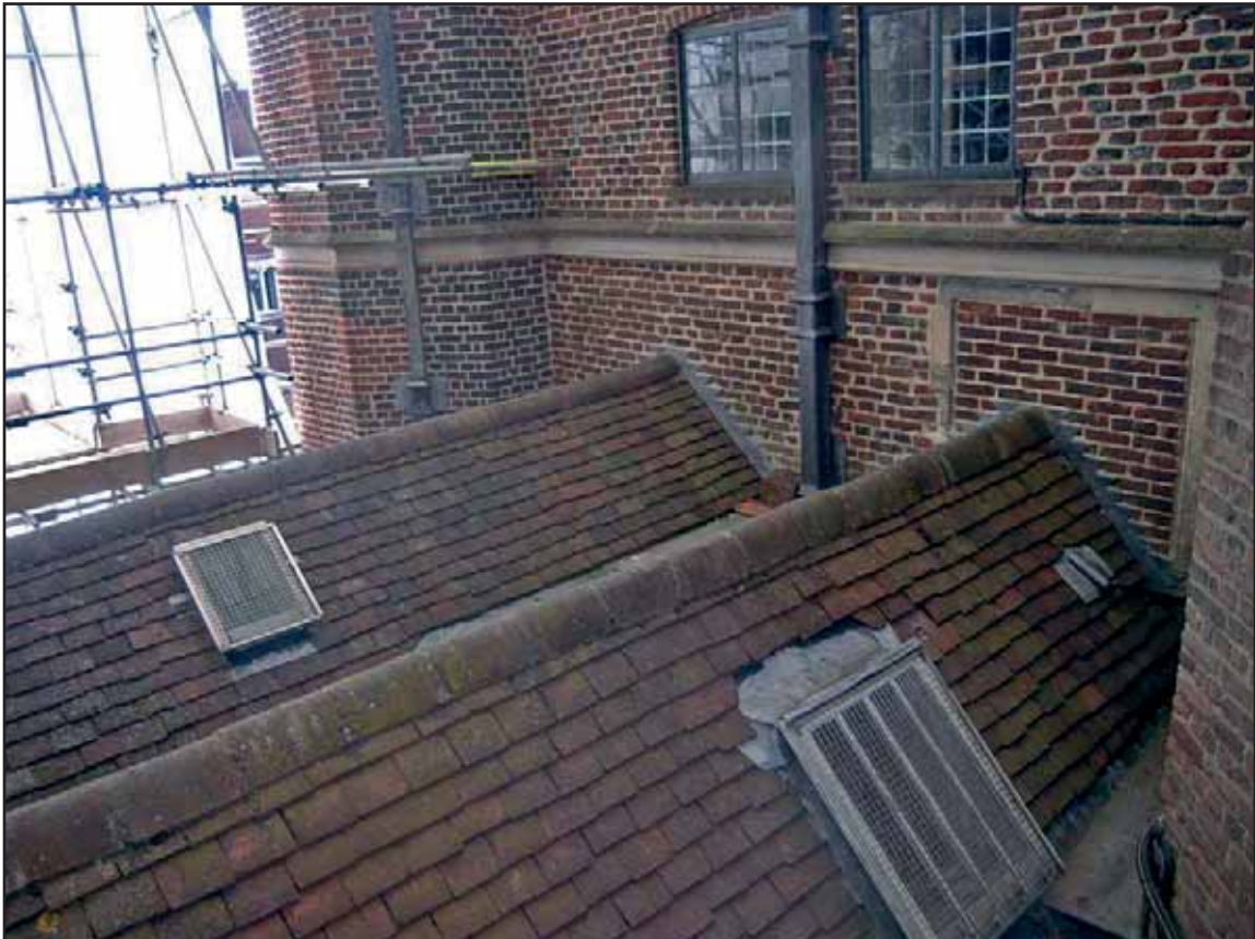
Plate 22: The Main Roof, looking south east
