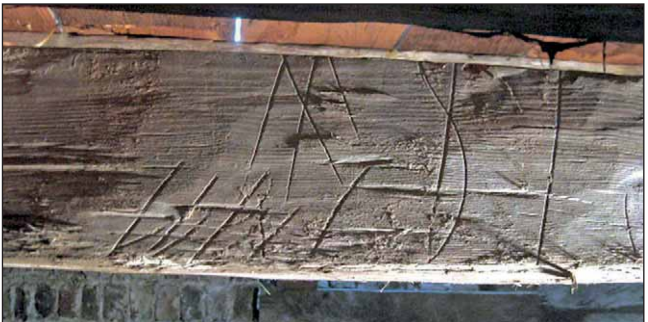
Plate 34: Baltic Marks on the east and under side of joist in Bay 2 of the Upper Structure of the Flat Roof
