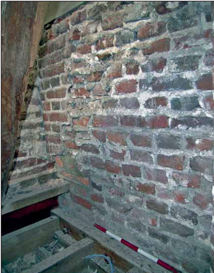
Plate 18: Buttery Return Wall, looking north west
