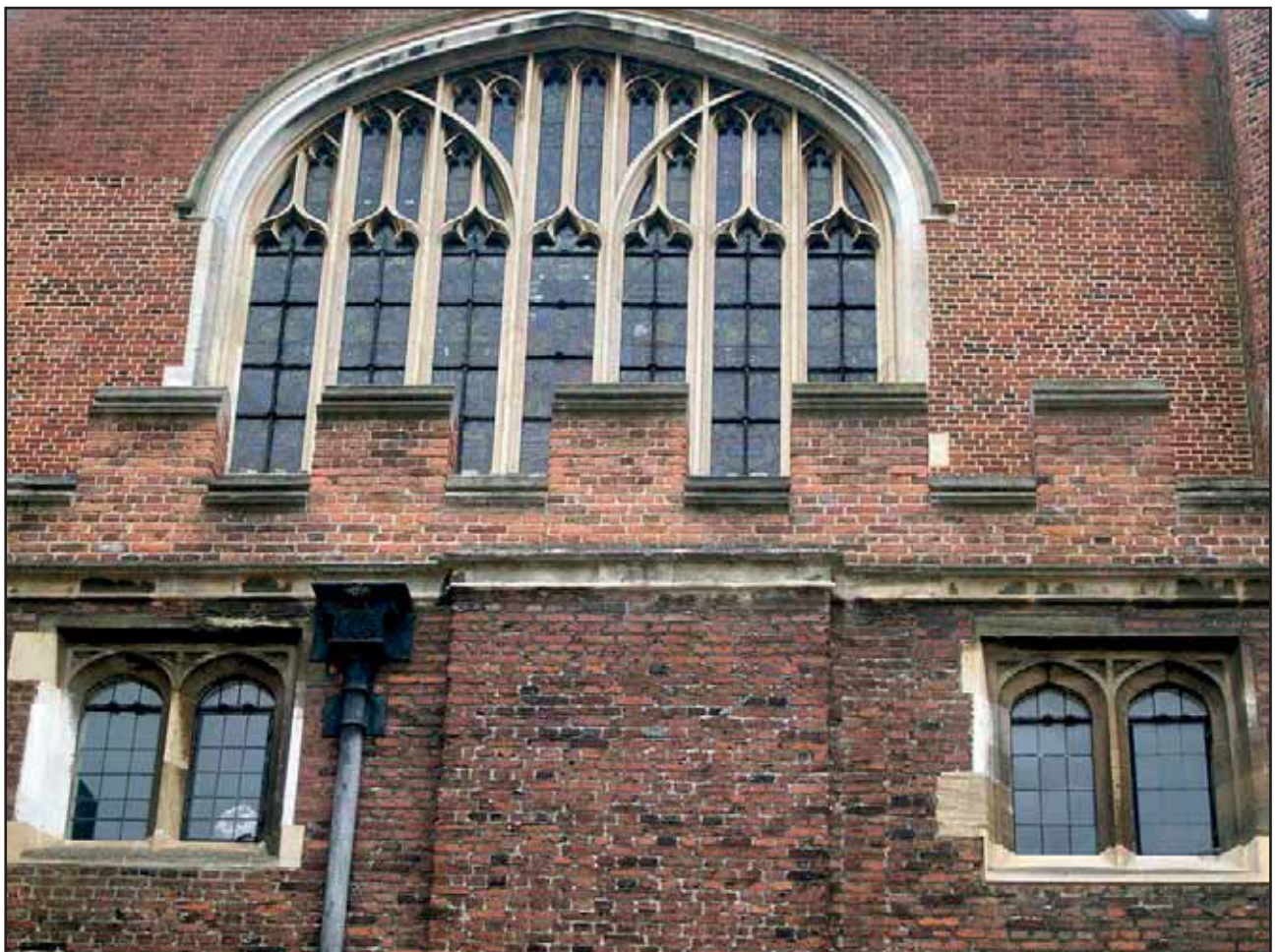
Plate 6: View of parapet of the Buttery, looking east
