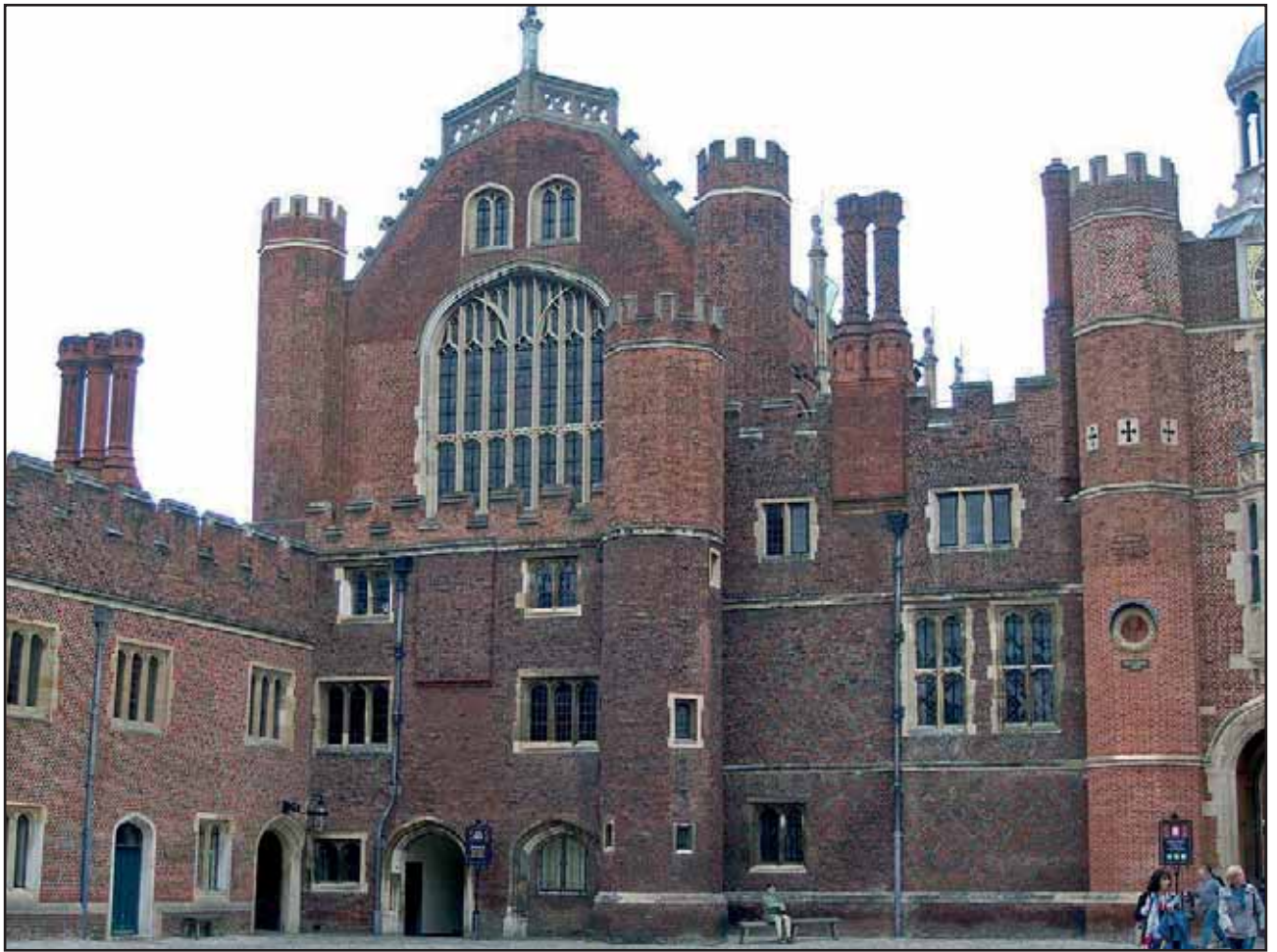
Plate 1: Base Court area of conservation, looking north east
