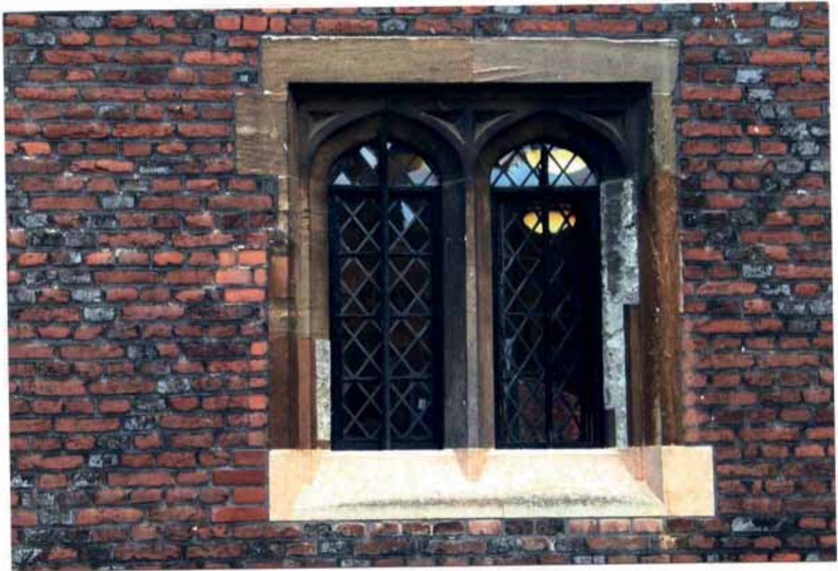
Plate 3. Base Court, ground floor window showing four phases of construction and repair. In order - Reigate stone (grey), Wheatley Limestone (grey-brown), Bath stone (brown), 20th century Bath Stoke Ground Base Bed (sill).
