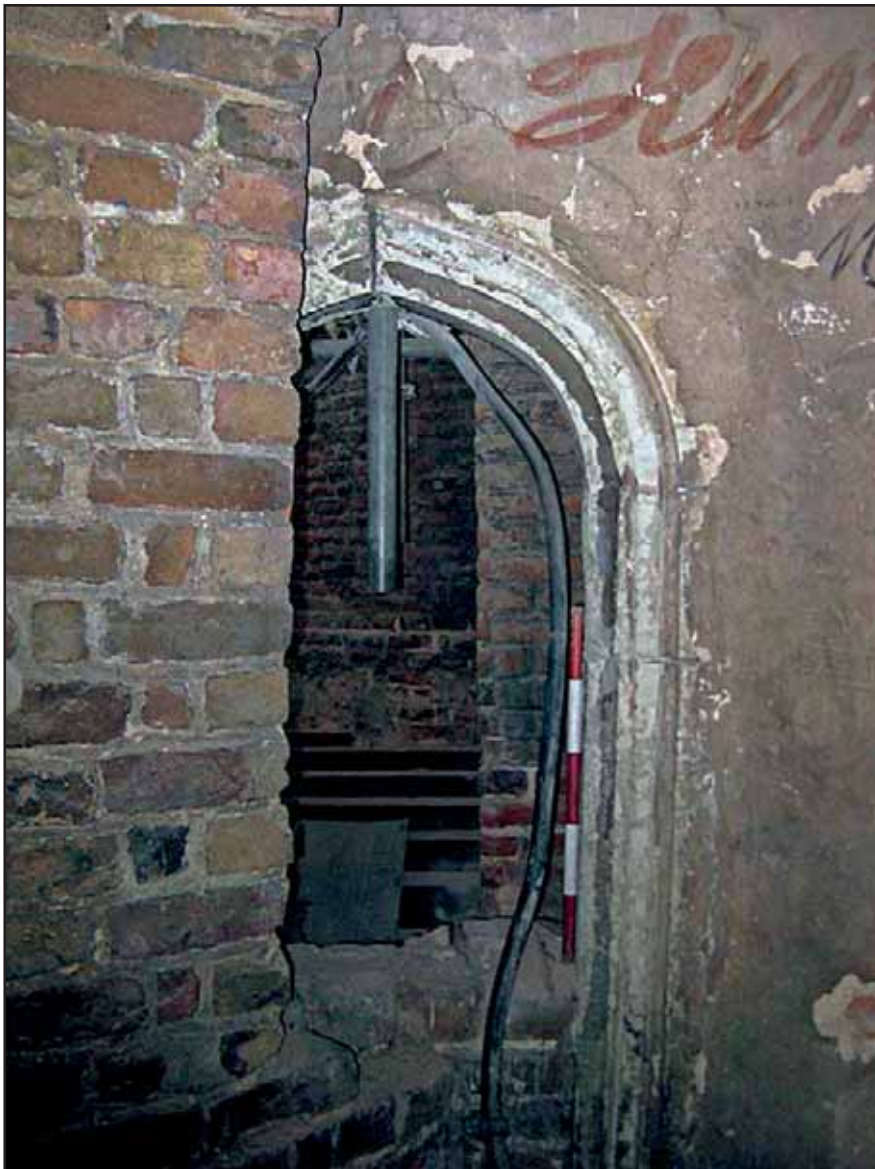
Plate 36: Doorway of Turret 12, viewed from the interior, looking east
