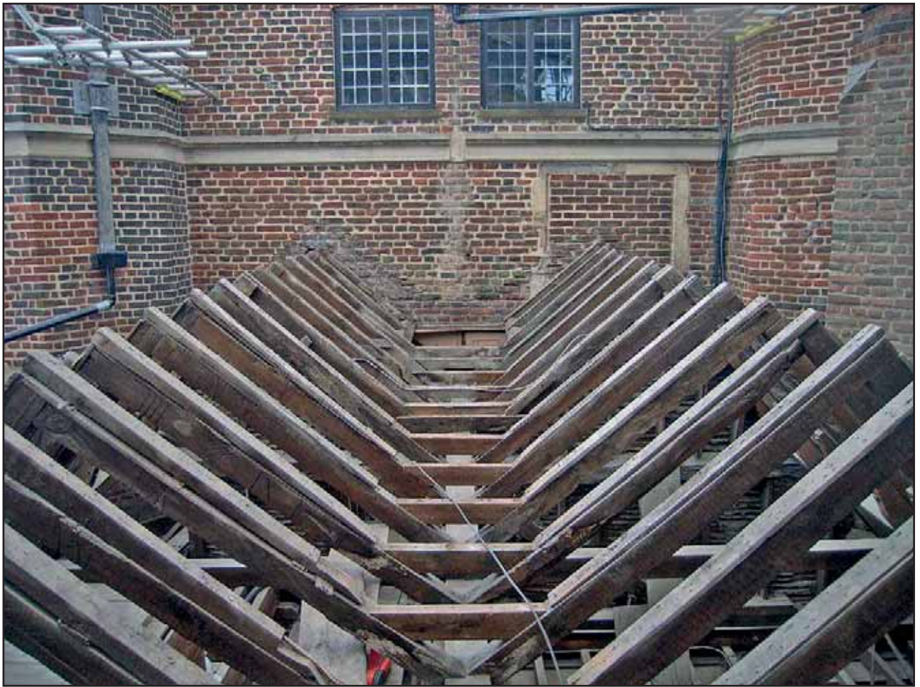
Plate 23: The exposed timbers of the Main Roof, looking south
