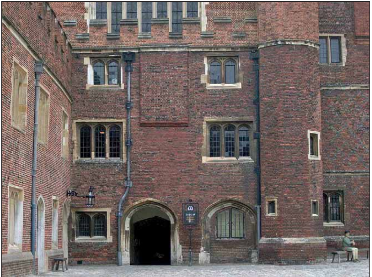
Plate 5: West Facing Elevation of the Buttery, looking east
