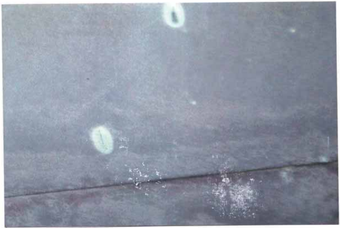
Plate 15. Reduction spots in slate. Detail of Plate 14.
