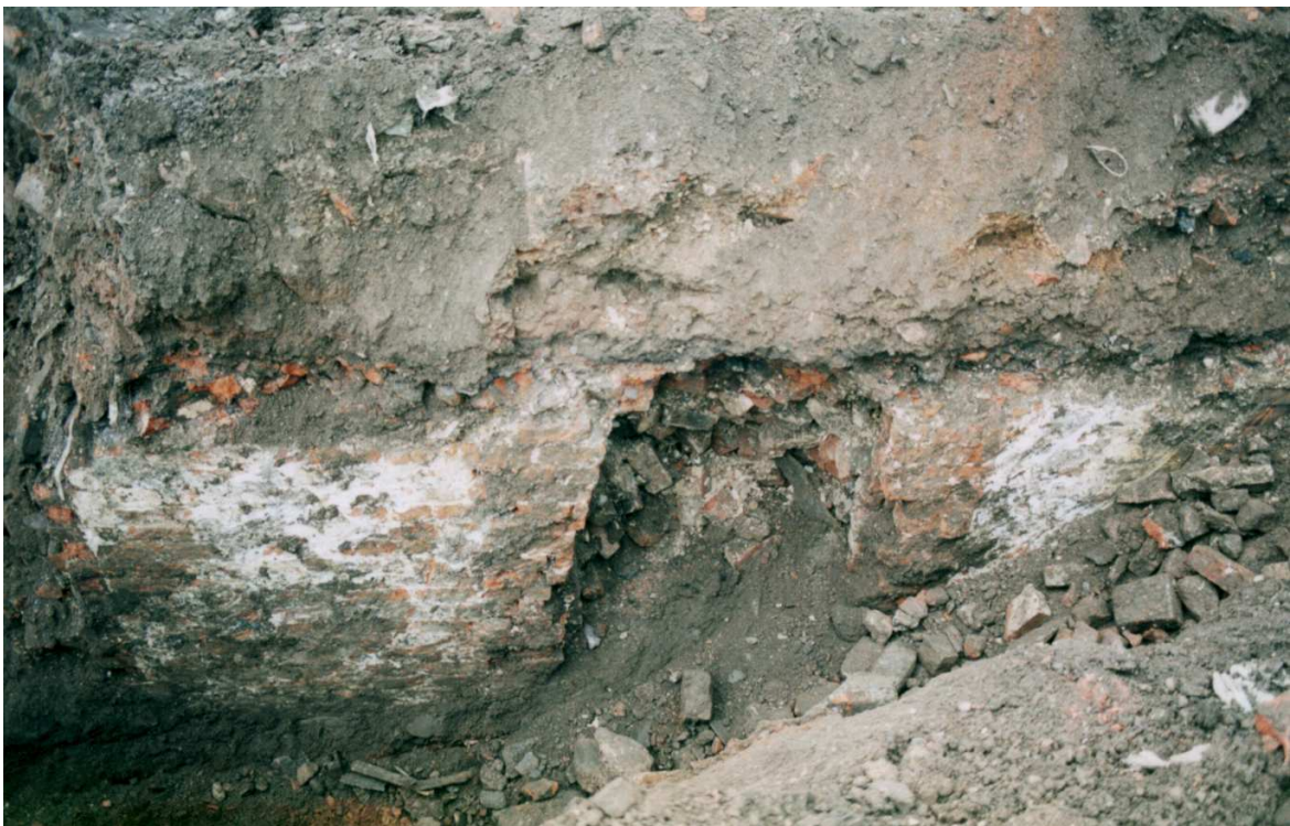
Plate 4 Cellar wall (Feature iv) between Units 17 and 18 looking north-east
