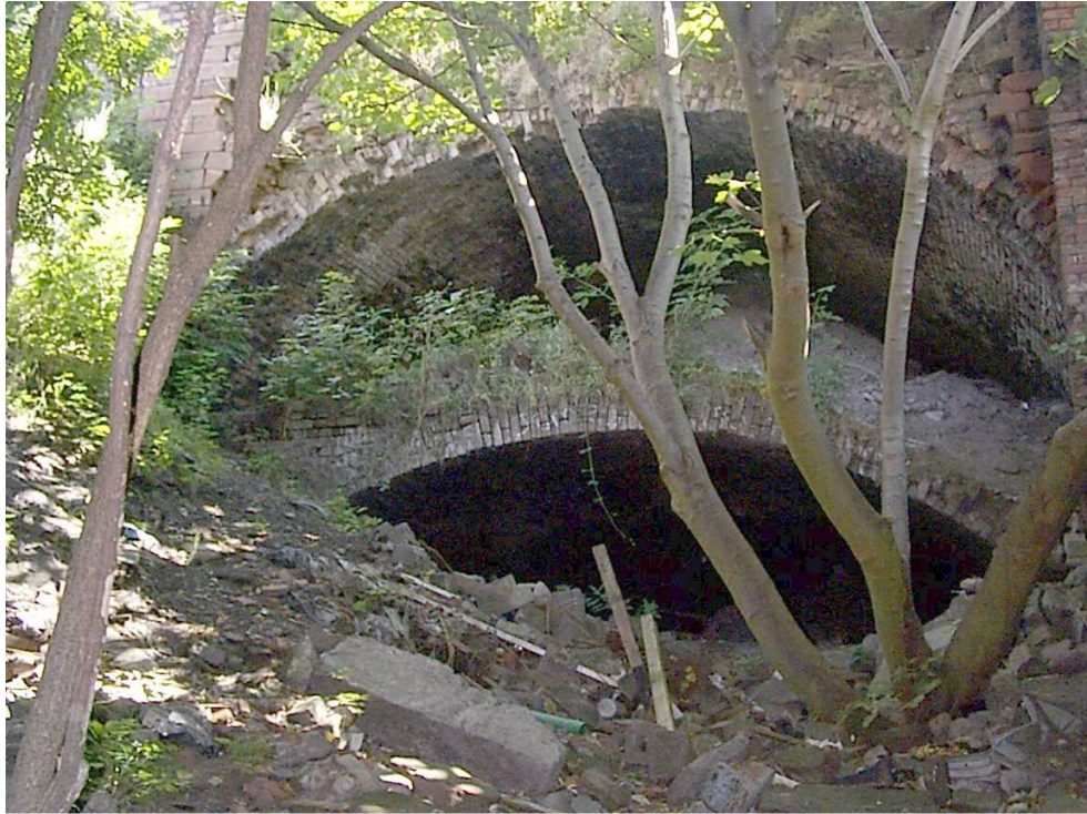
Plate 13 Entrance to double tunnel 9 – looking east
