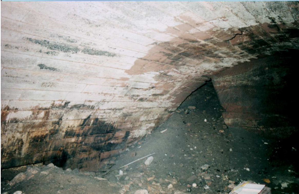
Plate 9 Tunnel 10, entrance to the northern passage prior to piling
