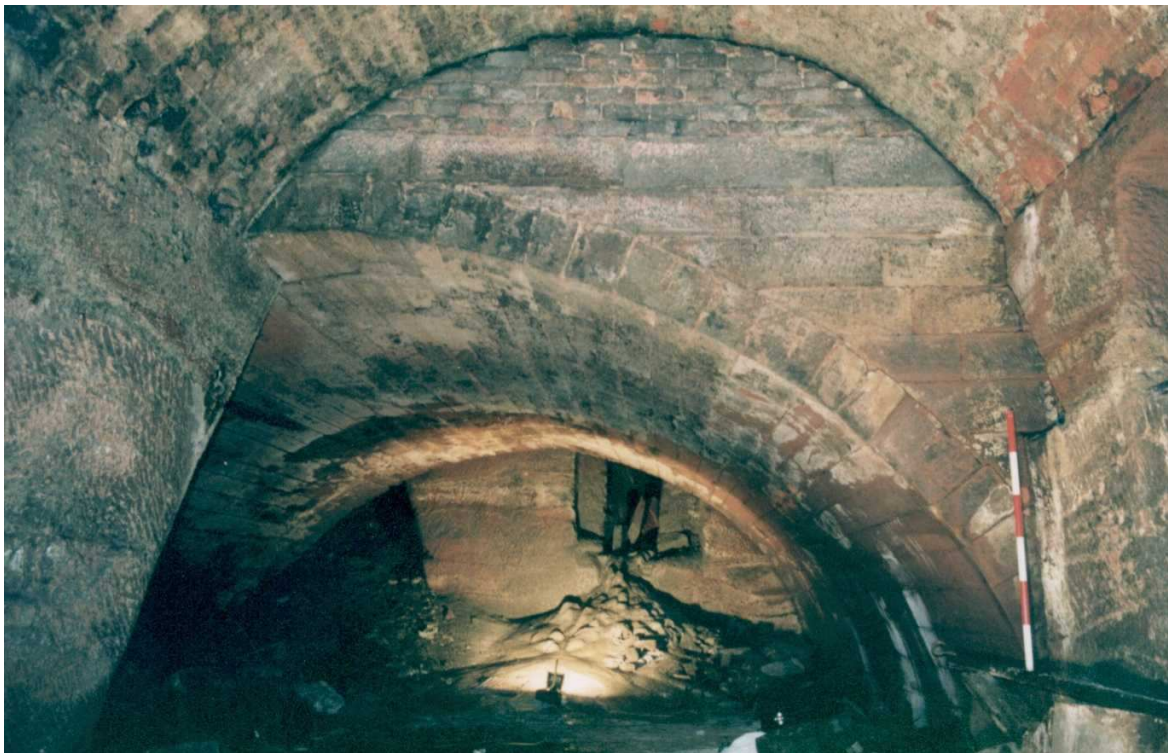
Plate 12 General view of the Tunnel 10 and passages, post piling – looking east
