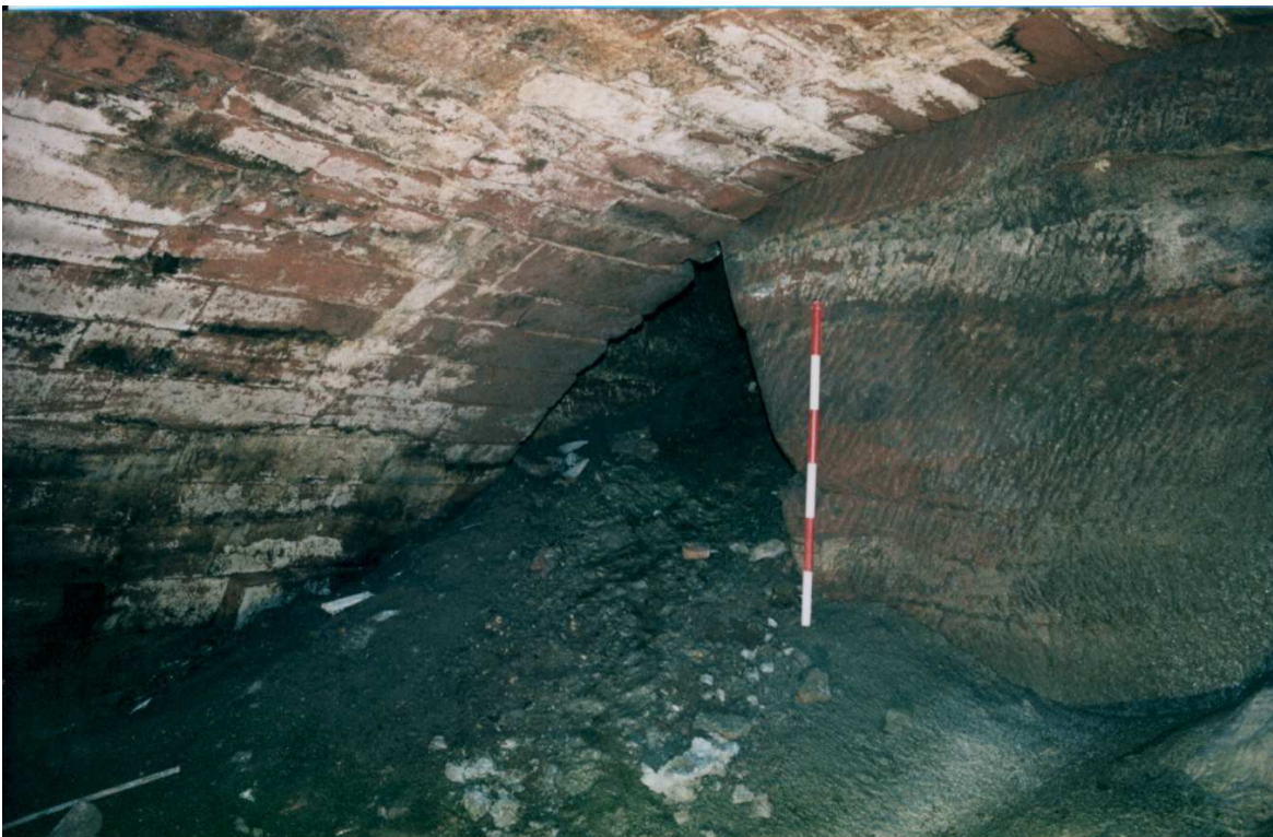
Plate 10 Tunnel 10, entrance to the northern passage after piling – looking east
