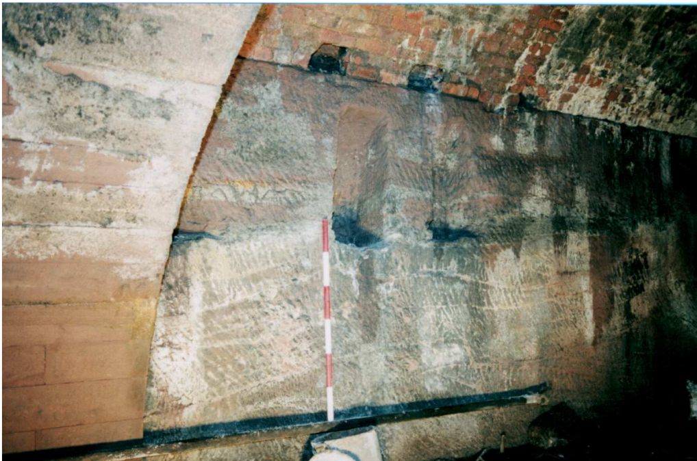
Plate 14 Arch former sockets in the south side of Tunnel 10
