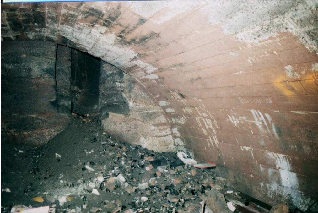
Plate 7 Interior of Tunnel 10, southern passage entrance, taken prior to the piling
