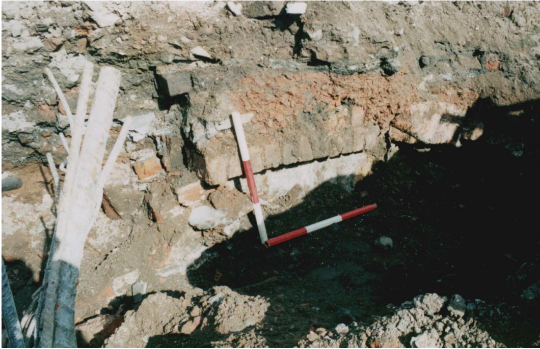
Plate 5 Upper part of vaulted cellar (Feature vi) after removal of the vault
