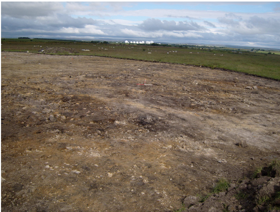
Plate 3: Topsoil stripped near Turbine 8, Area 3
