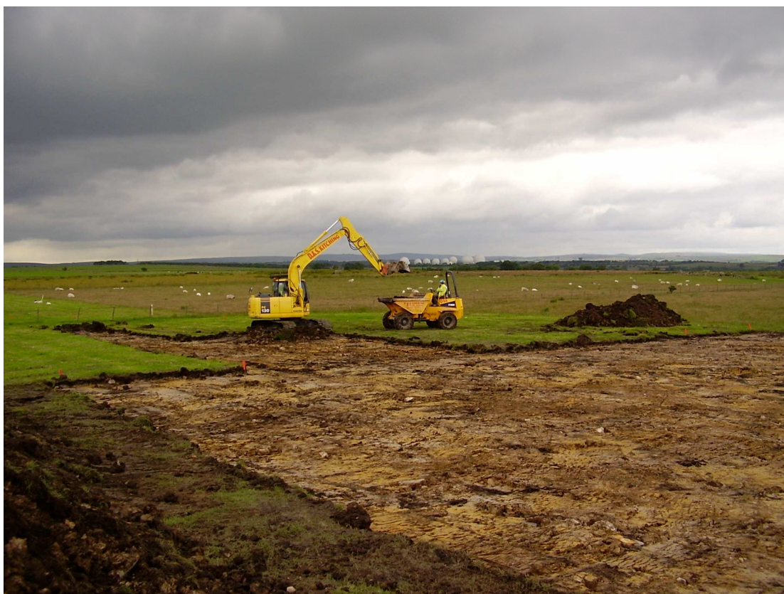
Plate 1: Working shot of topsoil strip
