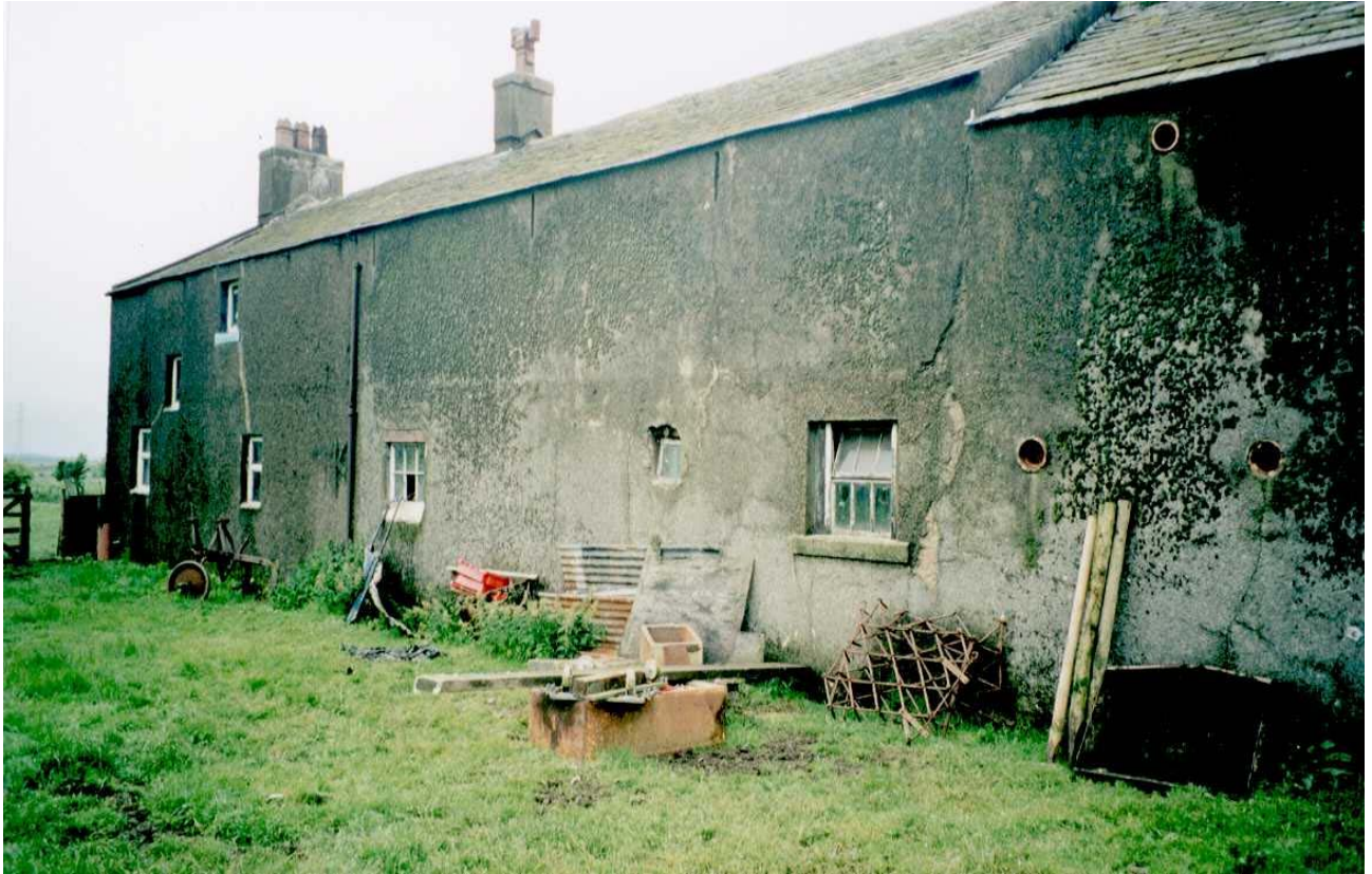
Plate 3 Sandbeds Farmhouse and Barn – South Elevation
