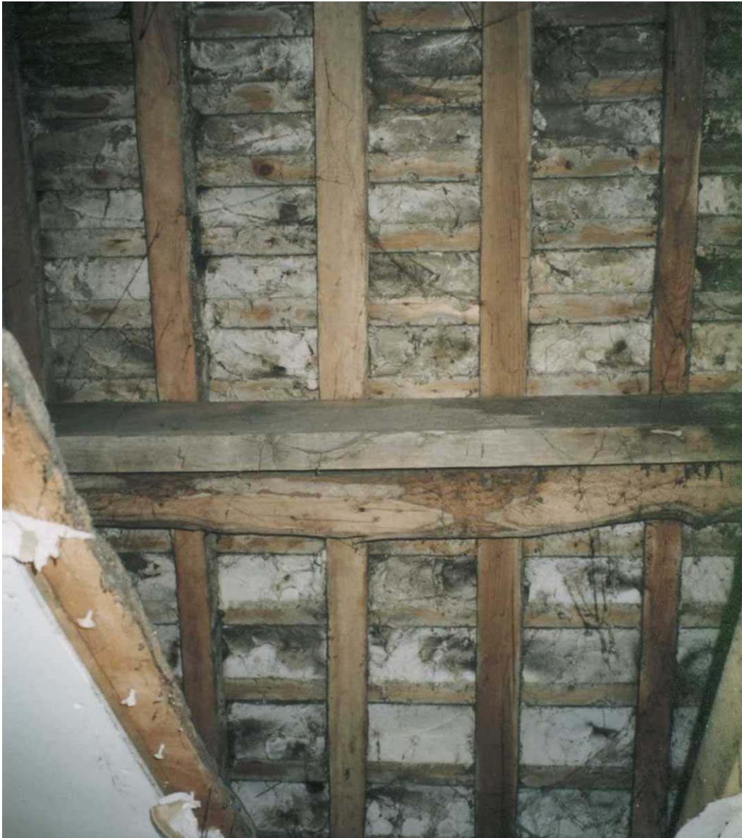
Plate 5 Sandbeds Farmhouse Roof, Showing Rough Sawn Purlin
