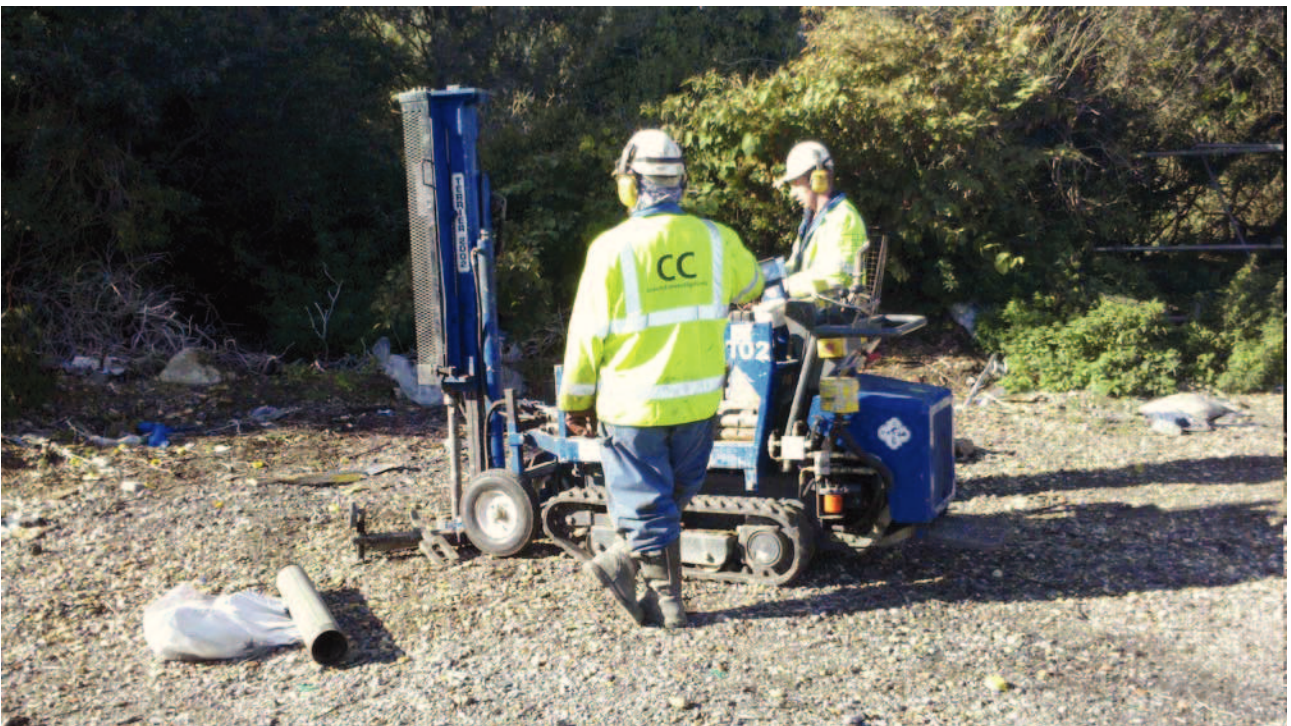
Plate 2: Borehole sampling
