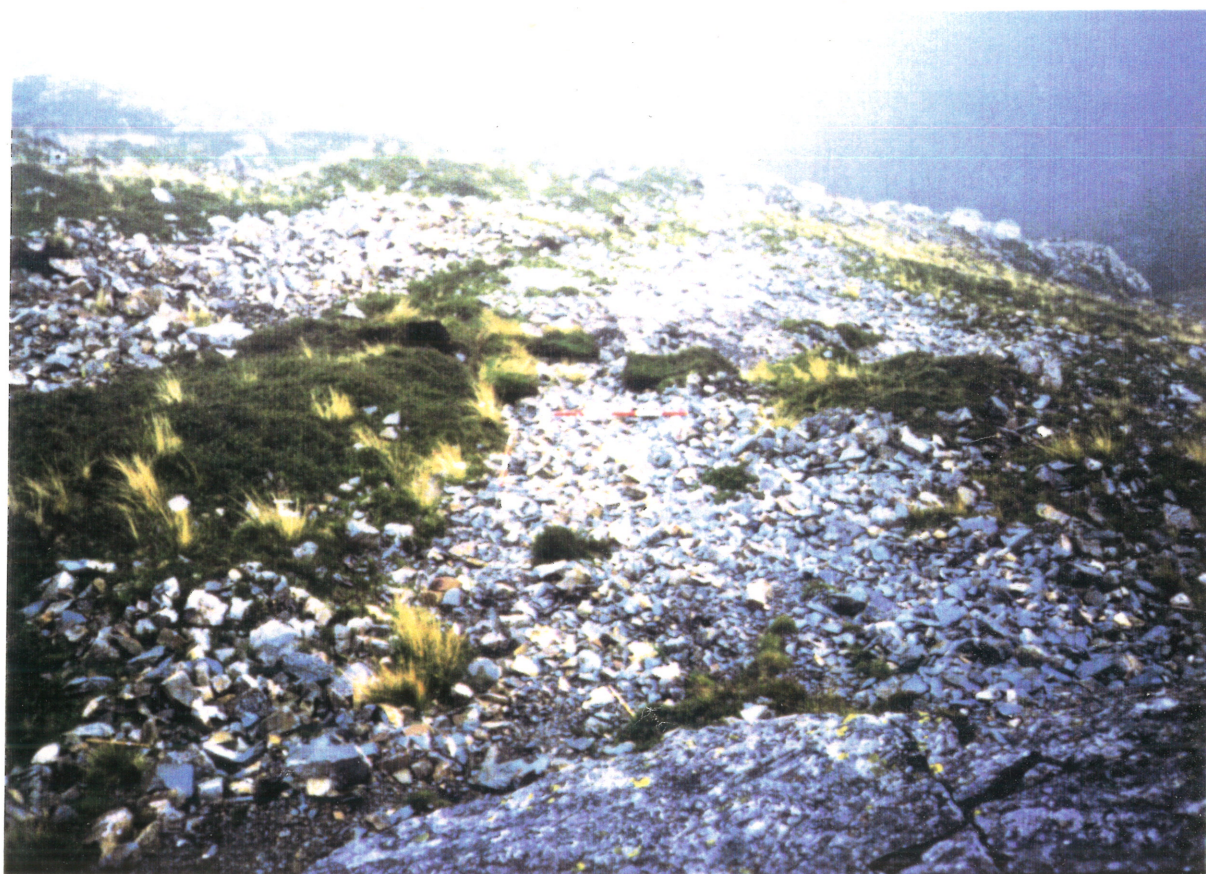
Plate 4 Harrison Stickle site 162 before repair
