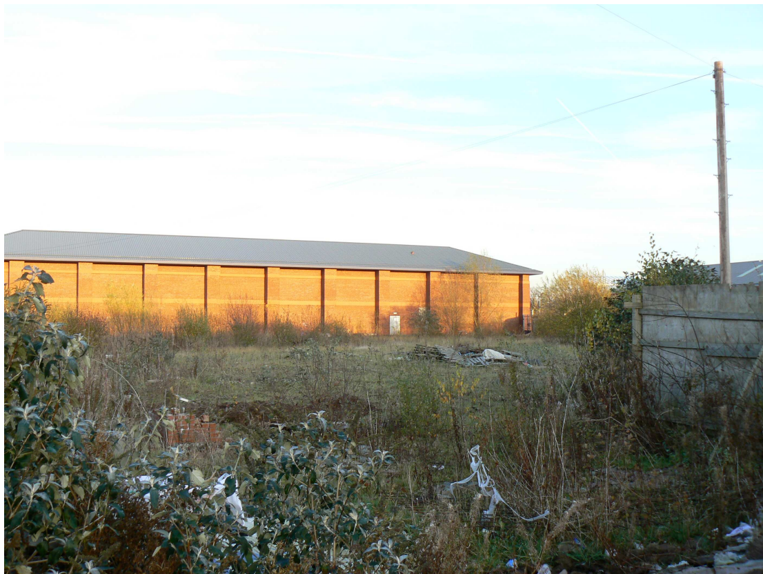
Plate 1: View looking north-east across the proposed Scheme Area
