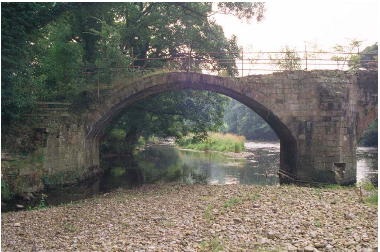
Plate 2 East arch of bridge looking south-west
