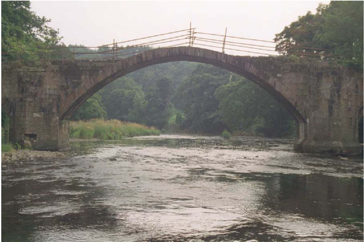
Plate 3 Central arch of bridge looking south-west
