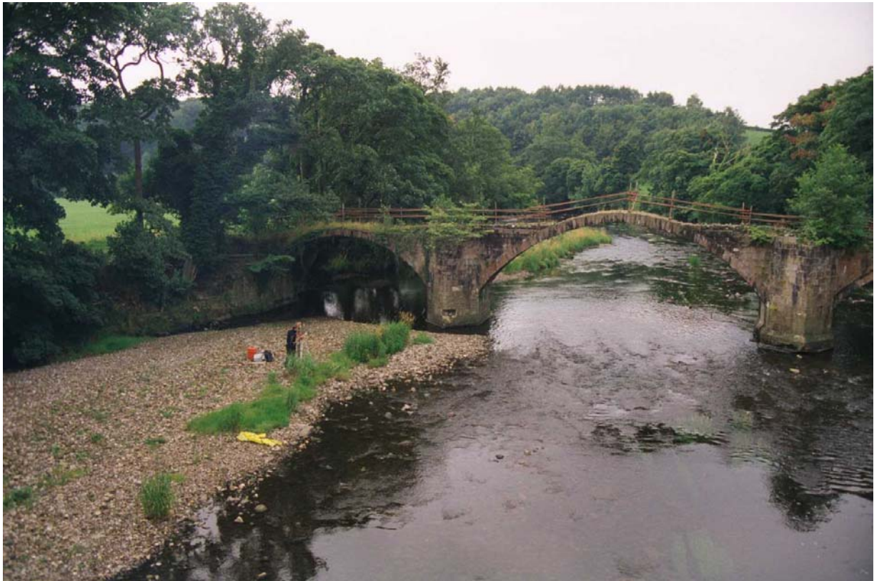
Plate 1 General view of Cromwell's Bridge looking south-west
