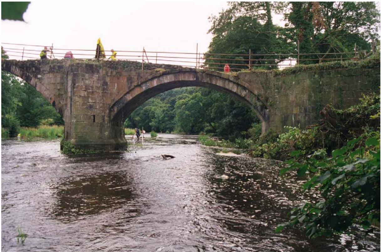
Plate 4 West arch of bridge looking south-west
