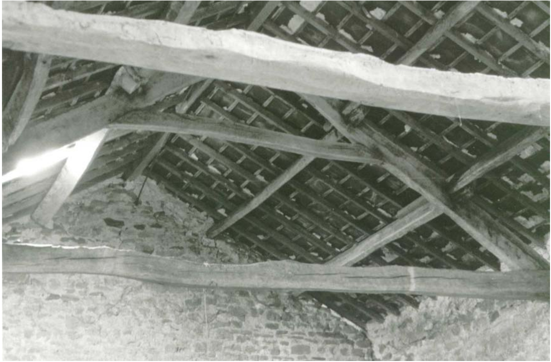
Plate 5: Southern Truss in the Barn from the south-west
