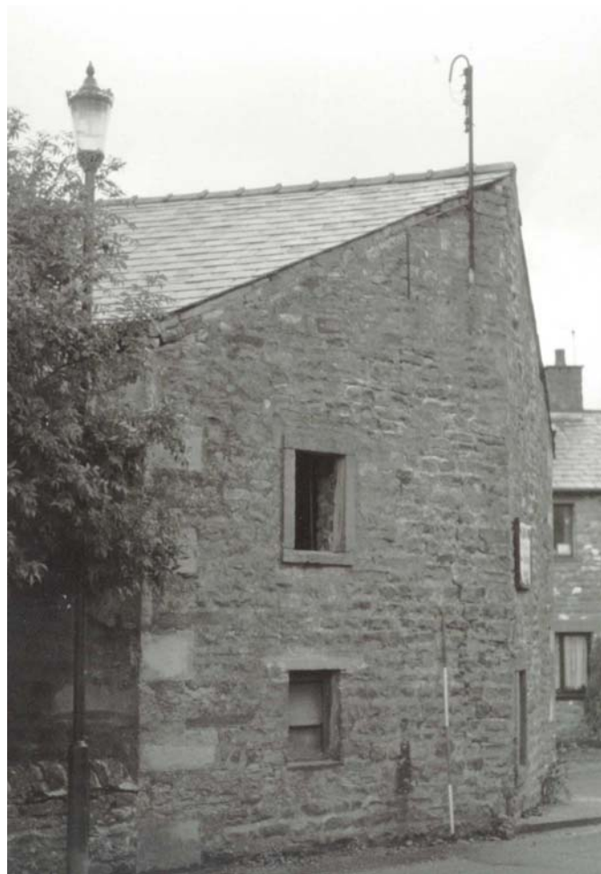
Plate 2: South External Elevation from the south-west
