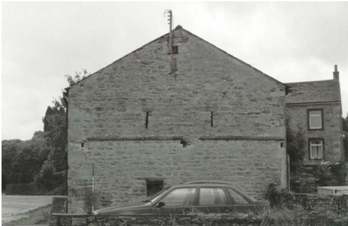
Plate 3: North External Elevation from the north
