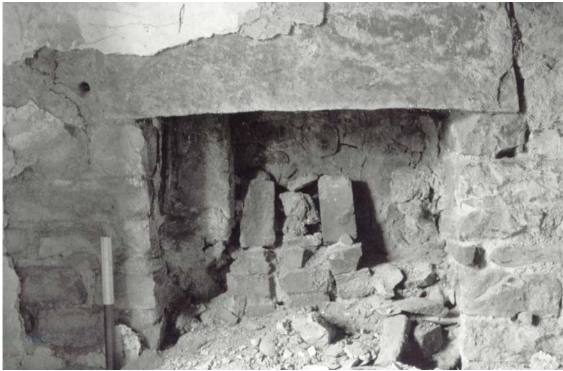
Plate 7: Fireplace in Room 4 from the north
