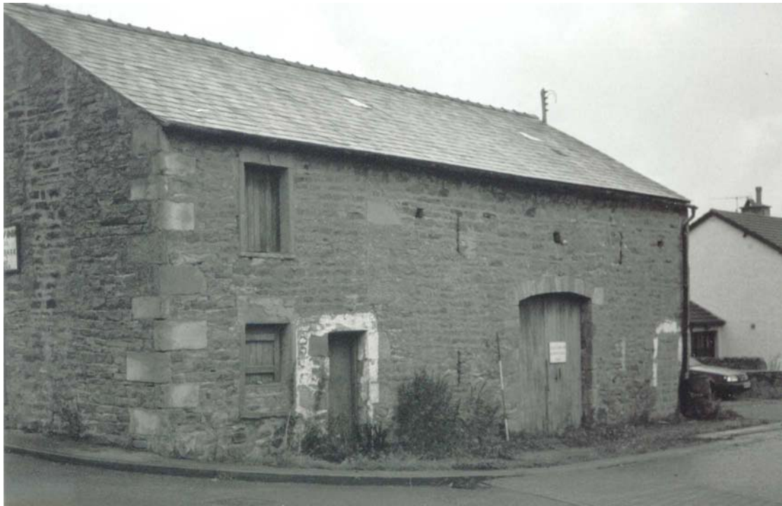
Plate 1: South and East External Elevations from the south-east
