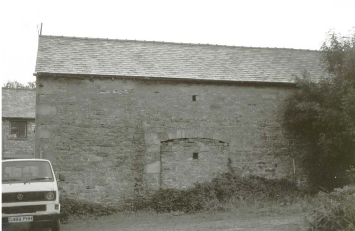
Plate 4: West External Elevation from the west
