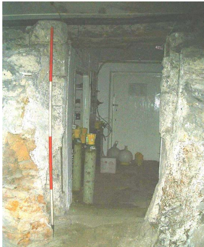
Plate 2 Relict Doorway looking south-east
