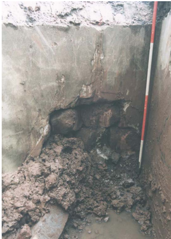
Plate 6 Trench 16 - Sandstone masonry exposed in eastern concrete wall
