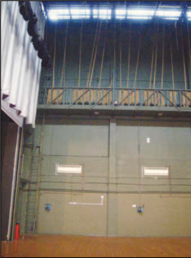
Plate 11: Adeline Genee Theatre, internal north-east view showing balcony and fly gallery within stage area
