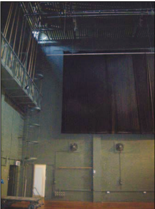
Plate 13: Adeline Genee Theatre, south-east view of stage area showing projection curtain, balcony and exits
