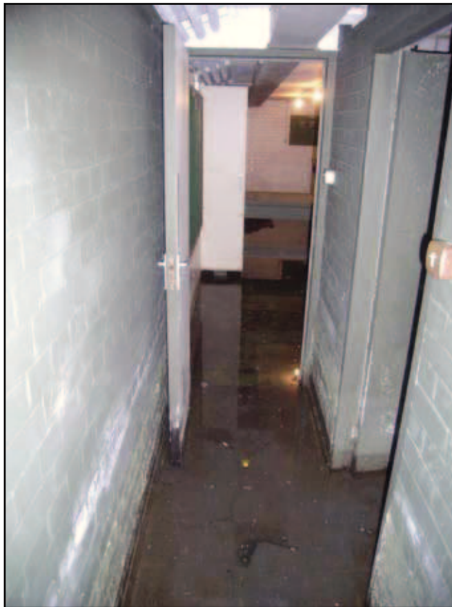
Plate 29: Towards Band Room from south-west
