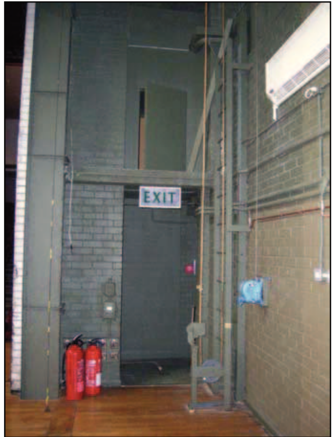
Plate 12: Adeline Genee Theatre, north-west view of north corner of stage showing curtain pulley and exit
