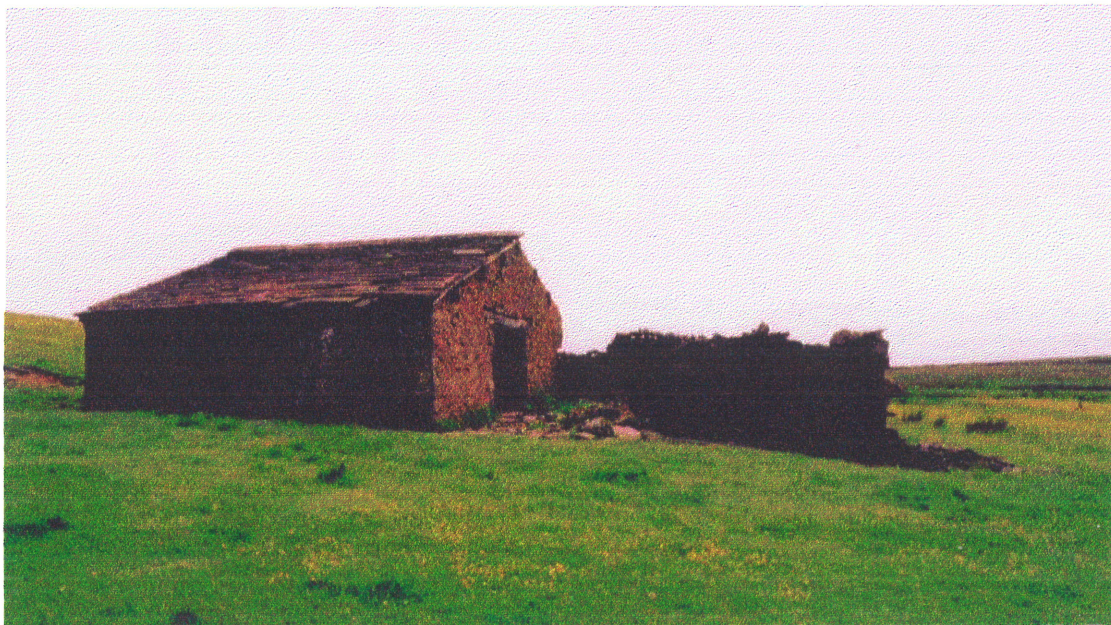
Fig 5 Photograph of field barn – Site 28
