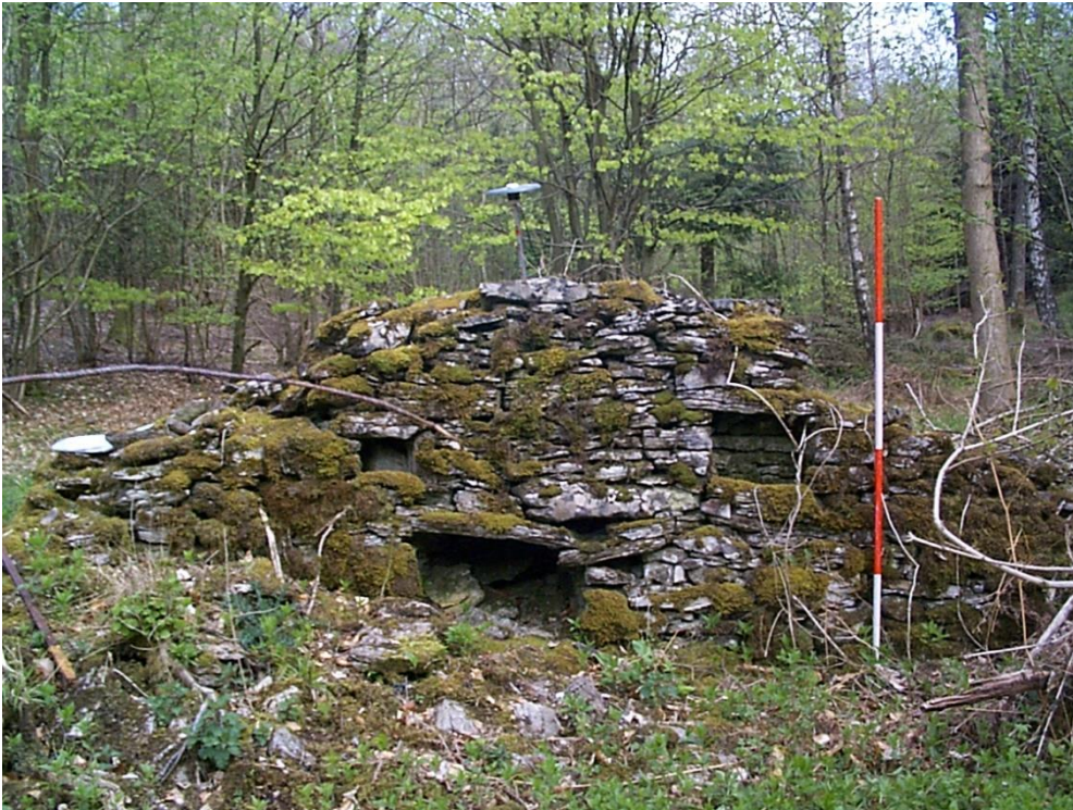
Plate 9 Building B17 in Barrowfield Wood
