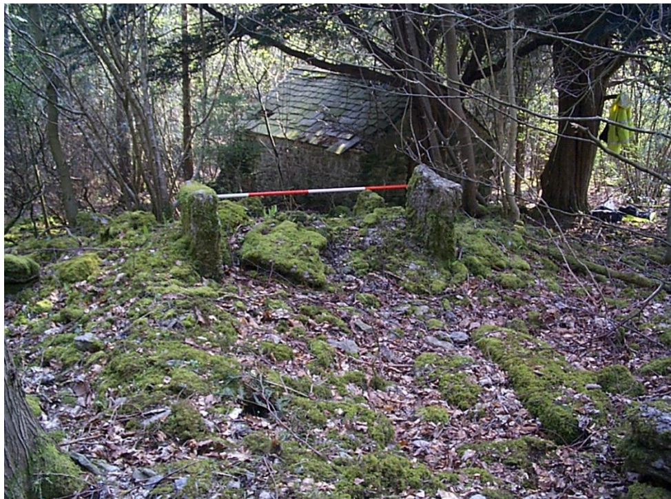
Plate 4 Building W20 (structure adjacent to W21)
