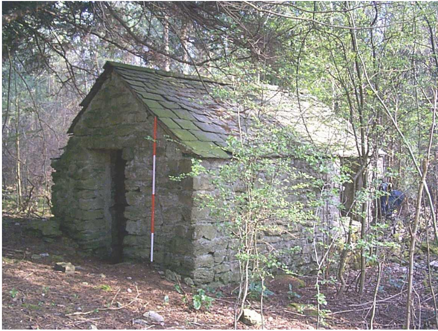
Plate 5 Building W21 at Fothersty Green
