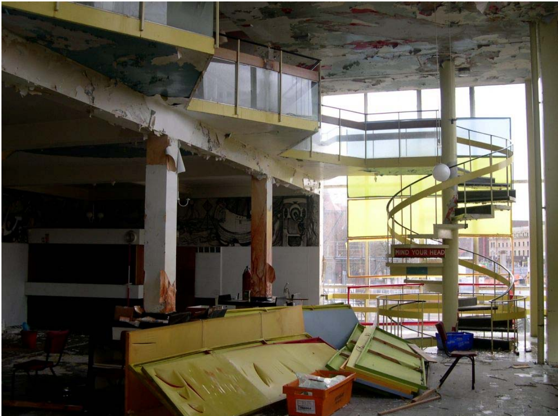
Plate 8: East aspect of the main dining salon (Room 110), and spiral staircase, First Floor
