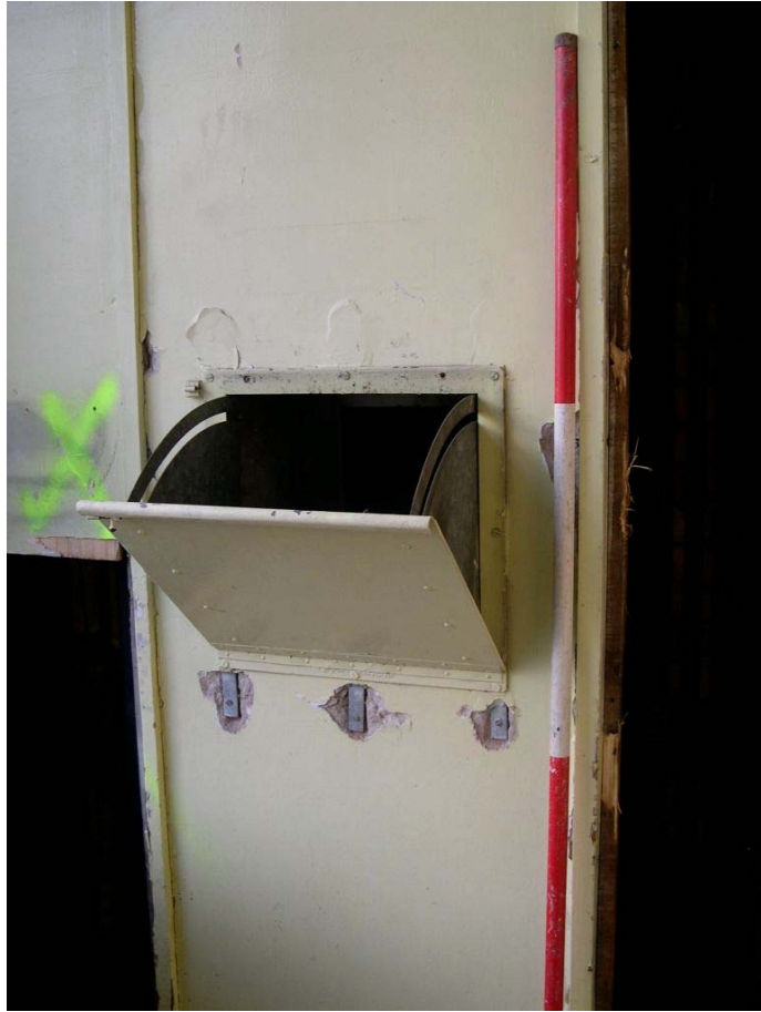
Plate 22: Example of a waste chute
