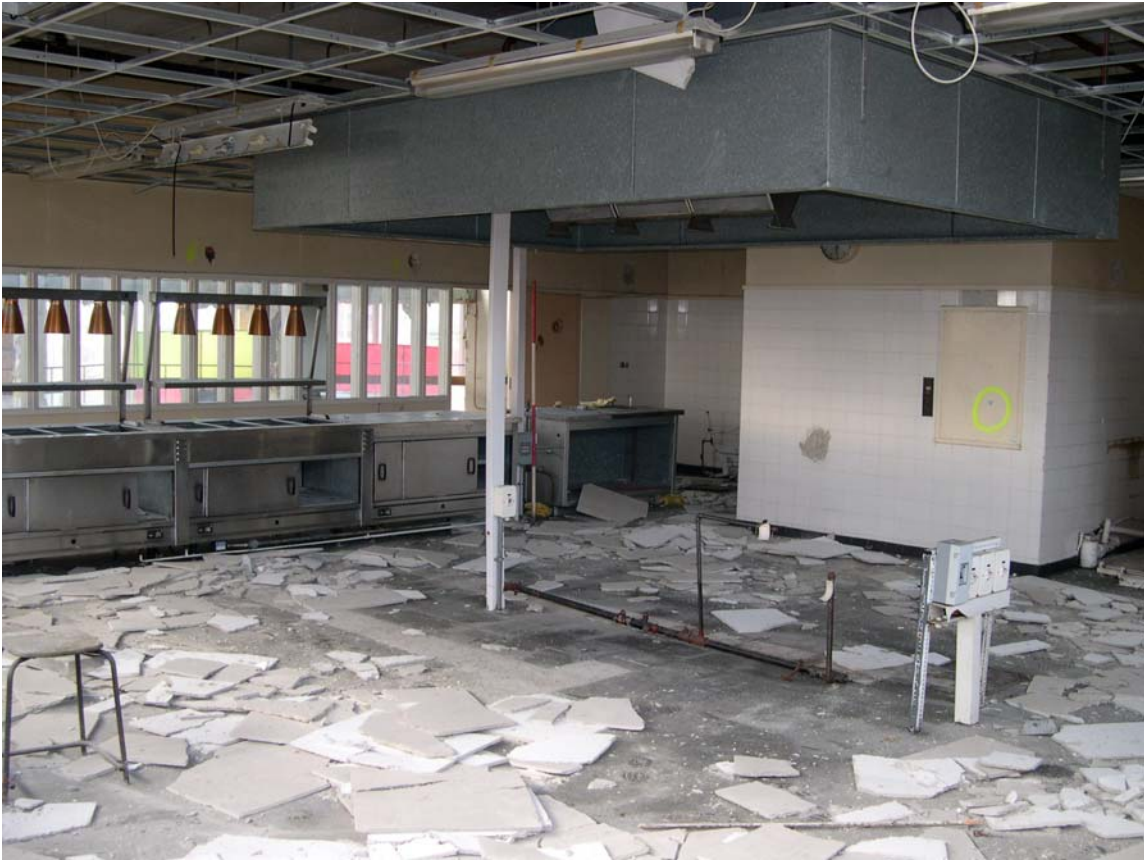
Plate 14: North-west aspect of Kitchen No.4, Room 209, Second Floor
