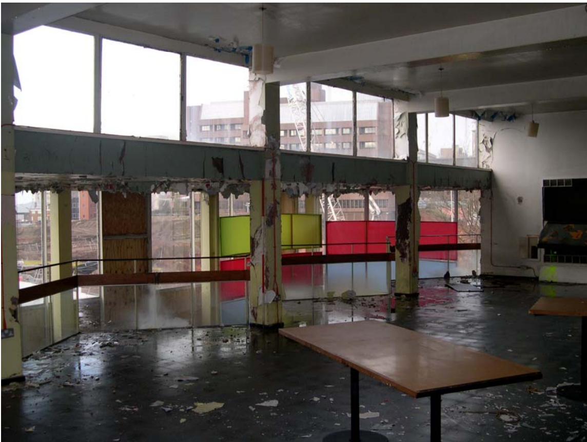
Plate 15: North-west aspect of the Refectory (Room 210), Second Floor
