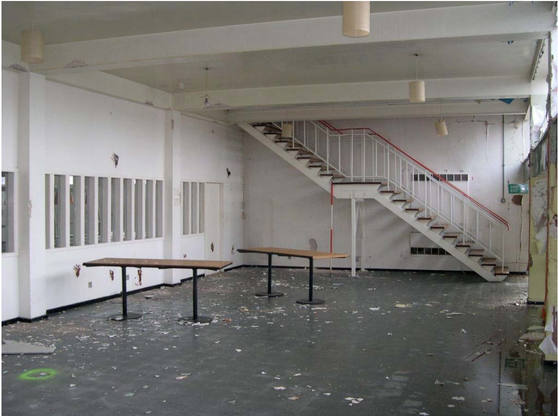
Plate 16: South aspect of the Refectory (Room 210), Second Floor
