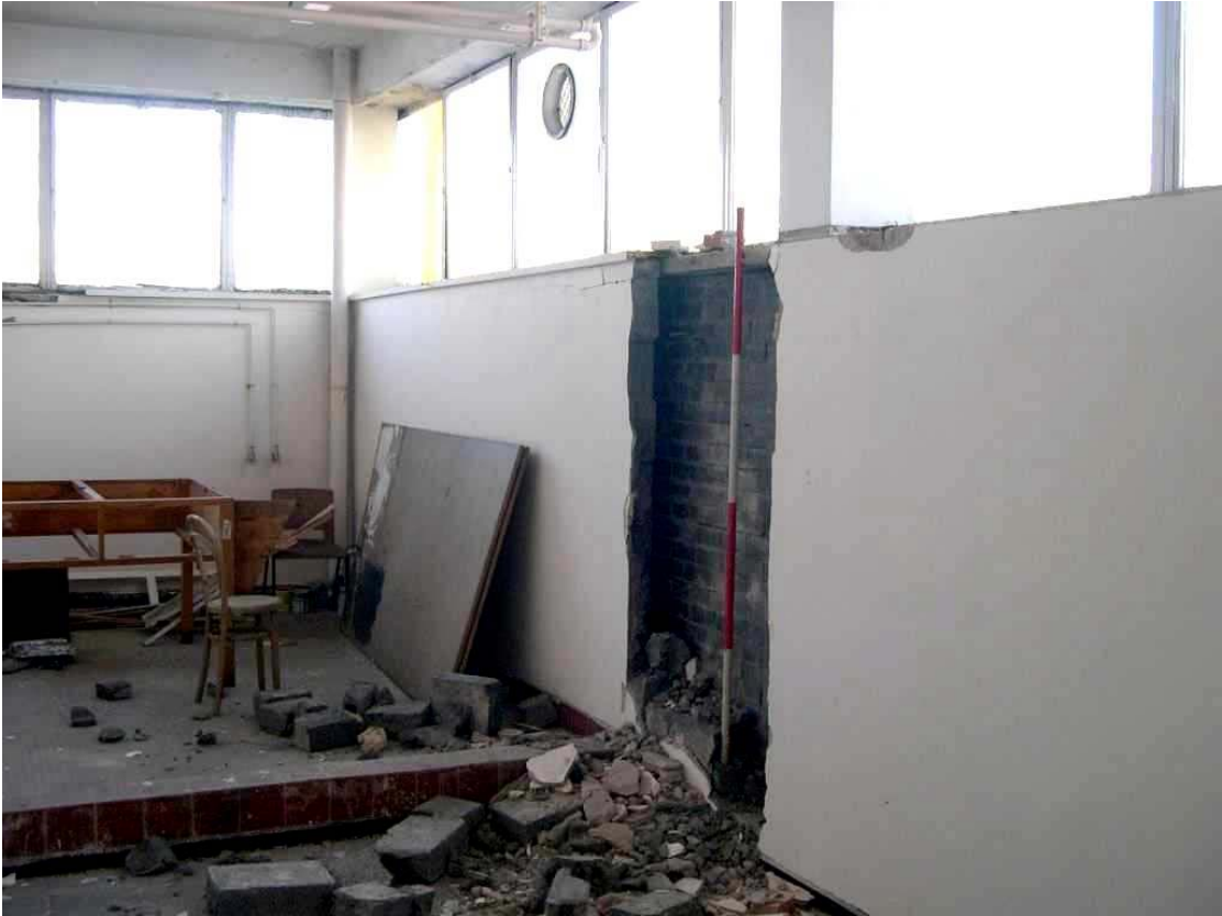
Plate 20: North-west aspect of Room 306 (Third Floor) showing the detail of external wall construction
