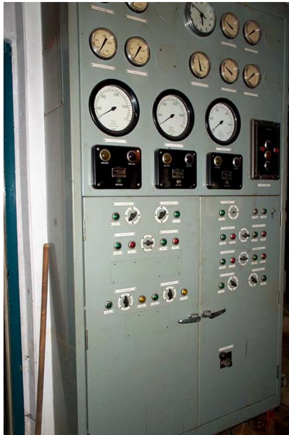
Plate 23: Thermostat, located on Ground Floor
