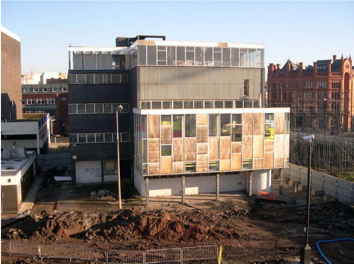
Plate 1: West external elevation of the Nautical Catering College
