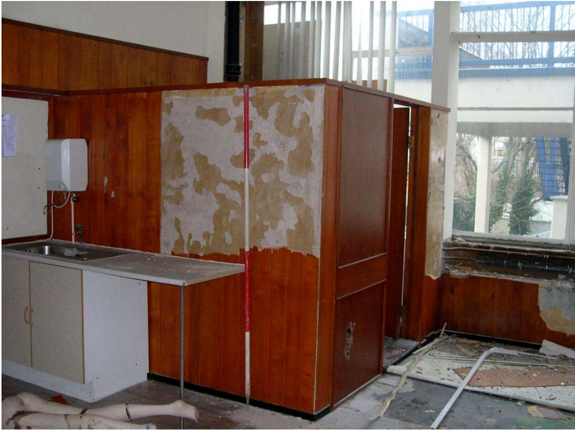
Plate 7: Partitioned area within the cabin lounge (Room 101), First Floor
