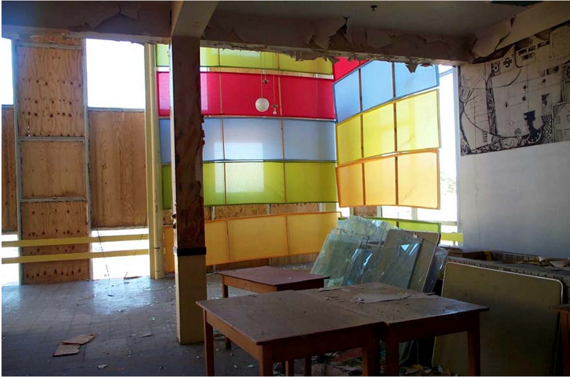
Plate 9: North-west aspect of the main dining salon (Room 110), First Floor
