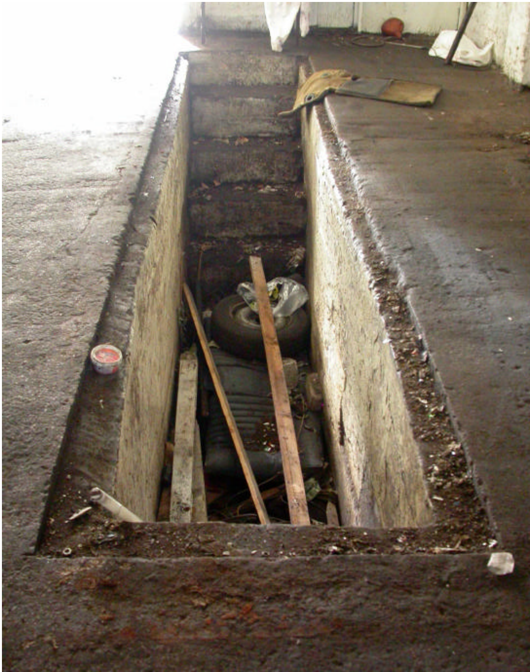
Plate 6: Inspection Pit on the Ground Floor
