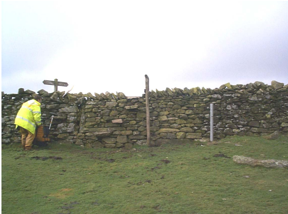
Plate 4: Site 11 Blocked gateway (looking west)
