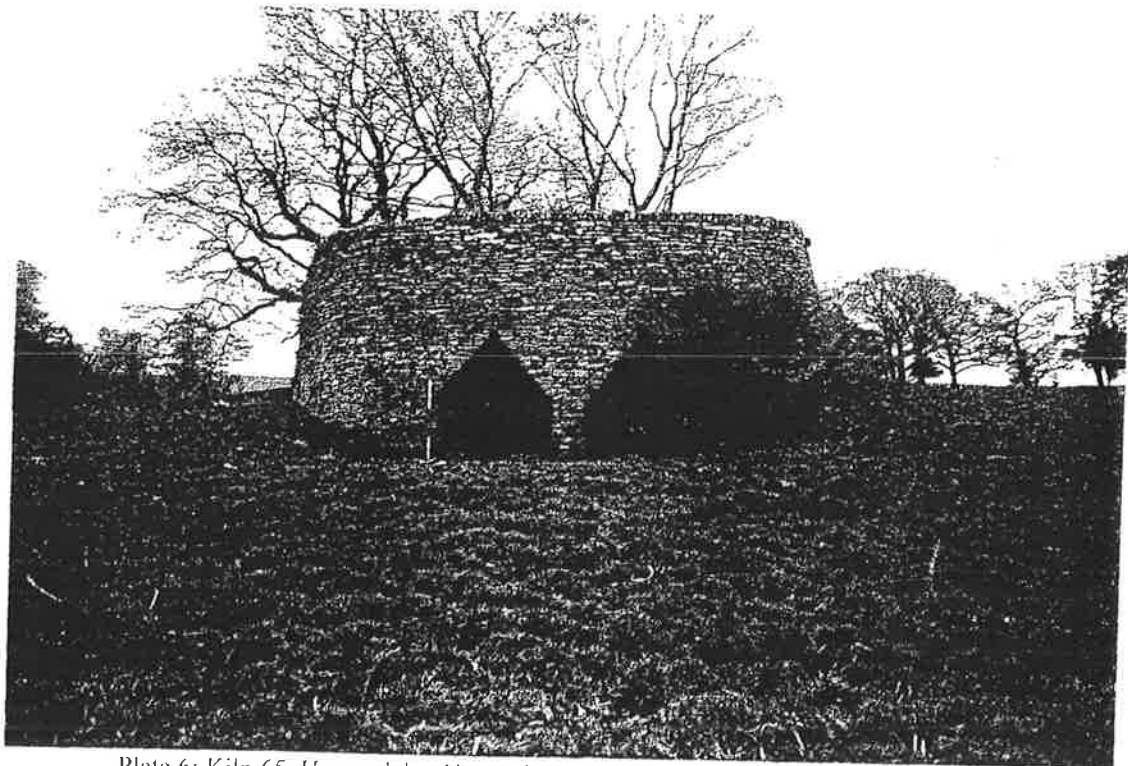
Plate 6: Kiln 65, Harsondale. Unusual double pointed arches in a quarry complex.
