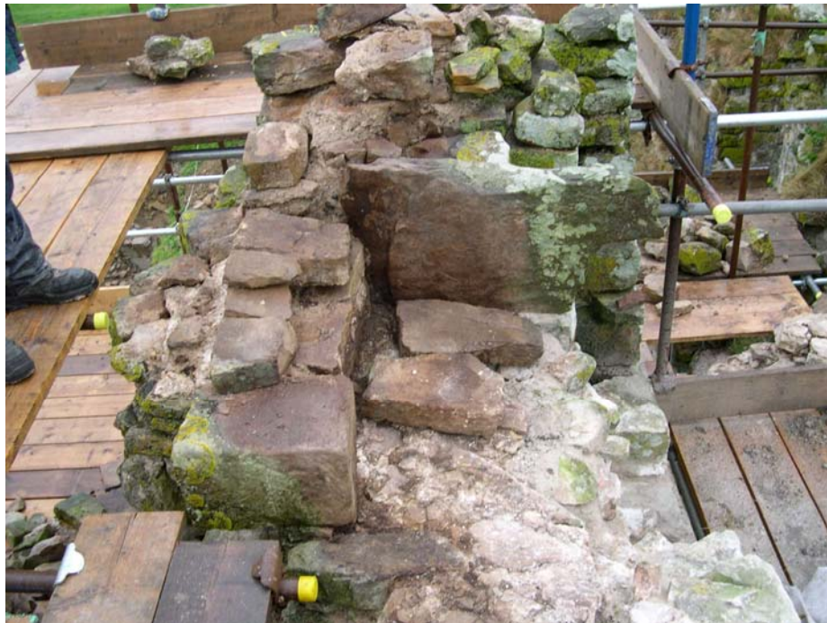
Plate 15: Sandstone jamb and passage to the parapet-level garderobe, south elevation of the barbican
