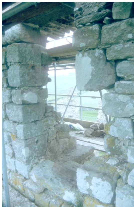
Plate 20: Jamb of eastern Phase 3 window, showing sockets for glazing bars
