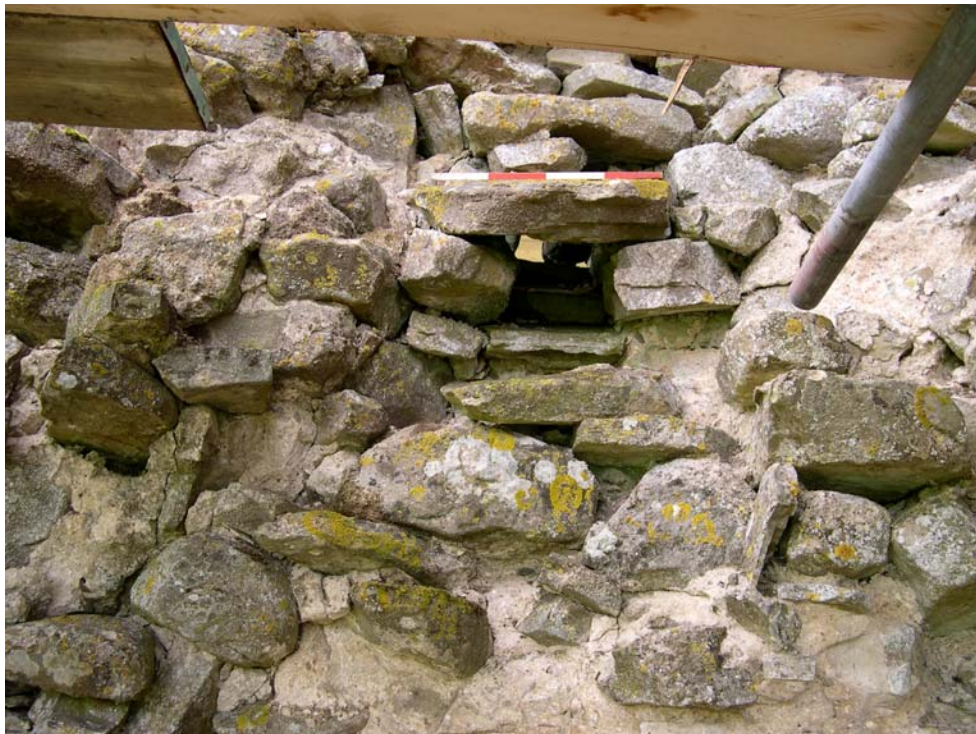
Plate 9: Probable loophole, west curtain wall, external face
