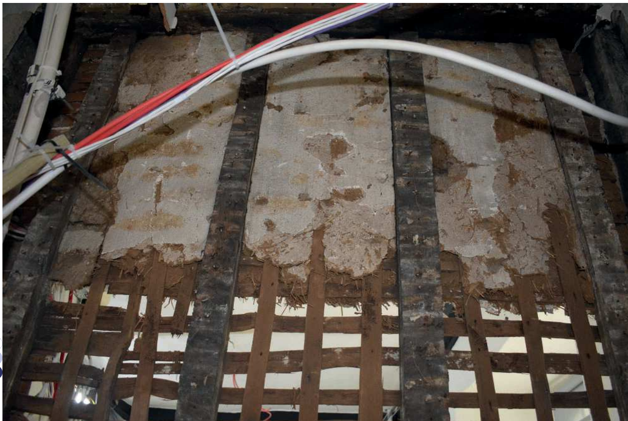
Plate 5: Historic plaster to west side of frame
