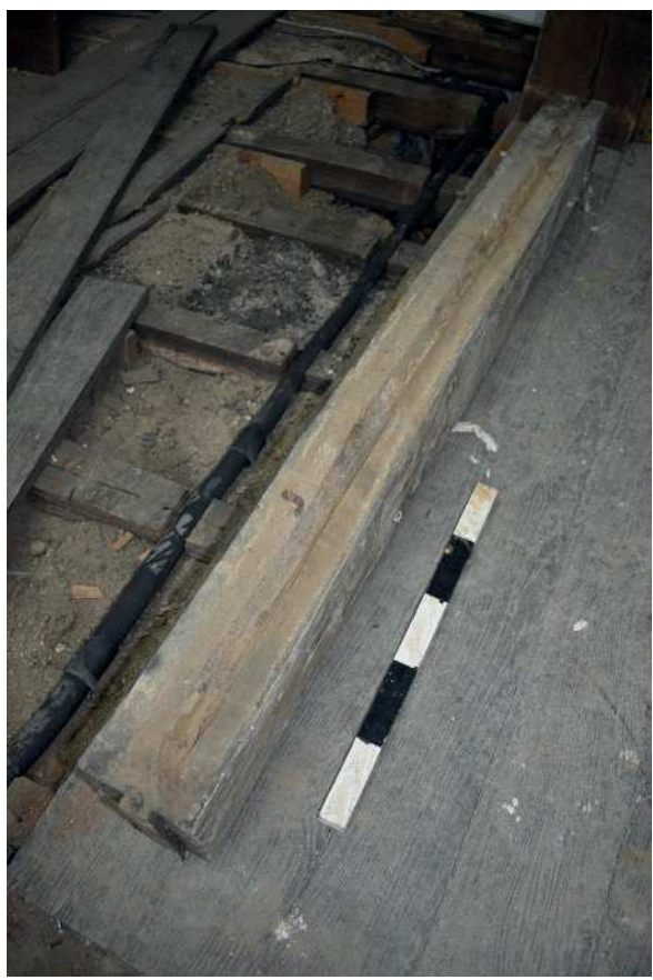
Plate 9: Groove in sill after dismantling of frame
