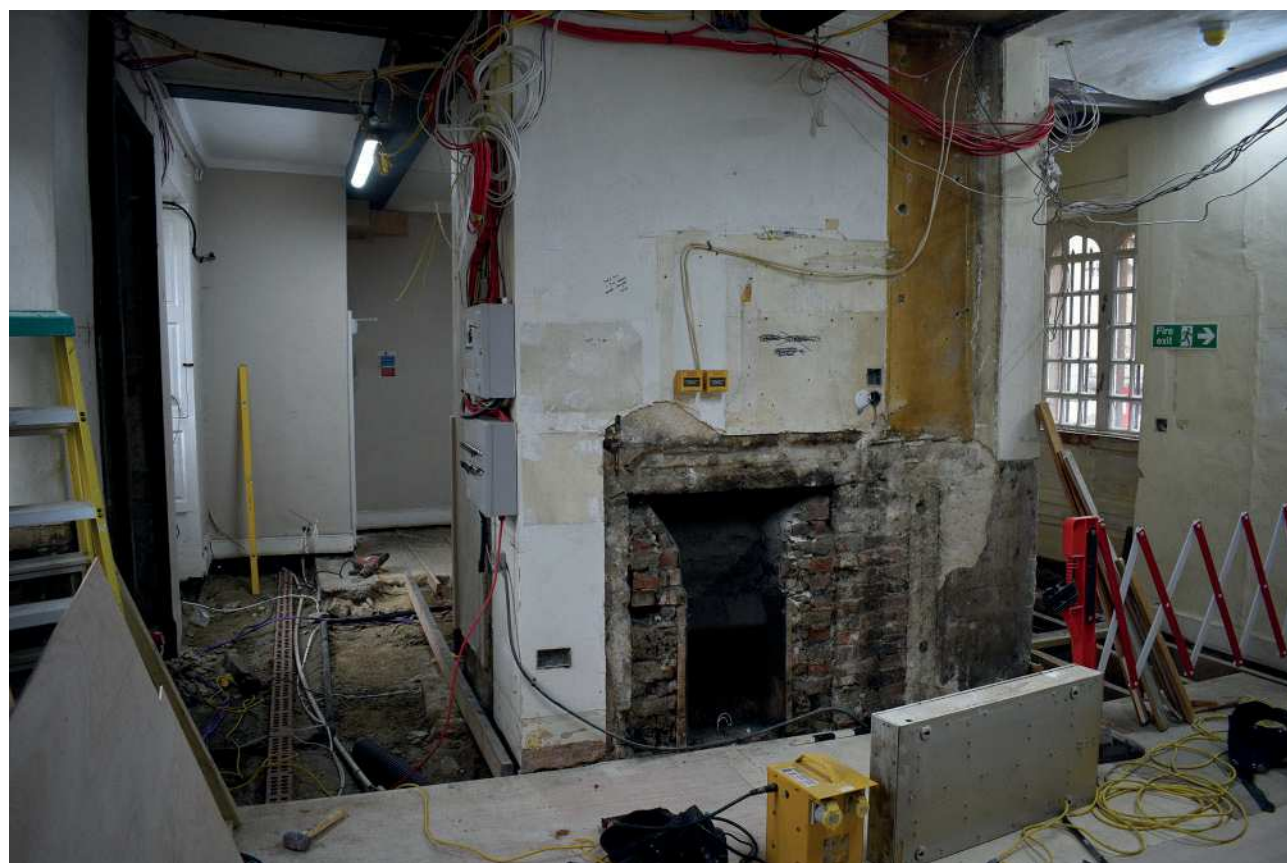
Plate 18: Fireplace exposed by works on west side of Porters' Room
