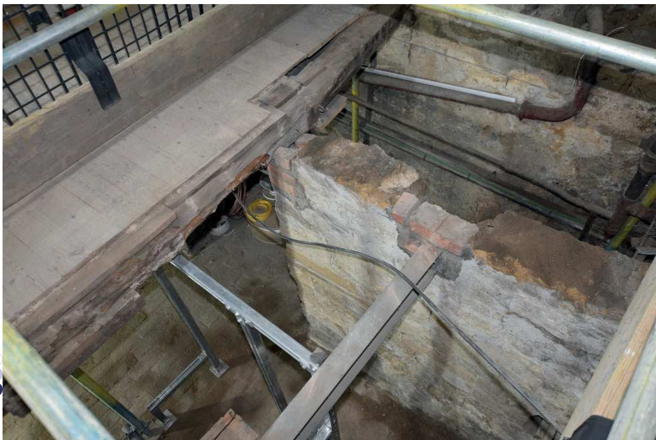
Plate 35: Eastern cellar after removal of ground floor joists
