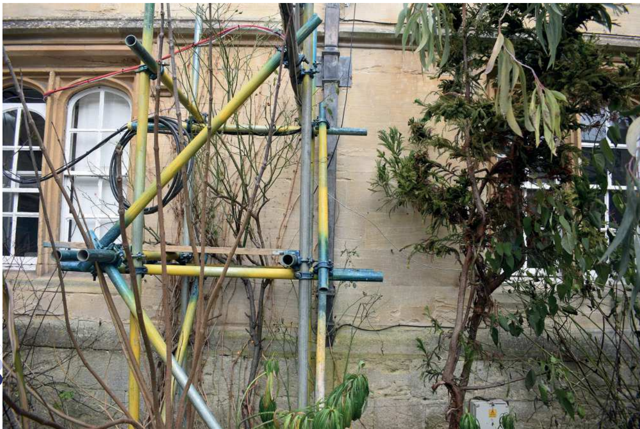
Plate 15: Refaced external wall in location of former window
