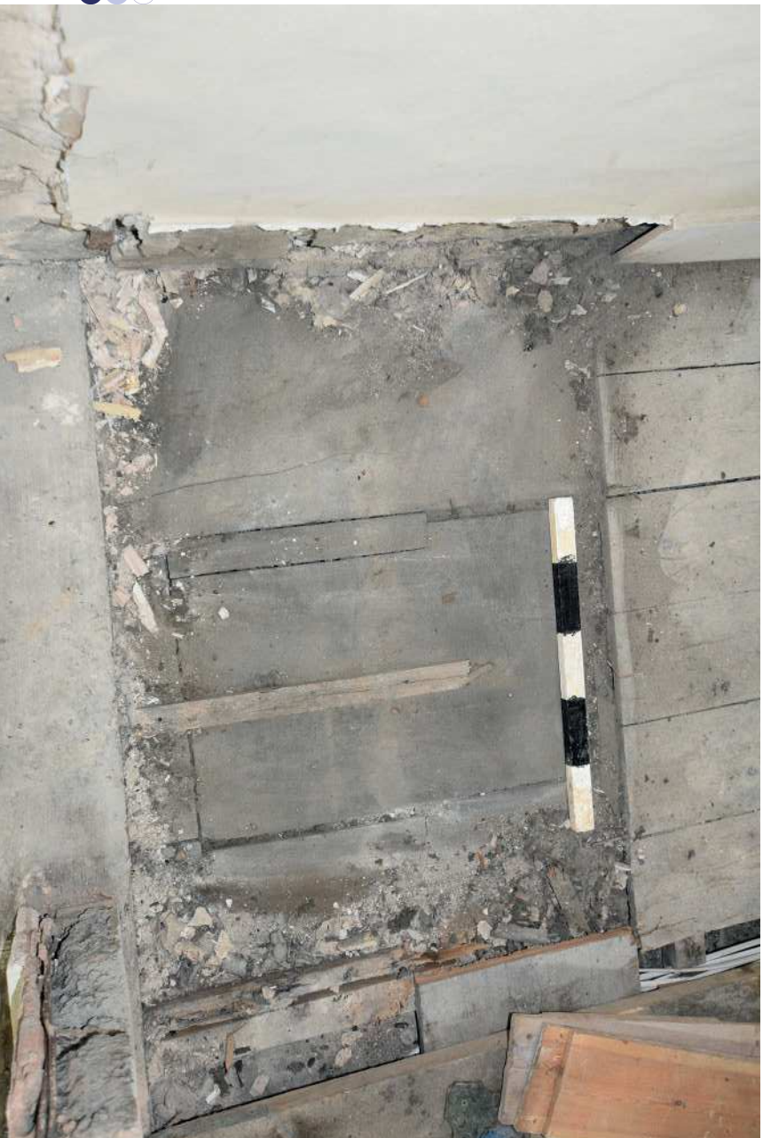
Plate 51: Wide early floorboards exposed in WC beneath later boards
