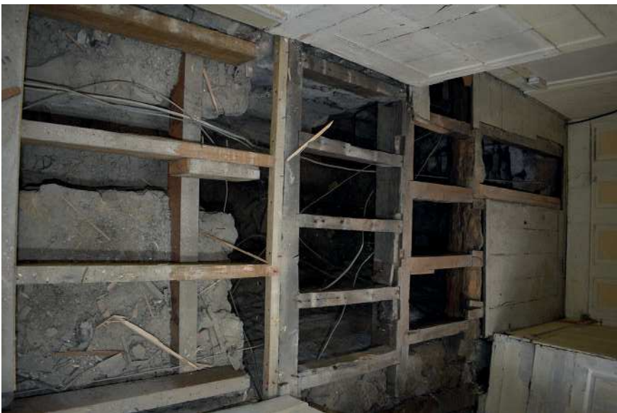
Plate 39: Floor joists over cellar (looking west)
