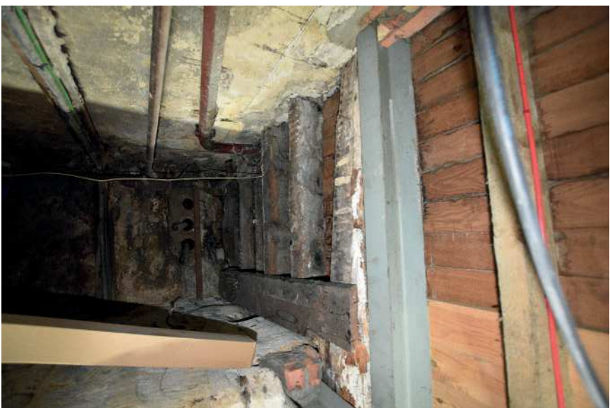
Plate 33: Eastern bay of cellar
