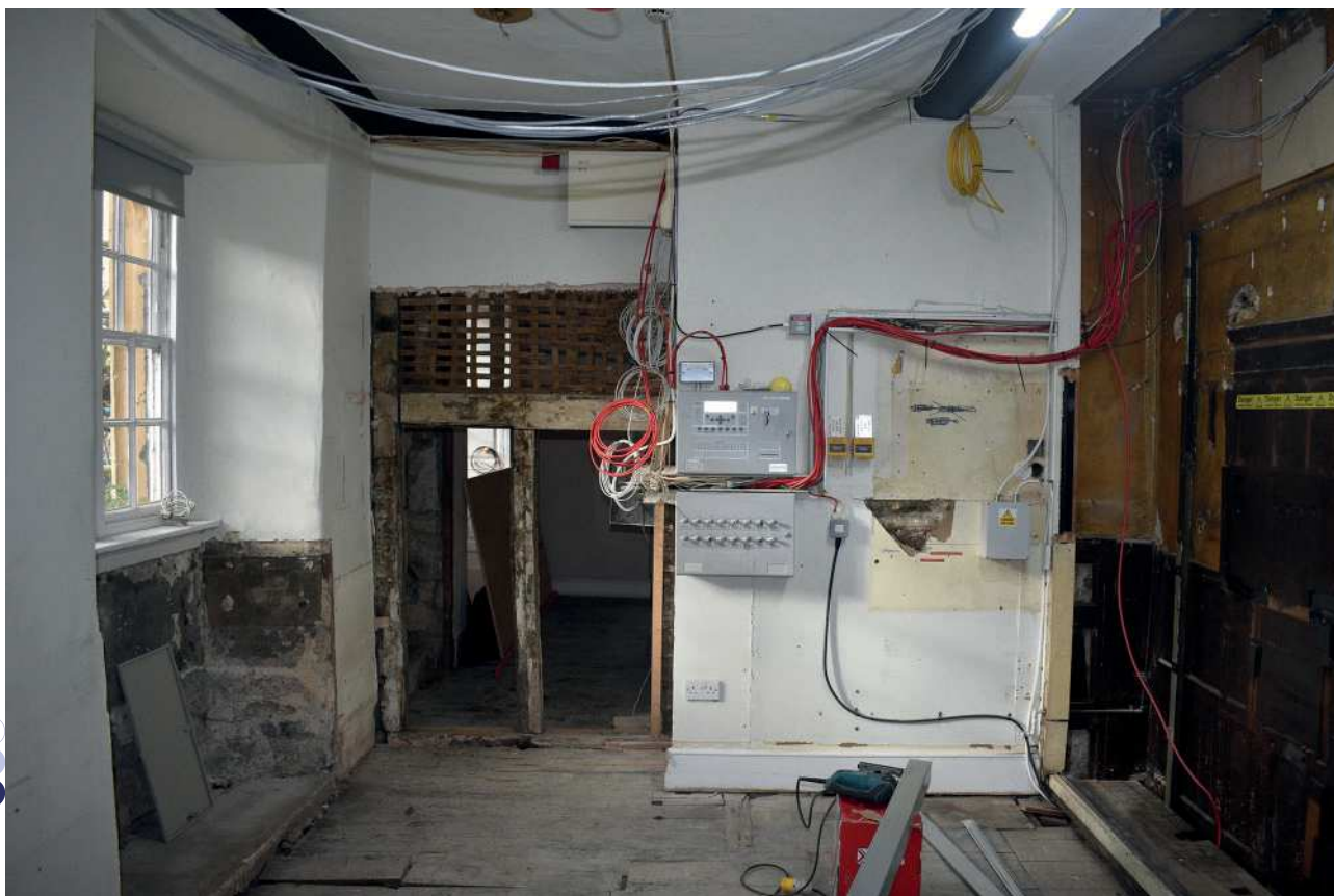
Plate 1: Porters Room (G1) looking west with partition frame exposed
