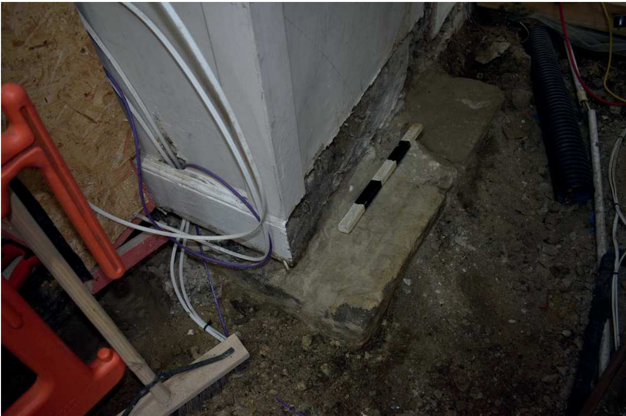
Plate 12: Footing by chimney after removal of frame
