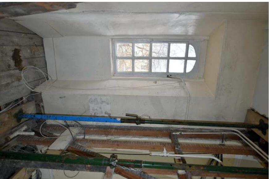
Plate 50: South wall in former first floor WC
