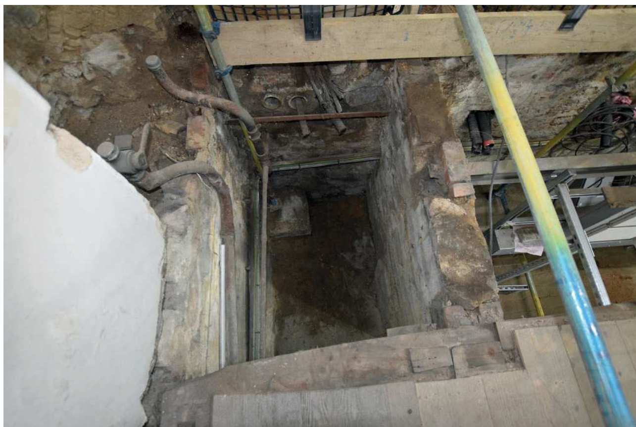
Plate 36: Eastern cellar after removal of ground floor joists
