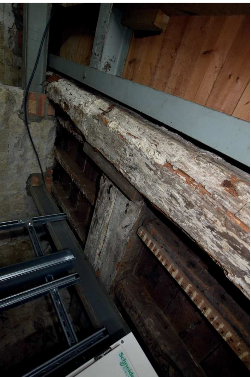
Plate 34: Floor joists in eastern cellar
