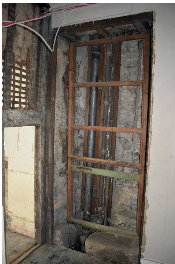
Plate 13: Location of former blocked window in south wall
