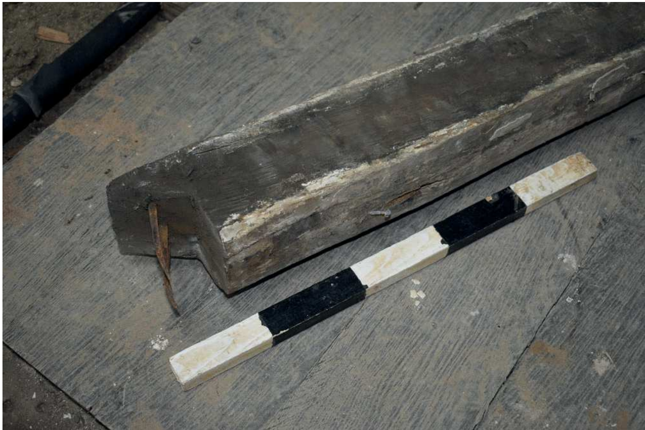
Plate 10: Secondary nailed door post after dismantling of frame
