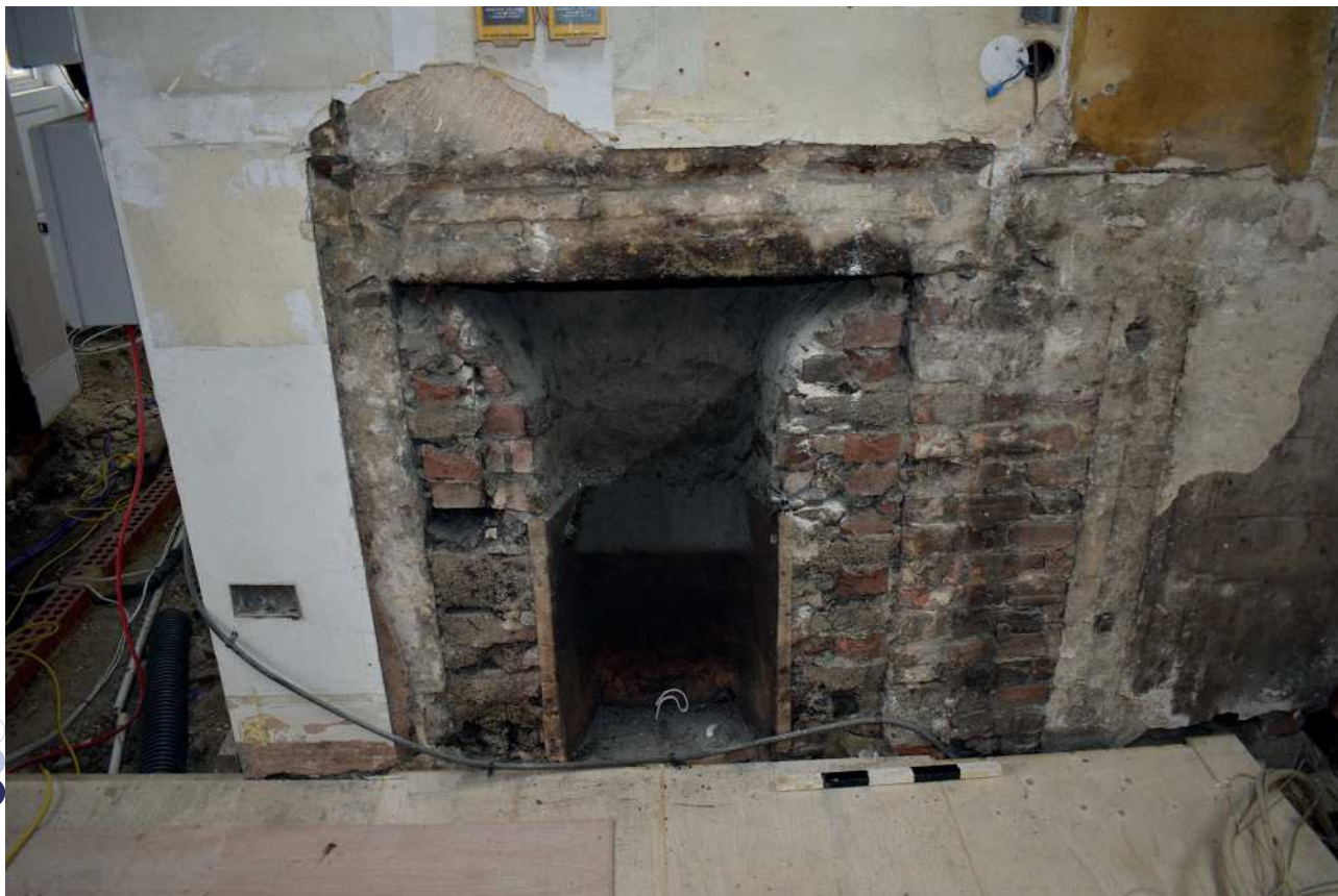
Plate 19: Fireplace exposed by works on west side of Porters' Room
