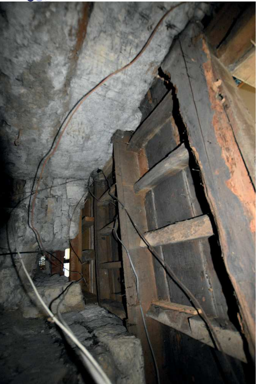
Plate 41: Western cellar looking east
