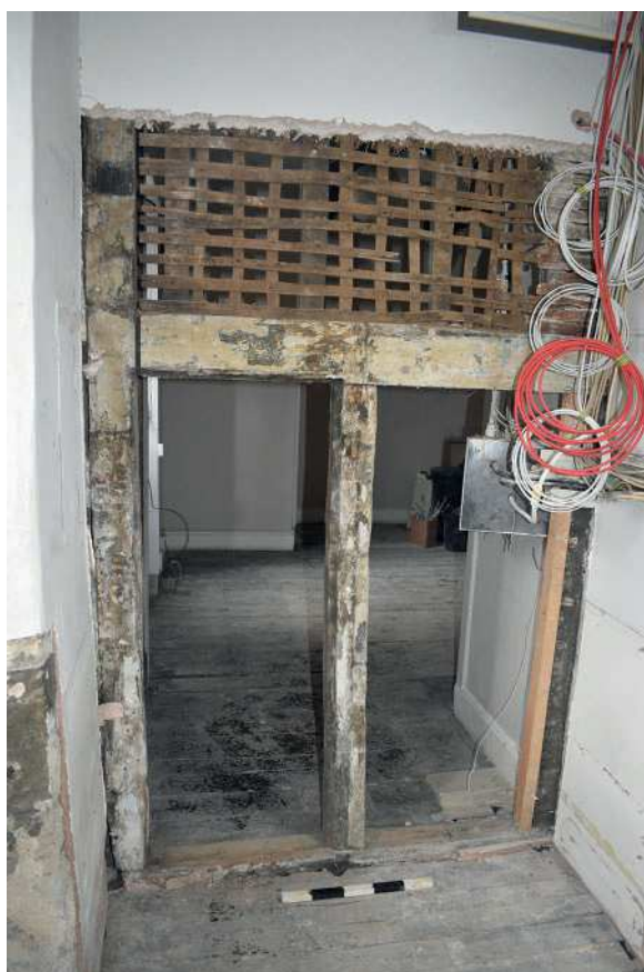
Plate 2: East side of exposed frame
