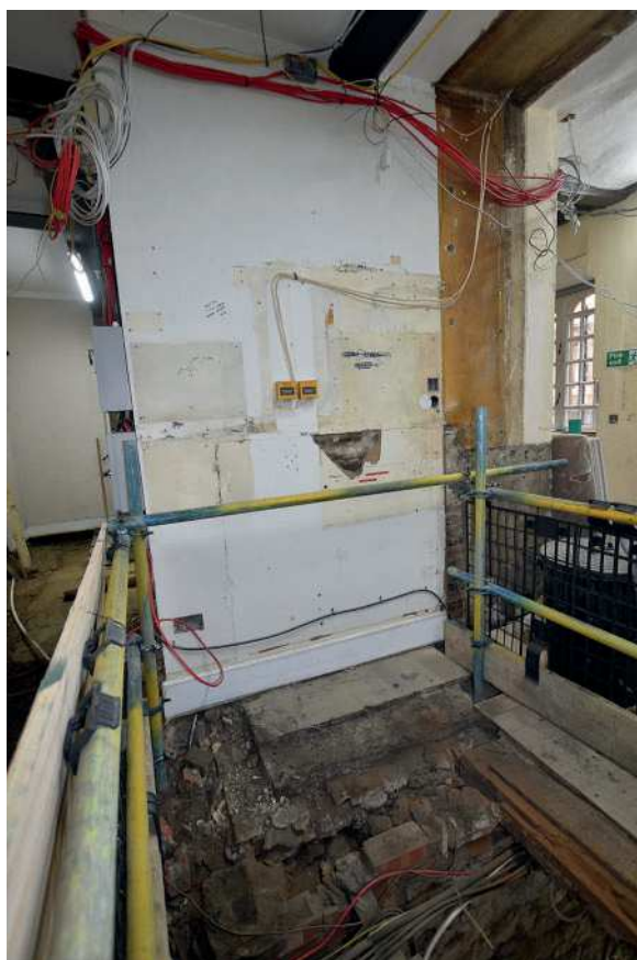
Plate 17: West side of Porters' Room during works
