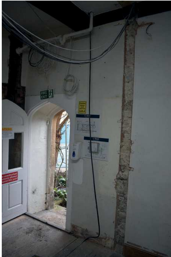
Plate 27: South-east corner of Porters' Lodge after removal of wall
