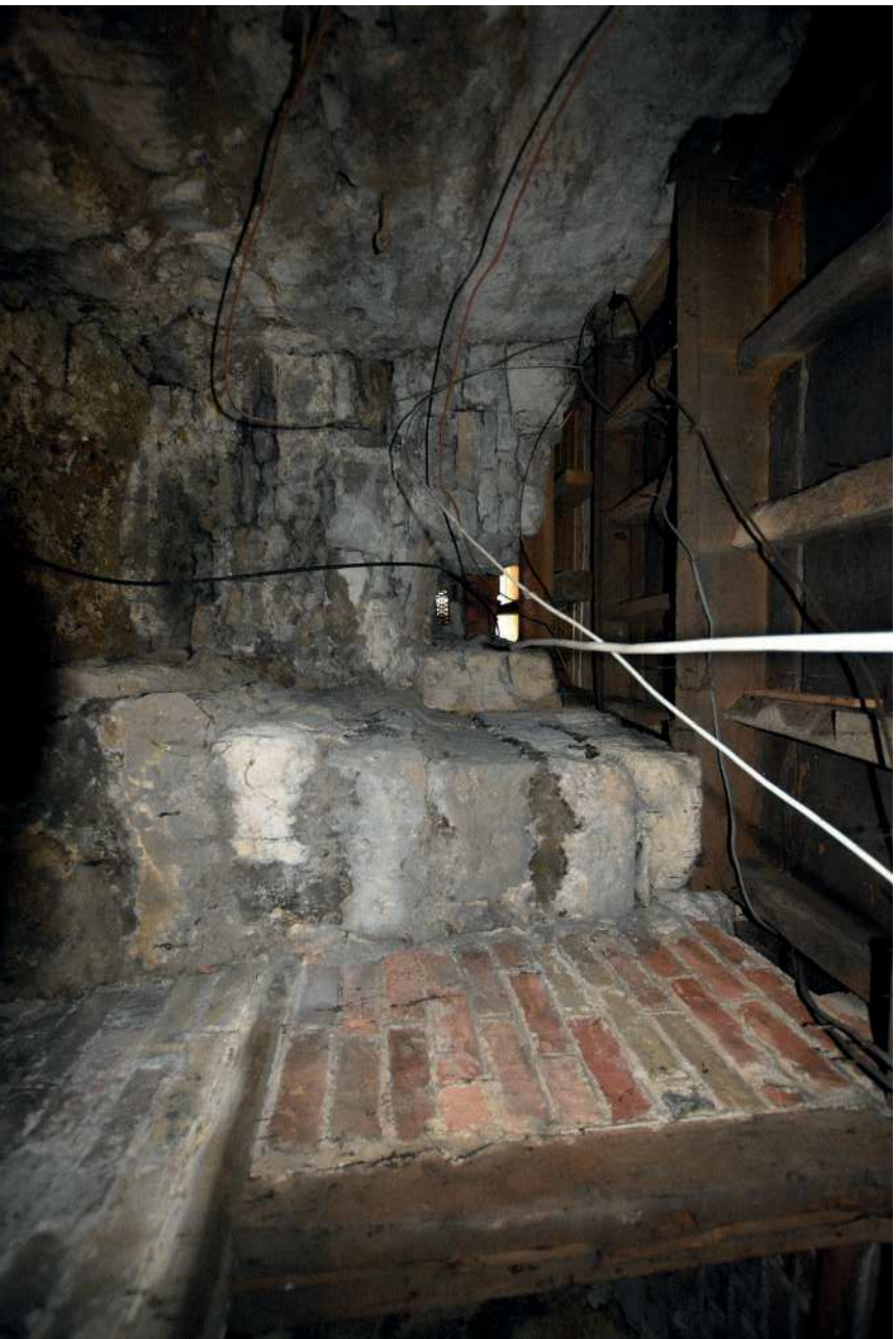
Plate 40: Western cellar looking east
