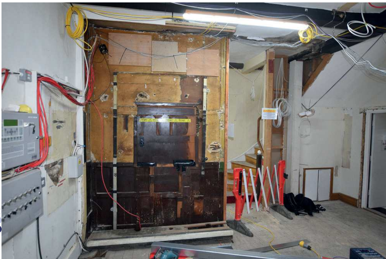
Plate 21: Panel on north side of Porters' Room exposed during soft strip
