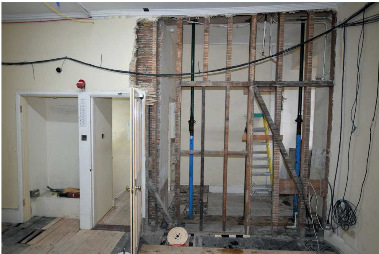
Plate 48: Exposed first floor partition looking east
