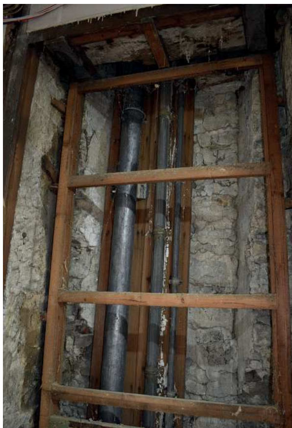
Plate 14: Location of former blocked window in south wall
