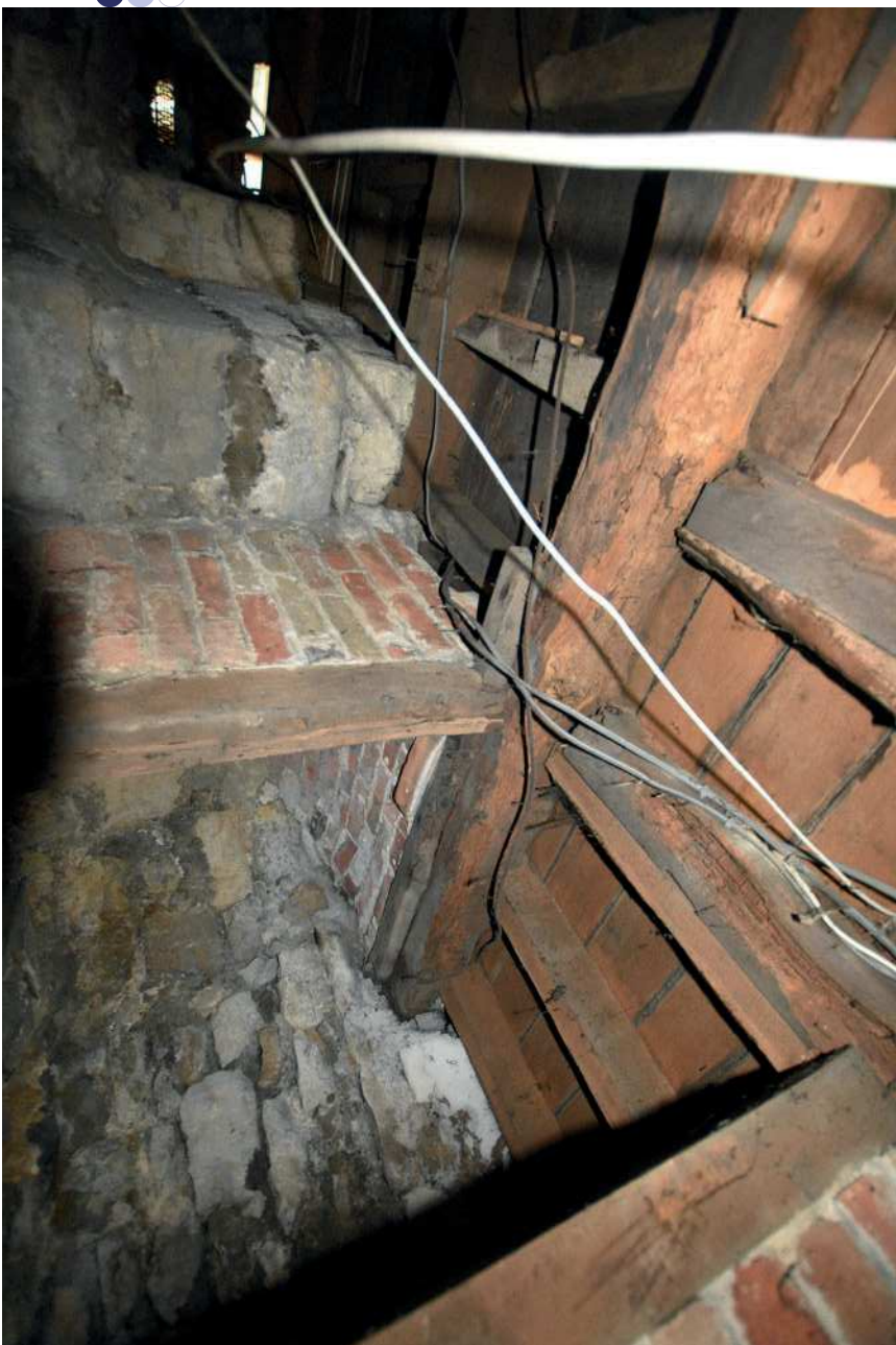
Plate 43: Western cellar looking south
