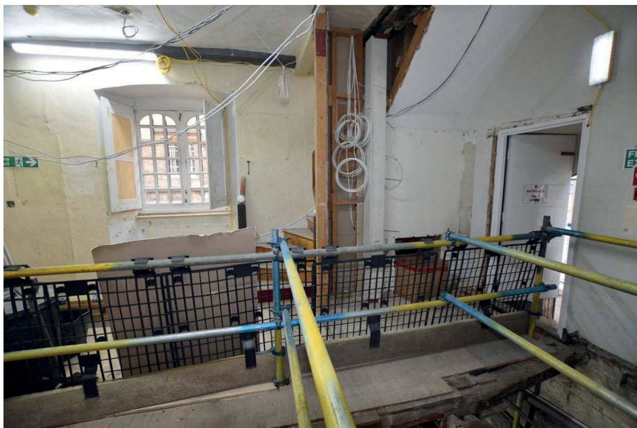
Plate 24: North side of Porters' Room during soft strip
