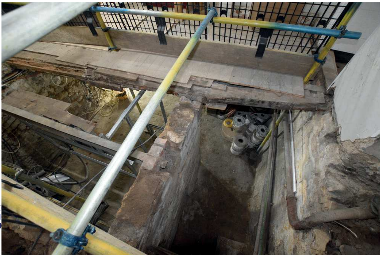
Plate 37: Eastern cellar after removal of ground floor joists
