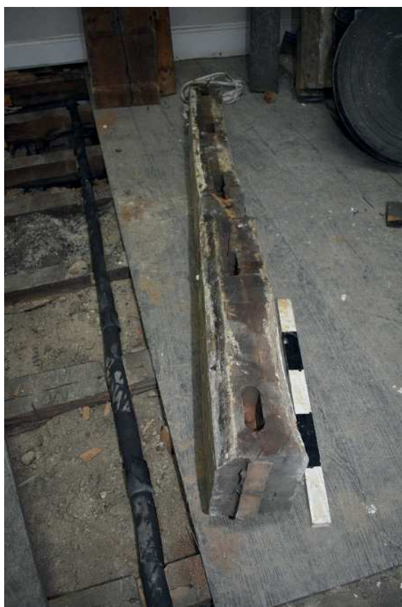
Plate 8: Mortises in underside of rail after dismantling of frame
