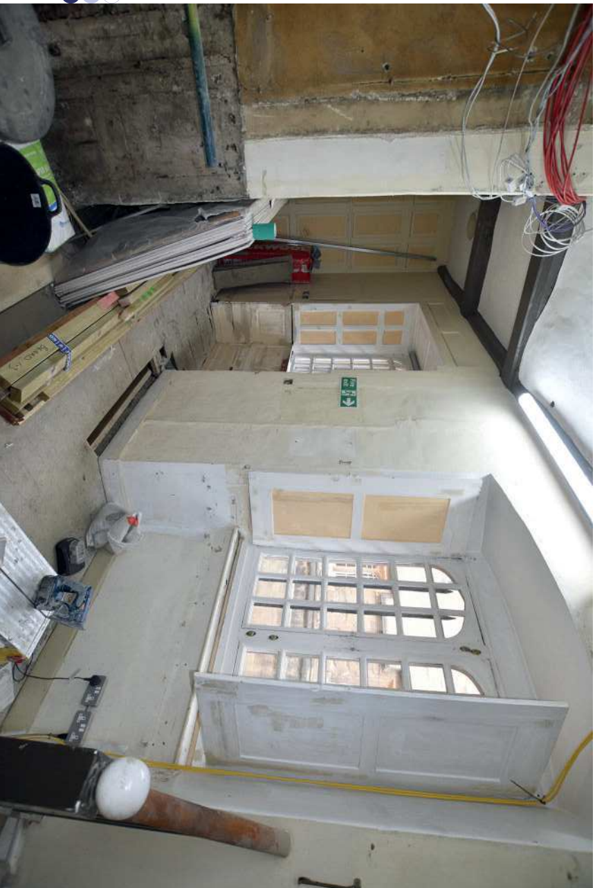
Plate 25: North wall after removal of panel
