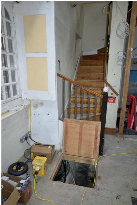
Plate 28: Hatch in floor towards north-east corner of Porters' Lodge
