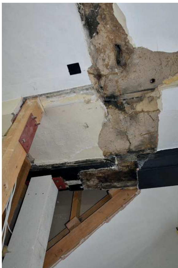
Plate 23: Line of early plaster to ceiling where panel removed
