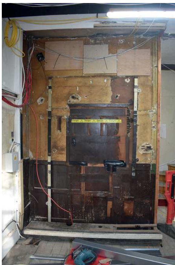
Plate 20: Panel on north side of Porters' Room exposed during soft strip
