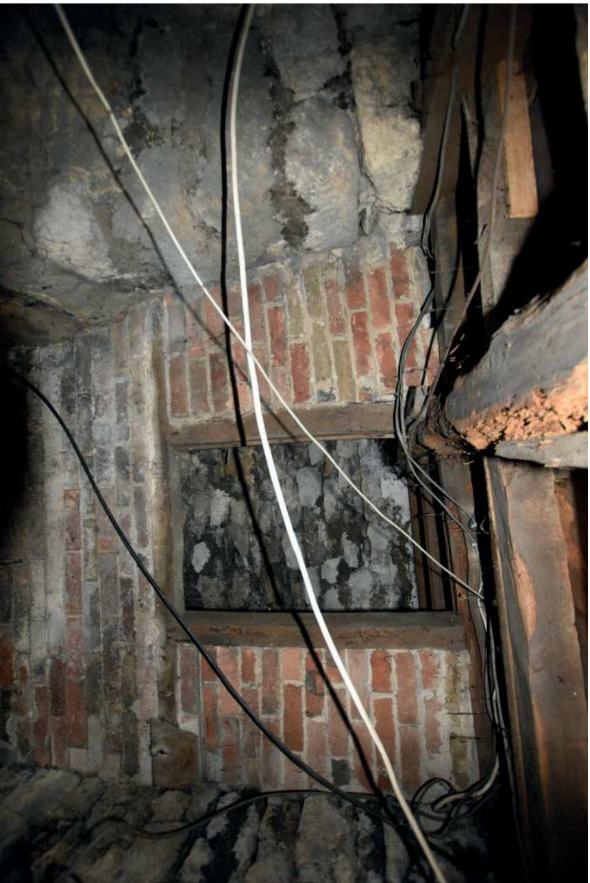
Plate 42: Western cellar looking south
