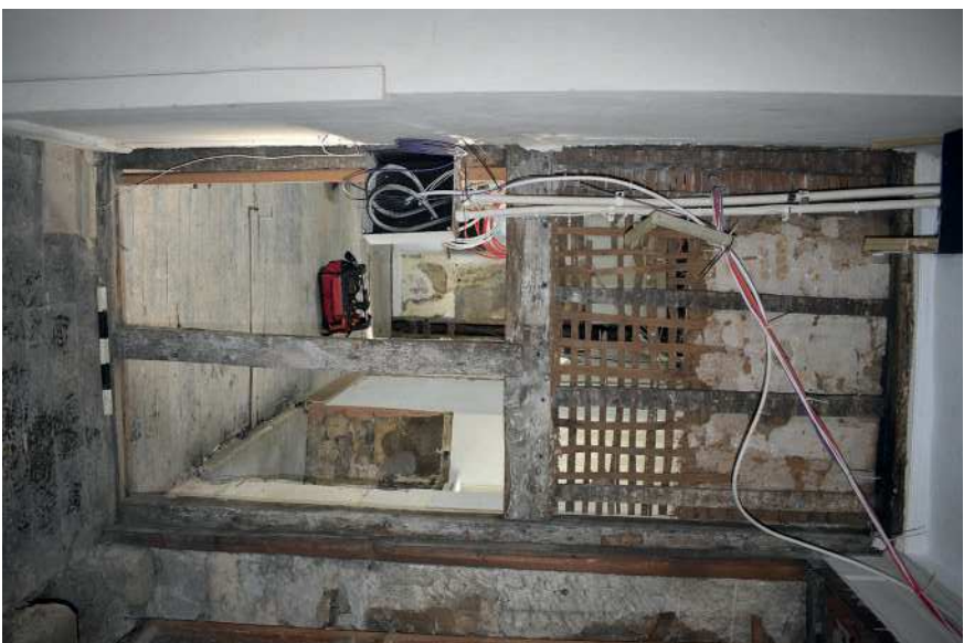
Plate 3: West side of exposed frame
