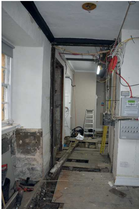
Plate 11: View looking west in Porters' Room after removal of frame
