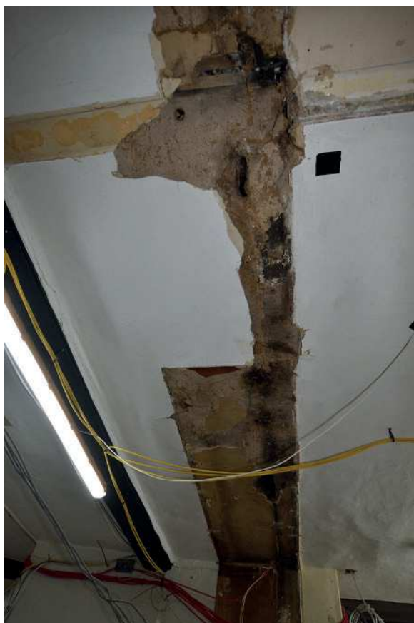
Plate 22: Line of early plaster to ceiling where panel removed
