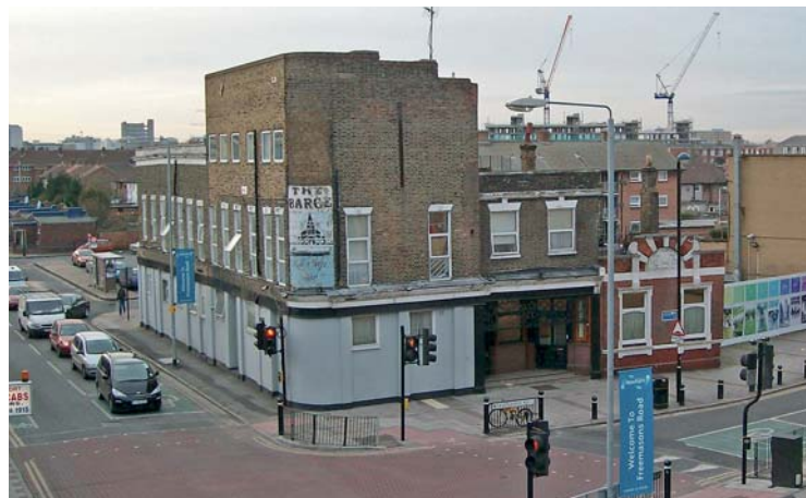
Fig 103 The Barge – formerly The Freemasons Tavern 2009
