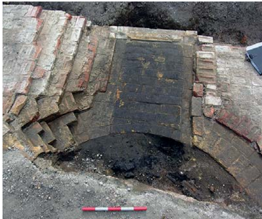
Fig 53 White Hart Depot: detail of the central area of the chimney structure, showing two solid brick bases to either side of a blackened area, which was an opening into the chimney for access
