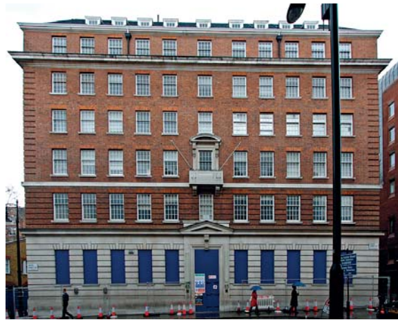
Fig 90 Exterior view of No. 65 Davies Street
