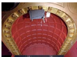
Fig 41 No. 148 Charing Cross Road: detail of the coffered vaulted ceiling
