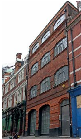
Fig 36 Exterior view of Nos 2-3 Fareham Street in 2010
