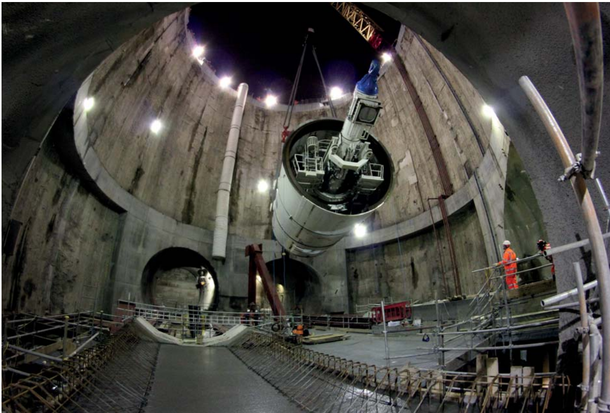
Fig 2 A Crossrail tunnel boring machine being lowered into position
