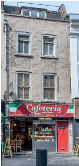
Fig 9 No. 101 Charing Cross Road (formerly No. 68 Crown Street) is one of only a handful of early houses to have survived the construction of Charing Cross Road in the late 19th century
