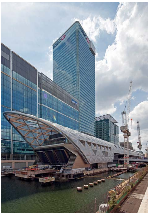
Fig 107 Crossrail's new Canary Wharf Station, May 2014
