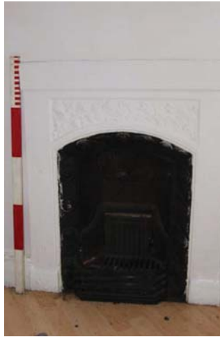
General view of 9 Diadem Court (left) 2010; detail of fireplace (right)
