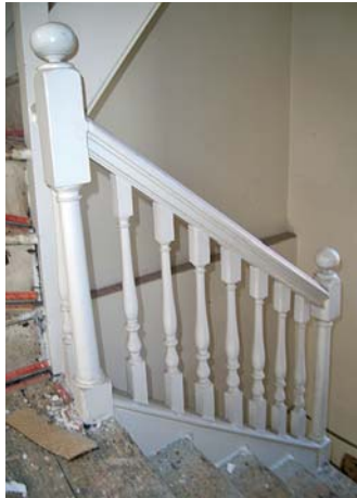
94 Dean Street, facing south-west (left) 2003; closed string staircase (right)
