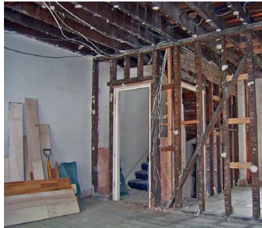
Fig 21 (right) Staircase at No. 94 Dean Street at first floor level, facing south
