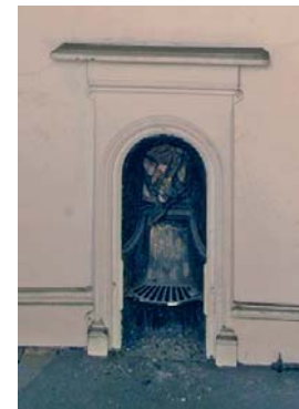
Fig 43b No. 7 Oxford Street: original fireplace on the fourth floor
