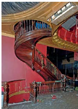
Fig 40 No. 148 Charing Cross Road: the spiral staircase at first floor level
