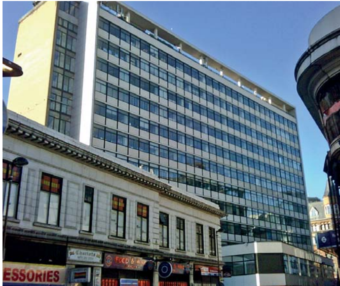
Cardinal House, Farringdon Road elevation. Facing south-west 2008
