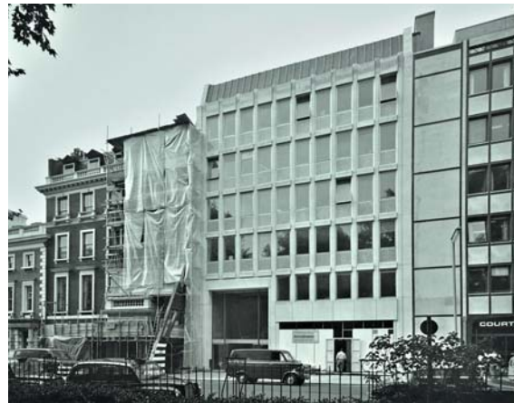
Fig 46 Nos 18 and 19 Hanover Square in 1973, modern steel framed buildings
