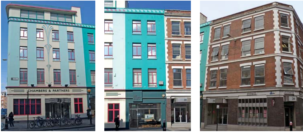
23 Long Lane/2 Lindsey Street (left), 22 Long Lane (middle), 20-21 Long Lane (right) 2009
