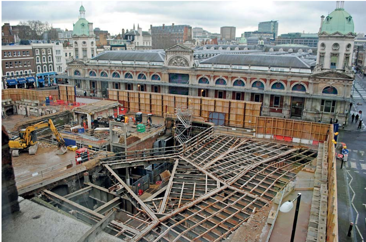
Fig 67 The demolition of Nos 54-64 Charterhouse Street (Smithfield House) revealed the steel decking structure that had suspended the building over the railway lines below
