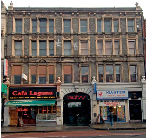
Exterior of 142 and 146 Charing Cross Road, facing east 2009
