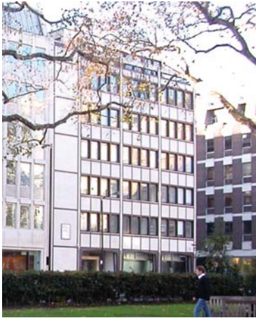
East facing elevation of 18 Hanover Square
