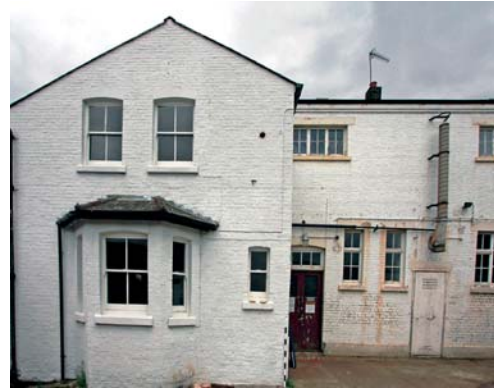
Fig 76 The former East London Soap Works, Bow; probable staff house and attached office building
