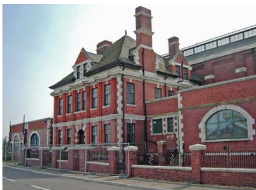
Fig 49 View of White Hart Depot main building looking from North Road
