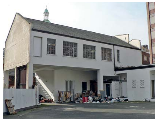
Fig 66 Nos 54-64 Charterhouse Street (Smithfield House) rear view
