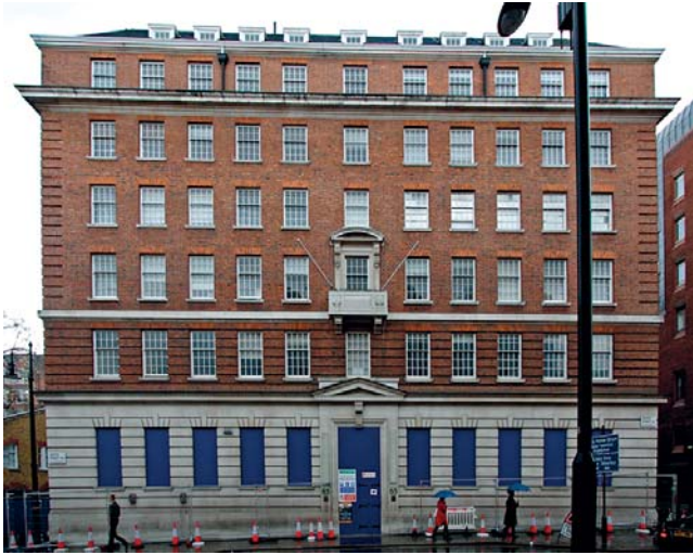
65 Davies Street, Davies Street elevation. Facing south-west 2010
