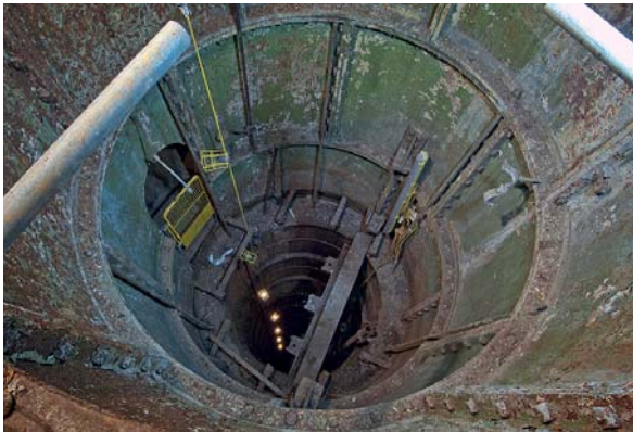
Fig 70 Lined shaft of the artesian well revealed during excavations for Crossrail at the Albion Brewery, Whitechapel
