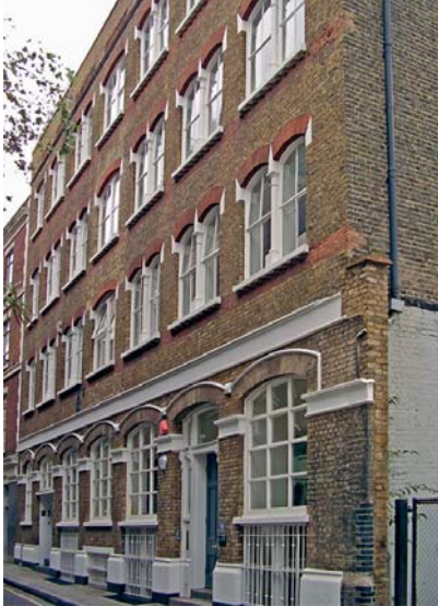
Hayne Street facade facing west 2010
