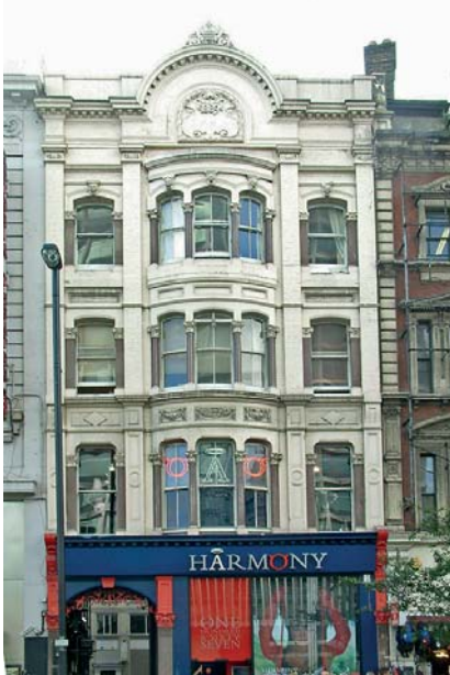
Exterior of 167 Charing Cross Road, facing west 2004
