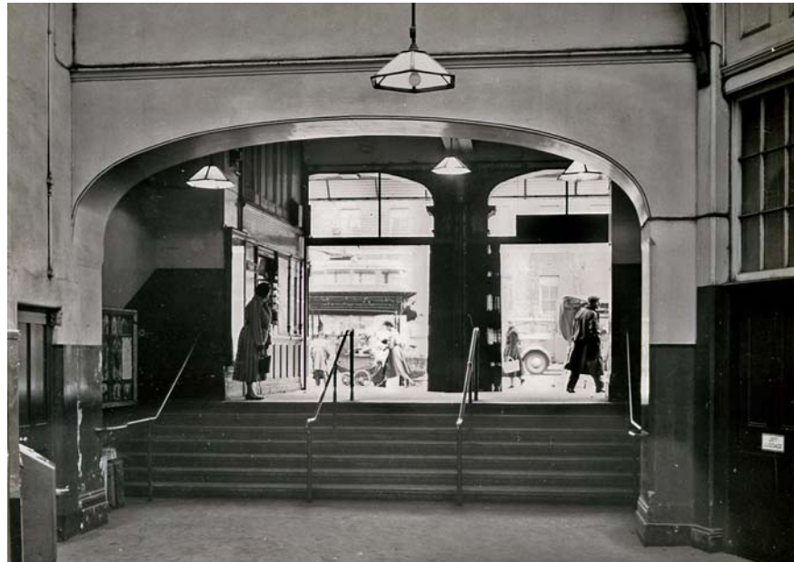
Fig 43 The ELR's Whitechapel station booking hall looking south to Whitechapel Road in 1957. The elliptical arch probably helped spread the load of the buildings overhead. (Collection of London Transport Museum, Image no: 440/199. © Transport for London)
