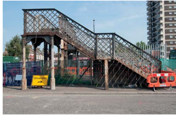
Henley's Footbridge, looking west (left) and north (right). Note replacement steel column
