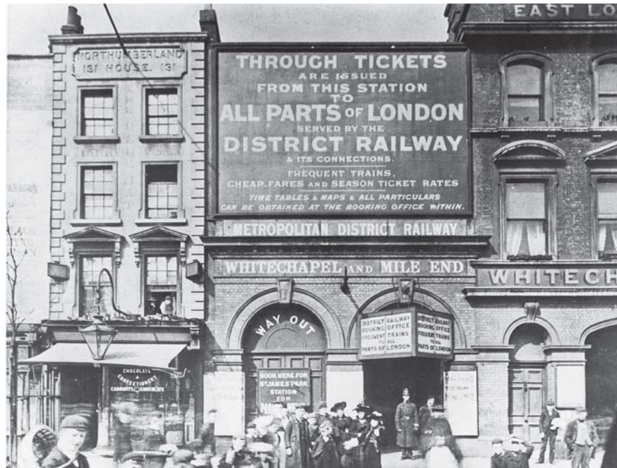
Fig 39 The MDR Whitechapel Road station entrance in 1896, with part of the ELR station entrance to the right (Tower Hamlets Local History Library and Archives).
