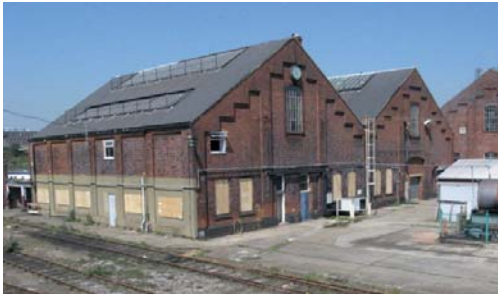
External view of the Stores looking north-west
