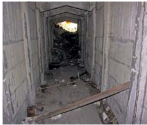
Fig 97 An internal view of Shelter 2 at Plumstead Goods Depot, looking east
