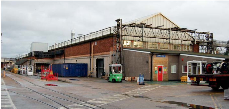
Ilford Depot's Workshop B, facing east
