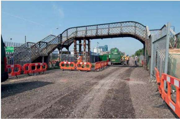
Henley's Footbridge, looking west (left) and north (right). Note replacement steel column
