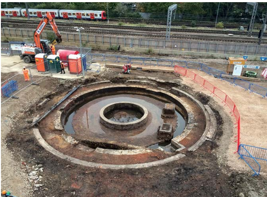
Fig 19 The concentric rings of the successive turntables which lay to the east of the NG Shed. The middle ring represented the outer wall of the earlier 40ft turntable (© Stefan Popa)
