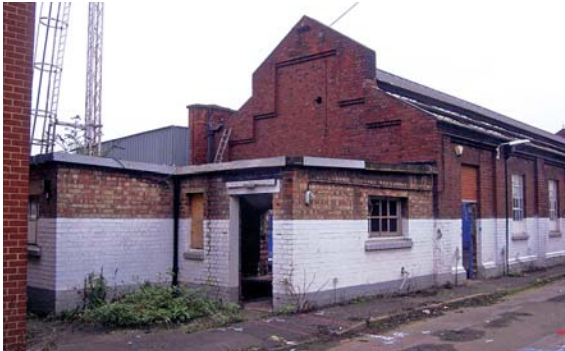
1906 sand furnace house, with mid to late 1940s extension in the foreground. Looking north-east
