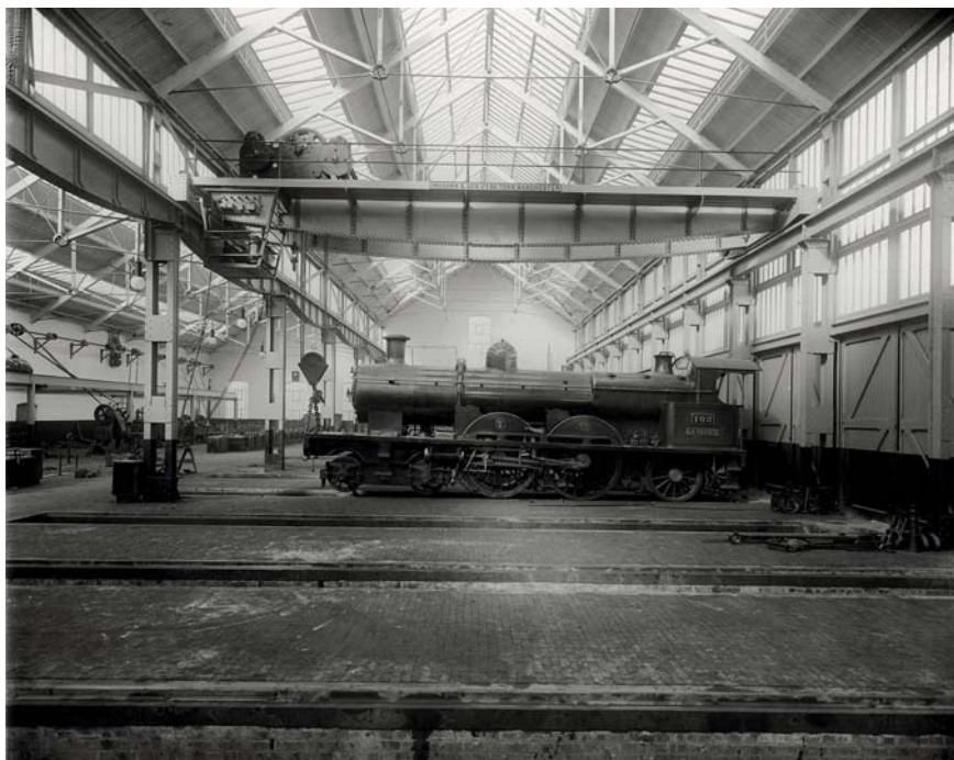
Fig 53 Old Oak Common's lifting shop is shown to good effect in a photograph probably taken not long after the depot opened in 1906. The locomotive is a Société Alsacienne de Constructions Mécaniques's four-cylinder compound which was unusual for having been bought by Churchward in 1903 specifically for evaluation purposes (NRM/ Science and Society Picture Library).
