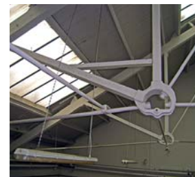
Fig 65 Cast steel junction rings in the stores building
