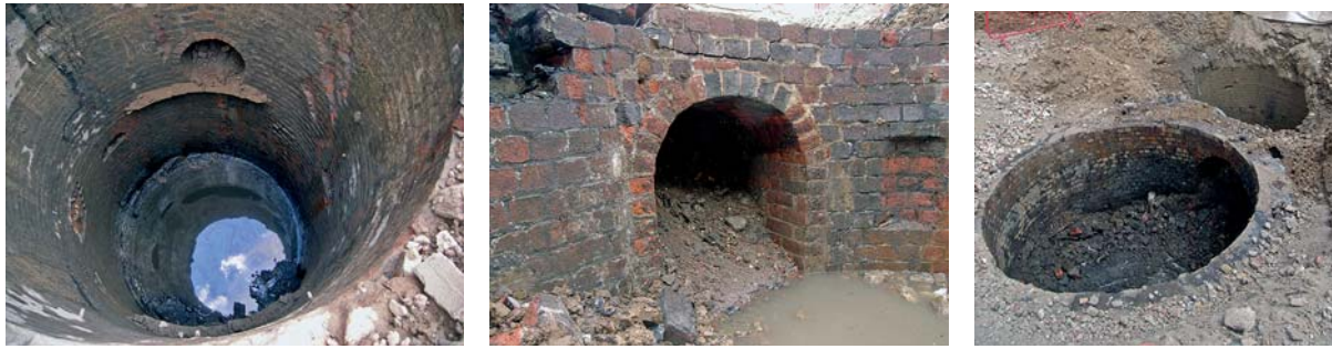
Fig 27 Westbourne Park's interconnected well shafts were exposed in 2014. Deep-level culverts linked the shafts to other nearby railway facilities
