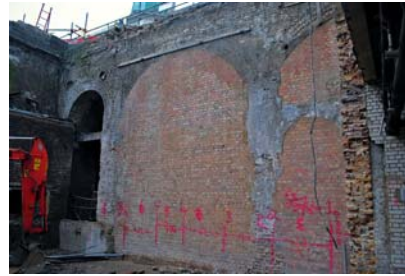
View of the rooms under 3 Lindsey Street (left), view looking west showing blocked up arches at platform level (right)
