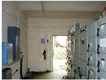
Fig 67 (left) Sign on Old Oak Common's electricity sub-station, photographed in 2010
