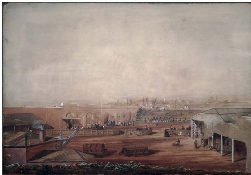
Fig 79 Paddington station in c 1840. The passenger station is to the left of the painting, the goods depot to the right (NRM/ Science and Society Picture Library)
