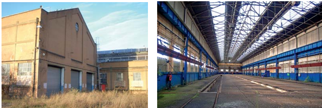
Eastern gable (left); internal view of the shed, looking west (right)
