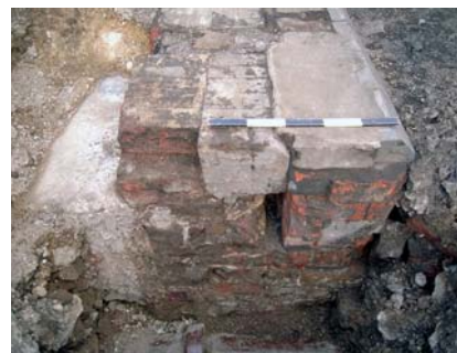
Fig 11 To allow the BG Shed to accommodate locomotives of mixed gauges the GWR reduced the width of the inspection pits by adding a brick skin to both sides of the pit. (Scale bar = 0.5m)
