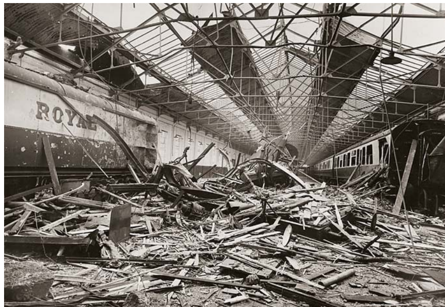
Fig 98 Old Oak Common's carriage paint shop after the air raid of 25 October 1940. The twisted pile of wreckage in the centre of the photograph is all that remained of TPO vehicle 836 (The National Archives)
