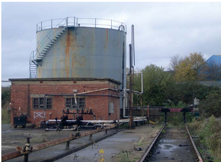
Fig 104 The fuel delivery siding at Old Oak Common in 2011. Almost everything in this picture was installed in 1946
