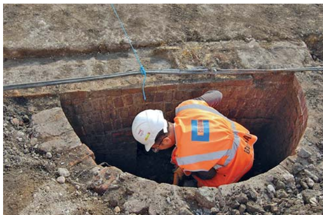
Fig 12 (left) A Marcon Sewer inspection chamber that had once lain inside the BG Shed. The lighter-coloured brick chamber was a post-demolition addition
