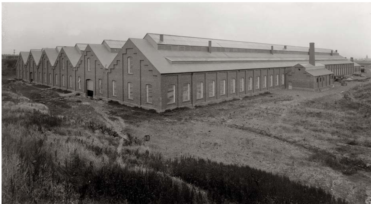
Fig 51 Old Oak Common's mighty four turntable engine shed nearing completion in 1906 (NRM/ Science and Society Picture Library)
