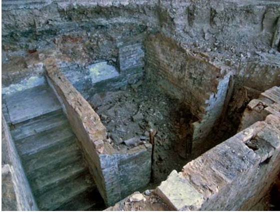
Basement of Alfred Villa, looking south east
