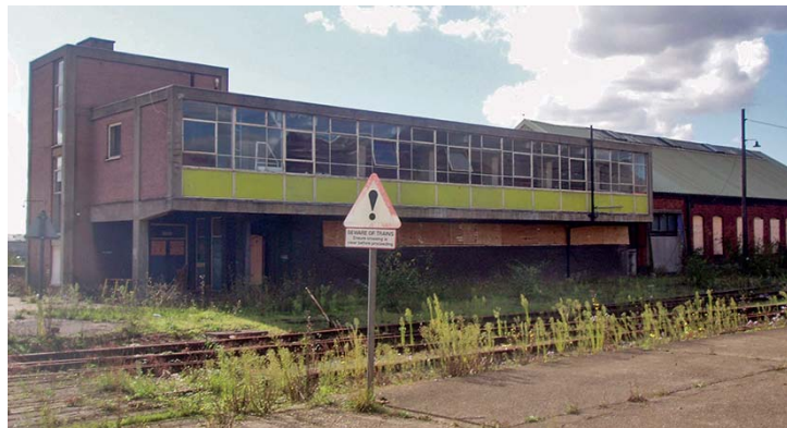
Fig 121 Old Oak Common's new Amenity Building opened in 1963
