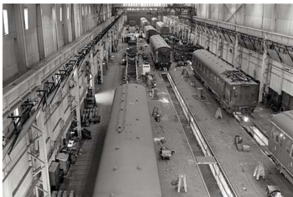
Fig 110 (left) A 1930s design (although not delivered until the late 1940s), the LNER's Shenfield AM6 rolling stock survived in service until the 1980s. Pictured here being overhauled in Ilford Depot's Workshop A in 1969 (NRM/ Science and Society Picture Library NRM 1995-7233_LIVST_RC_251)
