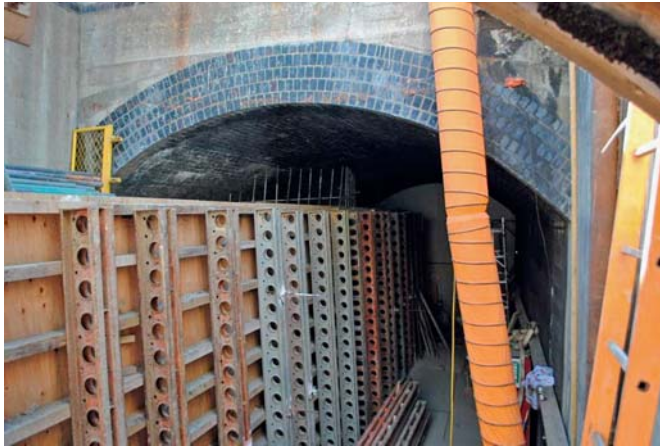
Entrance to shunt tunnel from the west. Crossrail works underway.
