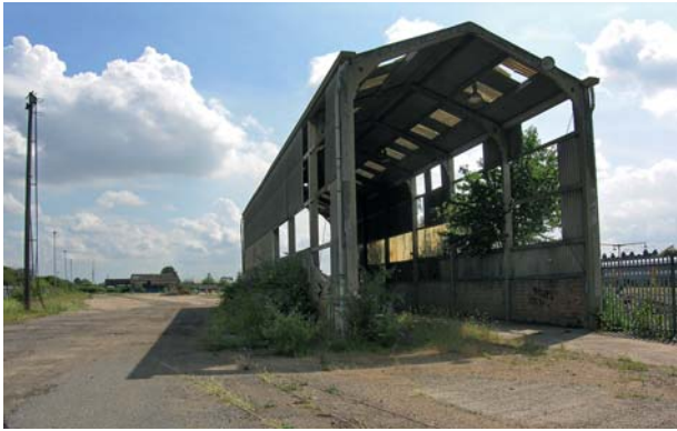
Post-1951 concrete-framed shed in Plumstead station goods yards
