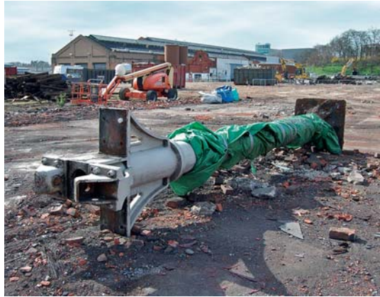
Fig 64 A single cast iron column supported the valley trusses of the Stores building. This was salvaged during demolition and is to be incorporated into the site's new Crossrail depot
