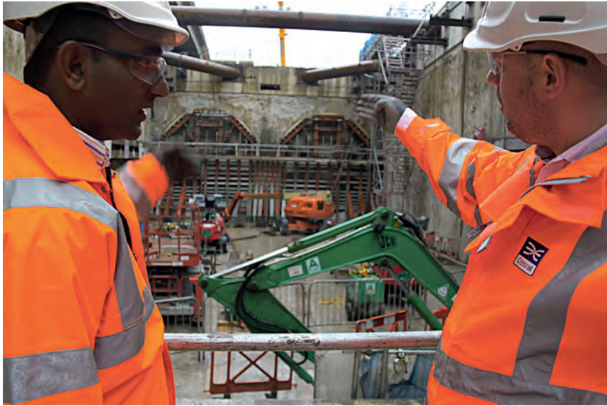
Fig 8 The Crossrail tunnel entrance being formed at Royal Oak Portal
