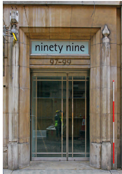
Fig 88 The doorway of No 99 Dean Street shortly before the demolition
