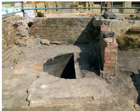
Fig 79 (left) Brick-lined pits in Crosse & Blackwell's 1877 warehouse on Charing Cross Road were part of a structure that supported a static steam engine
