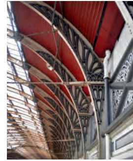
Fig 67 Decorative ironwork of the Paddington train shed (Photograph: © Robin Sones)
