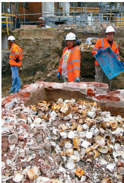
Fig 81 (left) Underground vault uncovered during excavations at Crosse & Blackwell's former warehouse on Charing Cross Road; (right) Part of the vast haul of discarded Crosse & Blackwell containers found in the vault
