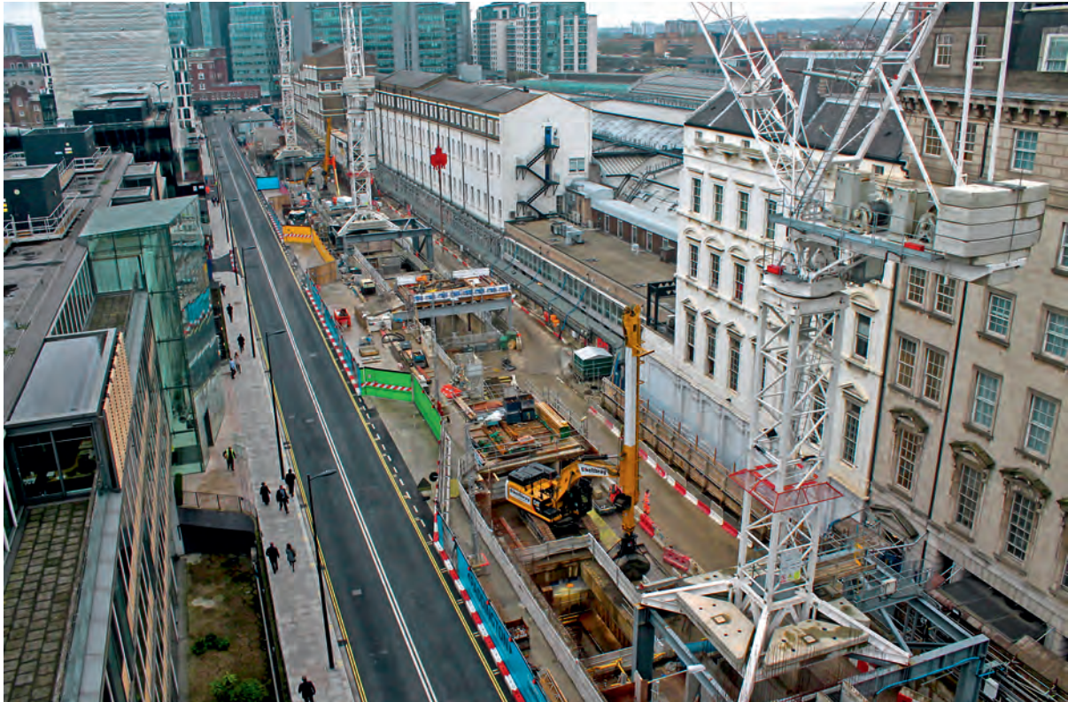
Fig 63 Work underway on the new Crossrail station in Eastbourne Terrace
