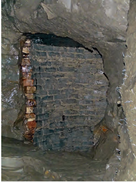
Fig 55 The Soho Square well as revealed in the Crossrail tunnel
