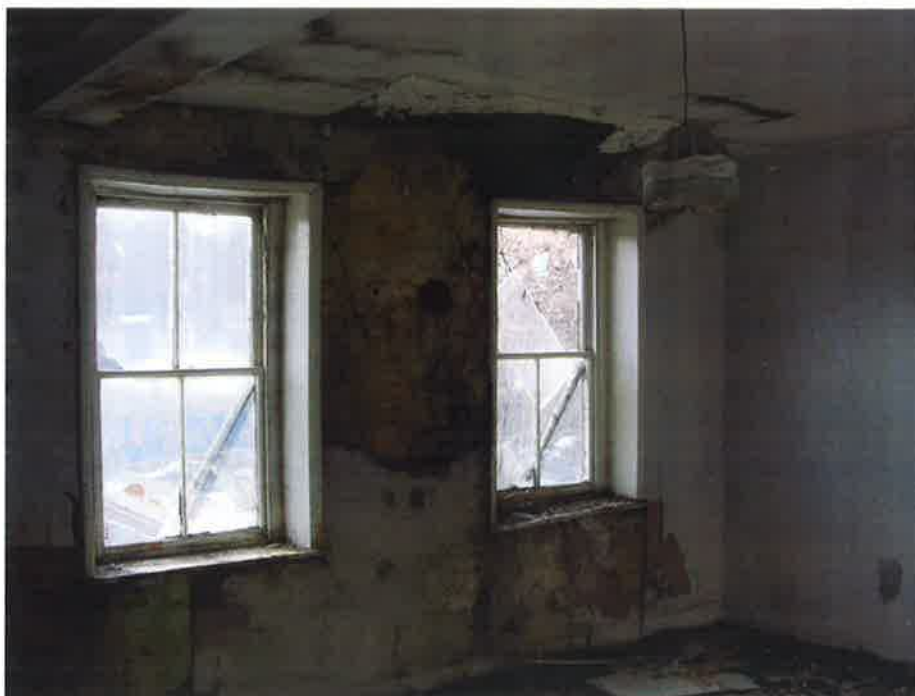
Plate 7: The sash windows on the south elevation of the second floor
