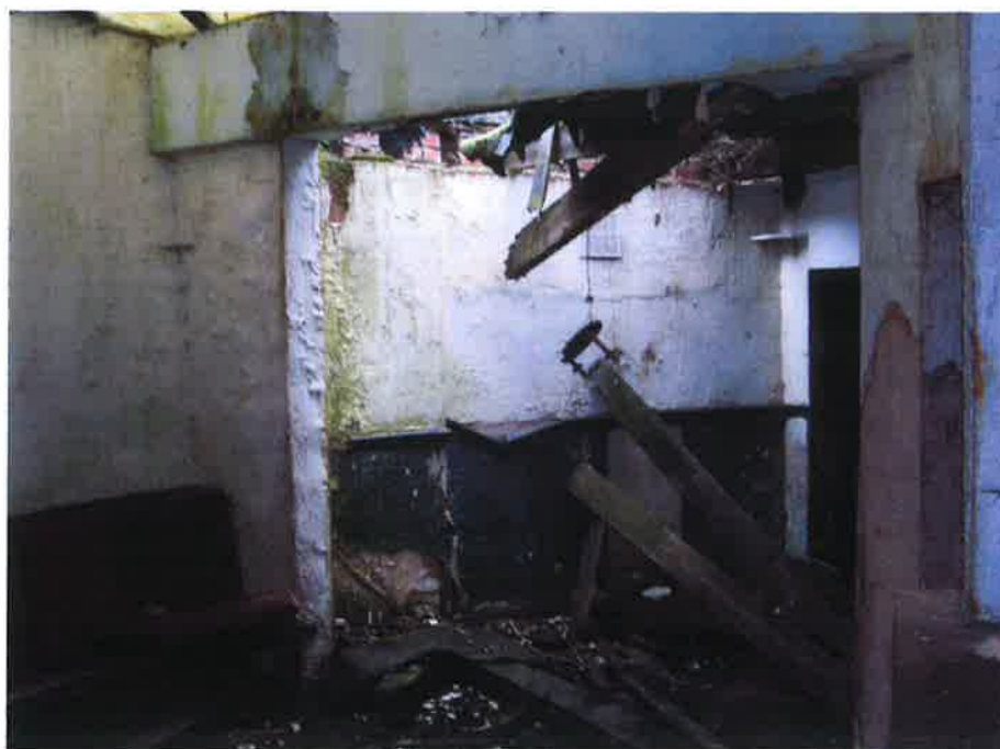
Plate 6: The north extent of the ground floor
