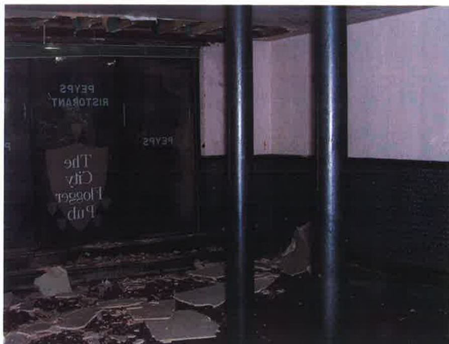
Plate 5: The south and west elevations of the ground floor
