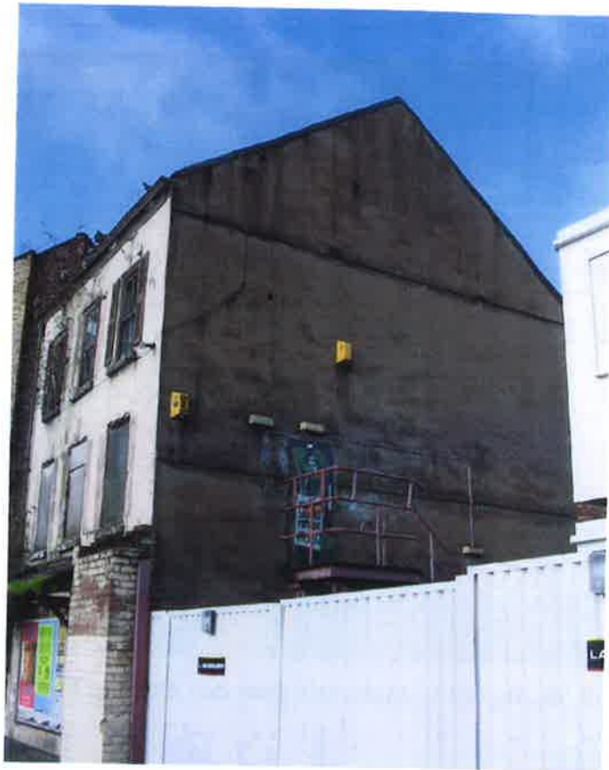
Plate 3: East-facing elevation of 31 Hanover Street
