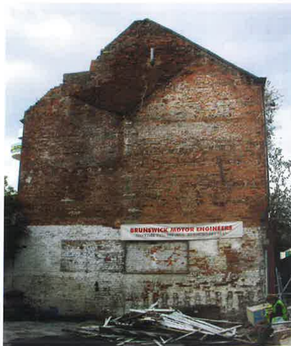
Plate 2: West-facing elevation of 31 Hanover Street
