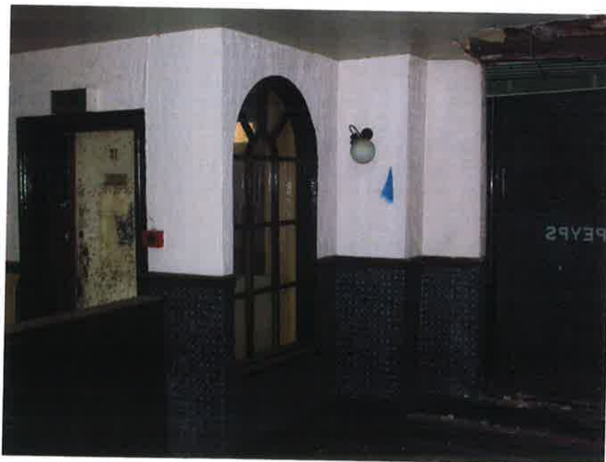
Plate 4: The modern porch and front entrance on the south elevation of the ground floor
