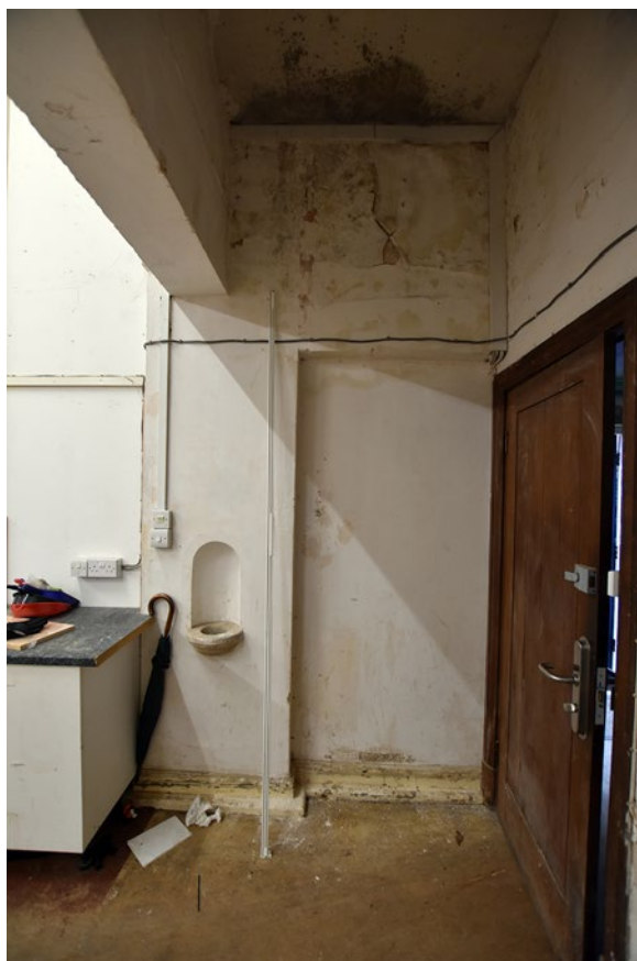
Plate 38: The north wall of the east porch with holy water stoup and blocked doorway
