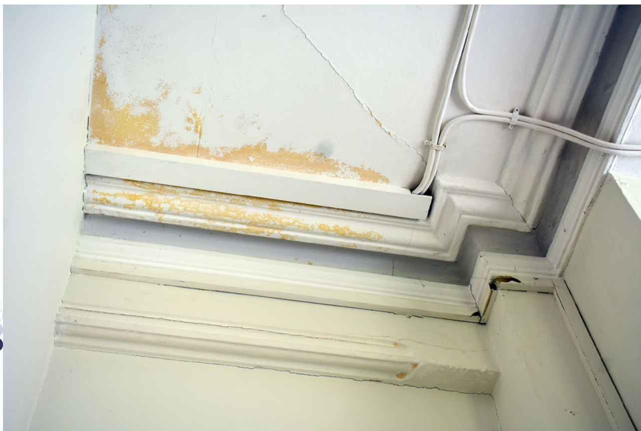
Plate 62: Part of cornice and principal joist from dining room preserved within a bedroom
