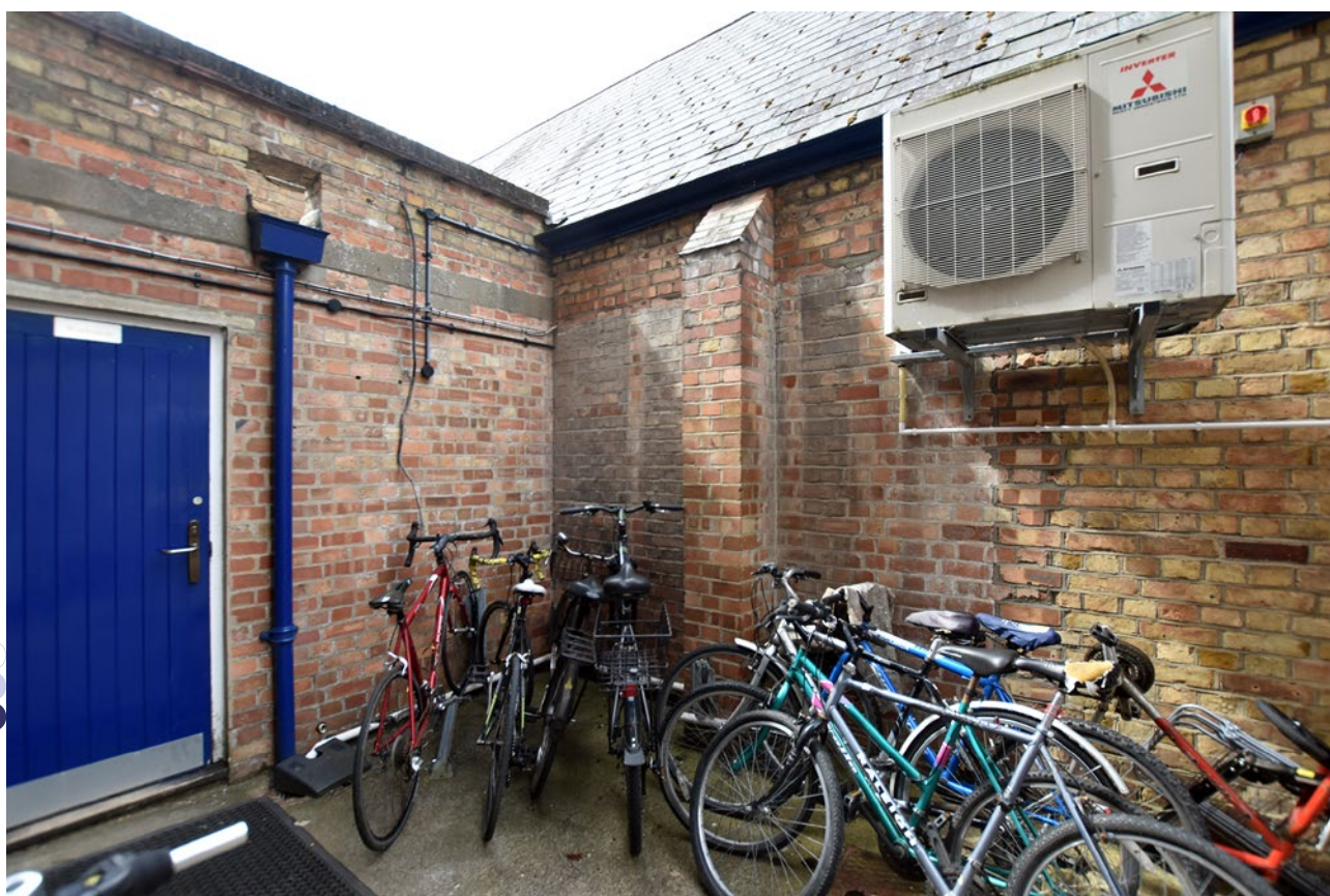
Plate 9: Large area of east elevation rebuilt in red brick
