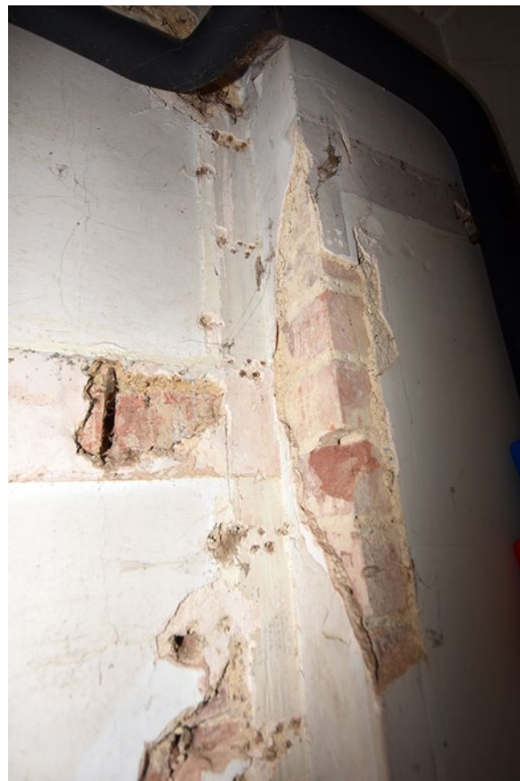
Plate 45: Loss of plaster revealing a red brick buttress
