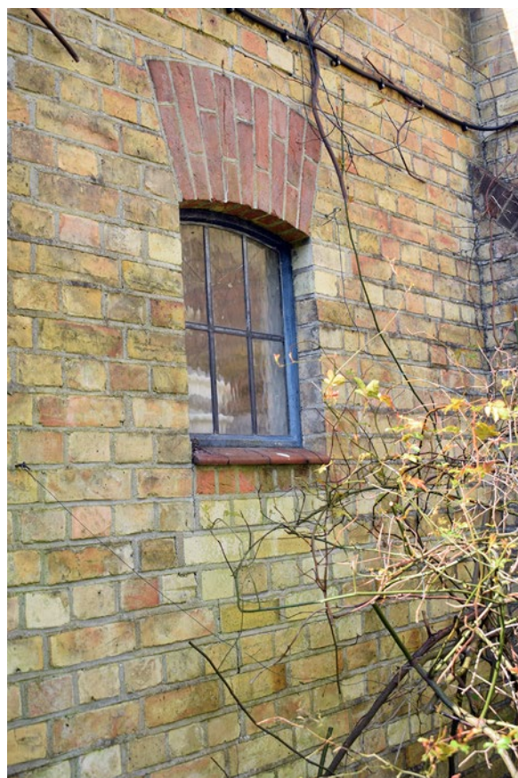
Plate 12: Window fitted within a reduced opening
