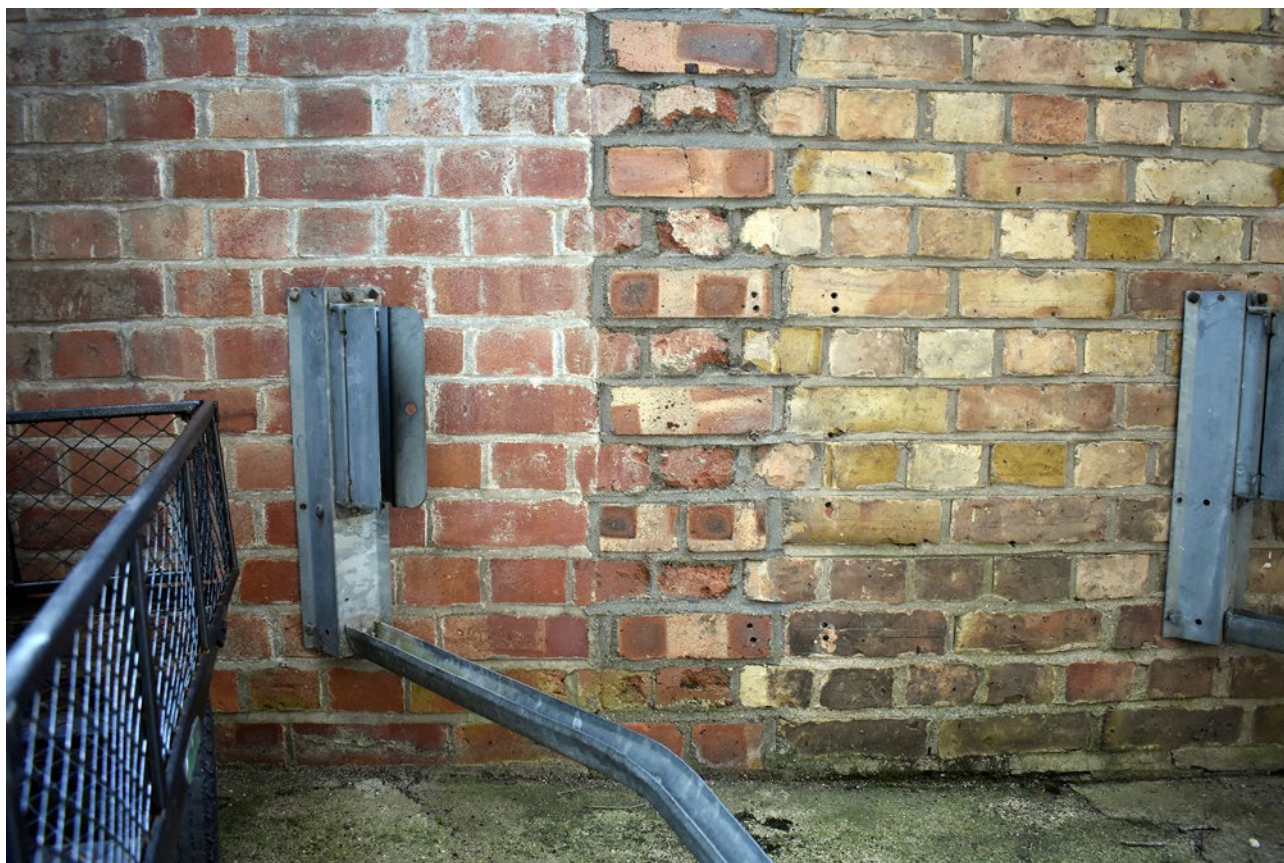
Plate 10: Change from original to secondary red brickwork
