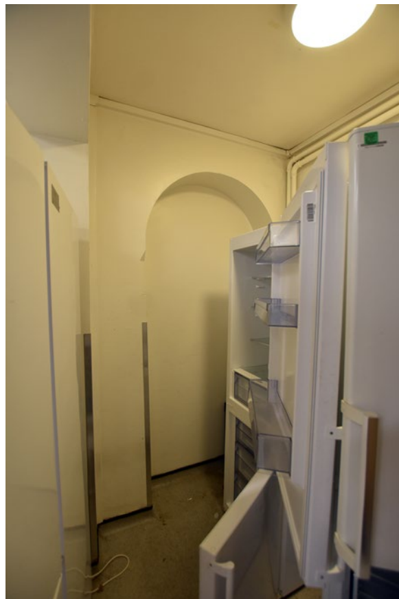
Plate 54: Blocked opening on the west wall of the kitchen
