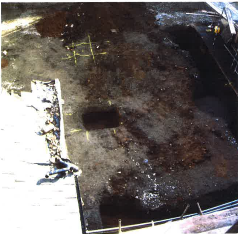
Plate 6: View of open-area groundworks at rear of site
