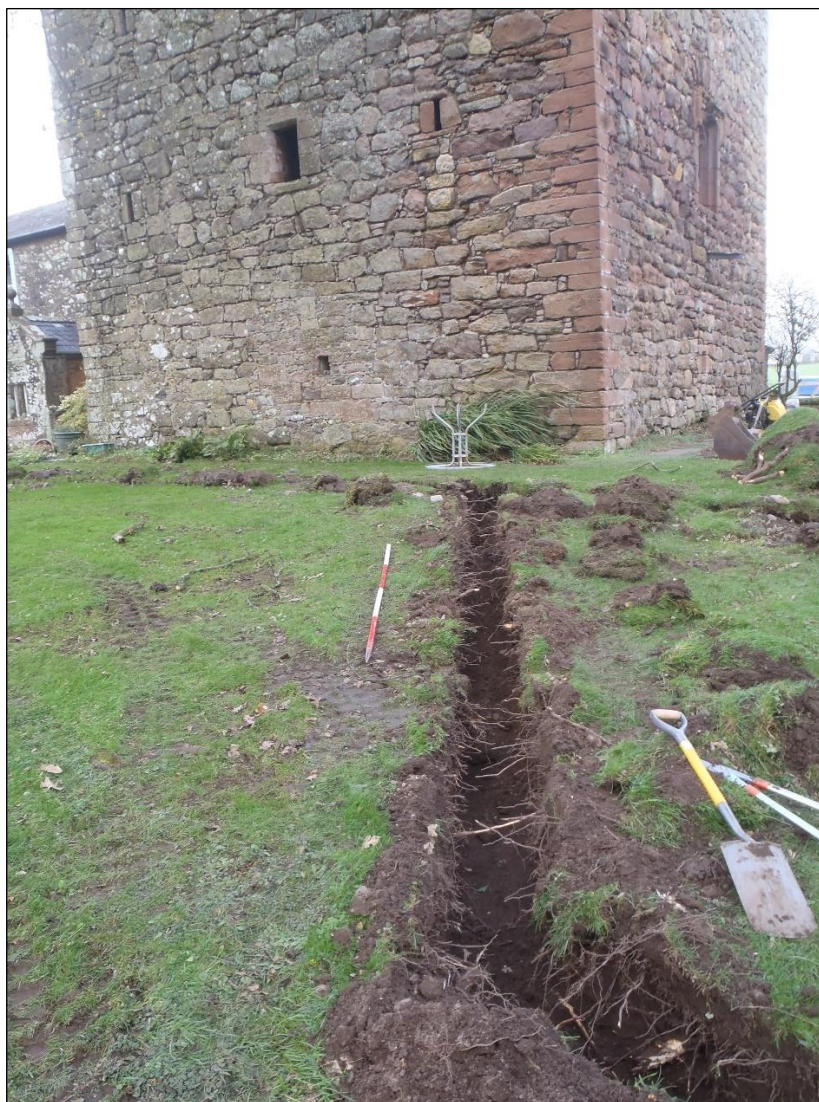
Plate 1: Trench for drain, looking north, 2m scale
