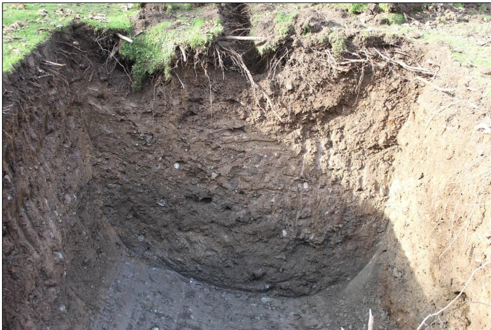
Plate 2: Pit for new septic tank, looking north-west
