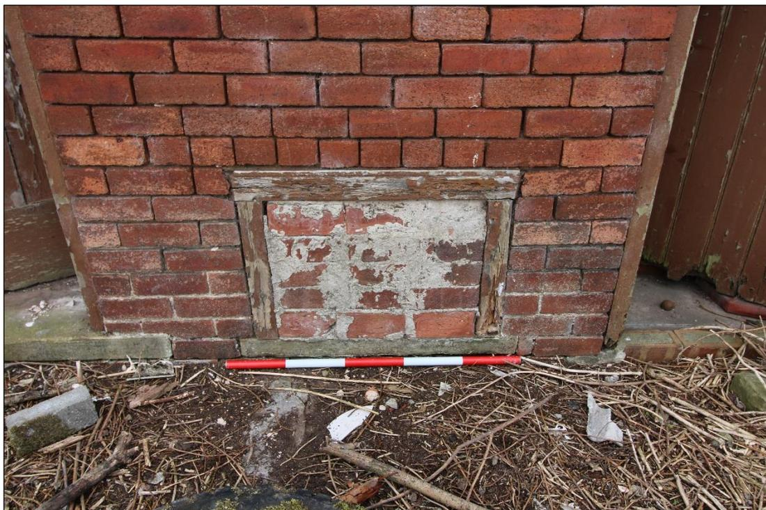
*Plate 31: Blocked aperture at base of wall, with 1m scale*
