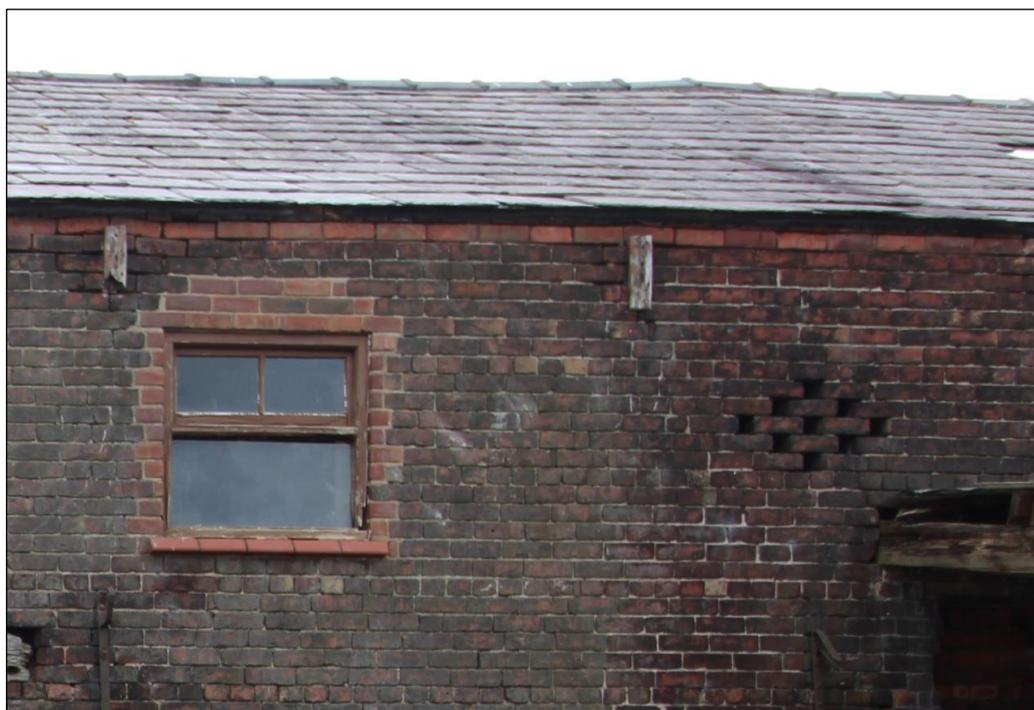
*Plate 24: Inserted first-floor window on western elevation, with ventilation loop to right, facing east*
