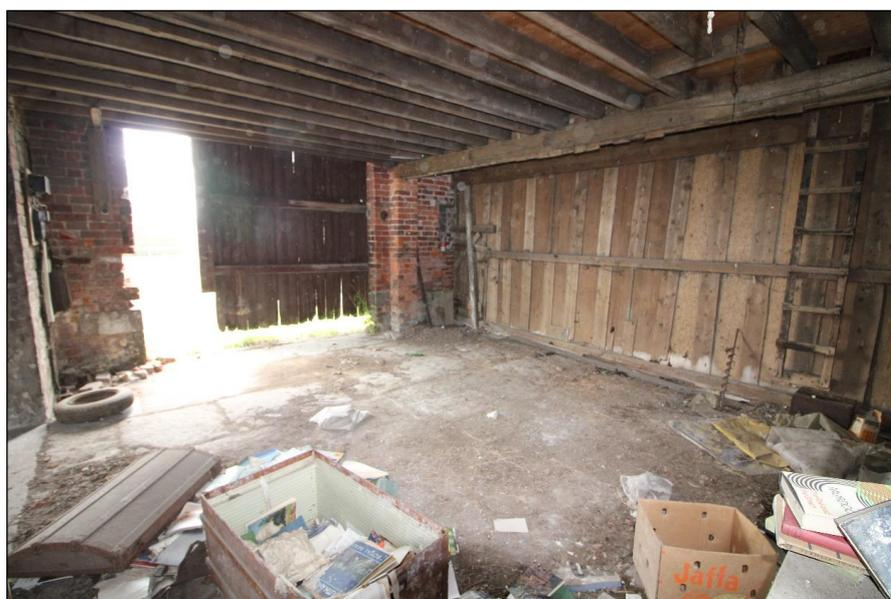
*Plate 39: Interior of northern cell, facing south-east. Note the trimmer in the ceiling to right of frame indicating the position of a former floor hatch*
