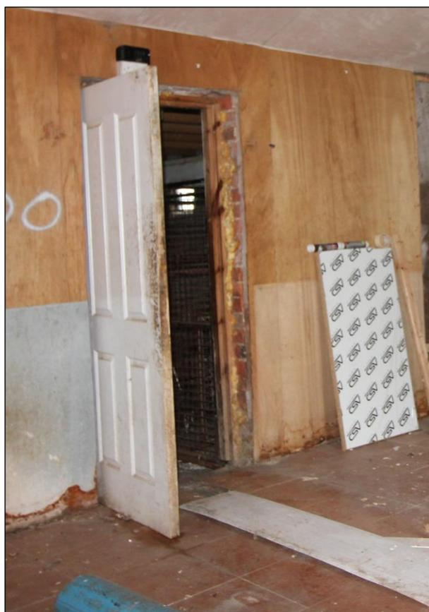
*Plate 63: Western doorway, showing brick jambs in cross-section, facing north-west*
