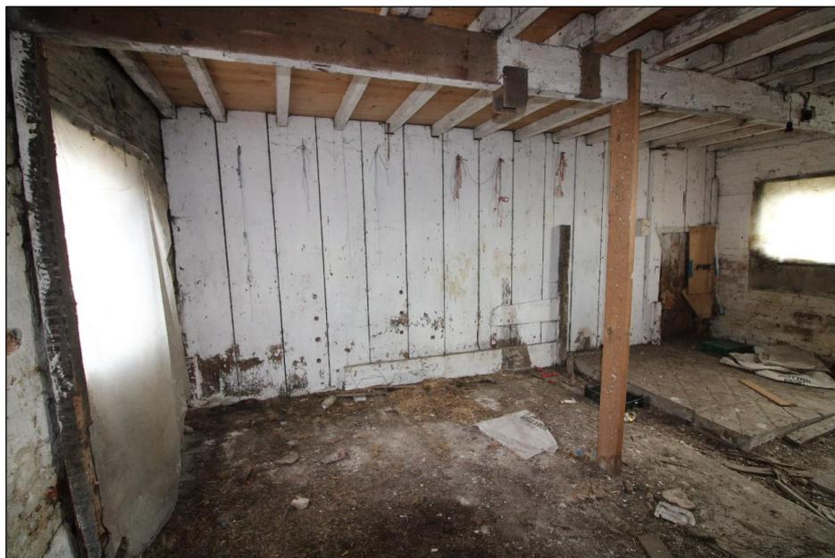
*Plate 36: Northern partition, constructed in vertical timber boards, facing north with low door to right of frame*
