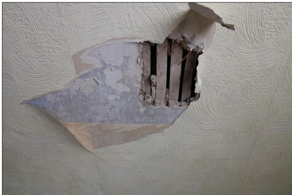
*Plate 51: Lathe and plaster revealed in inspection hole to west of ceiling beam*
