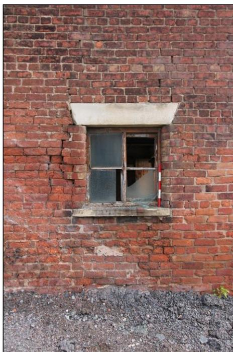
*Plate 18: Horizontal sliding sash window at eastern end of the southern gable*
