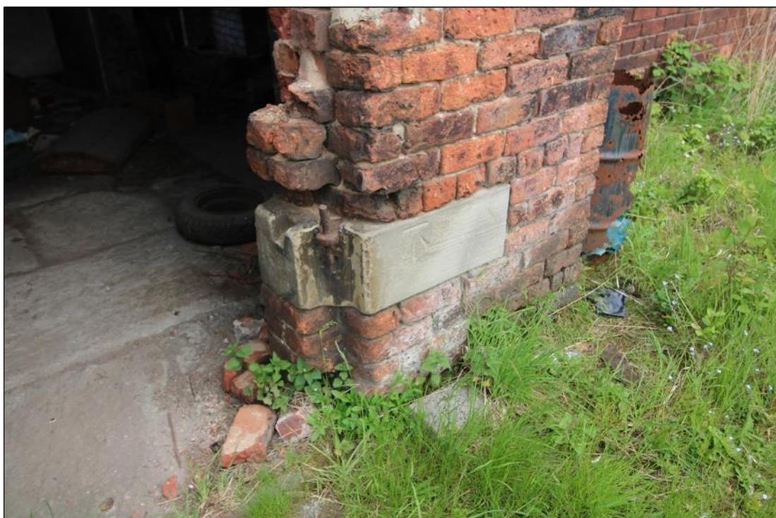
*Plate 12: Pintle hinge, with threshold notch to left and OS bench mark to right, facing west*
