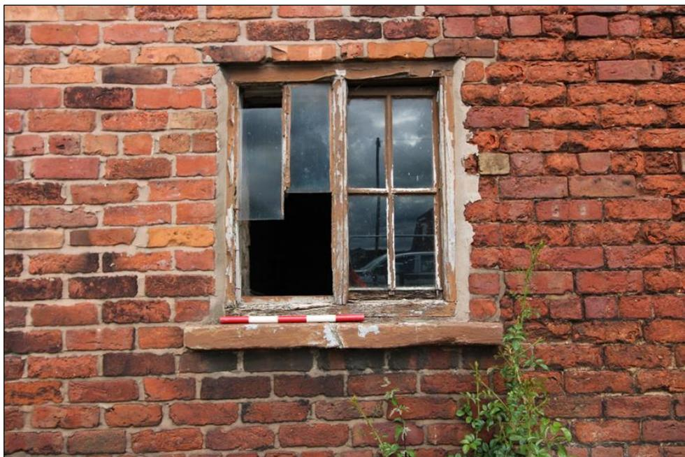
*Plate 15: Sliding sash window at southern end of eastern elevation, facing west with 0.5m scale*
