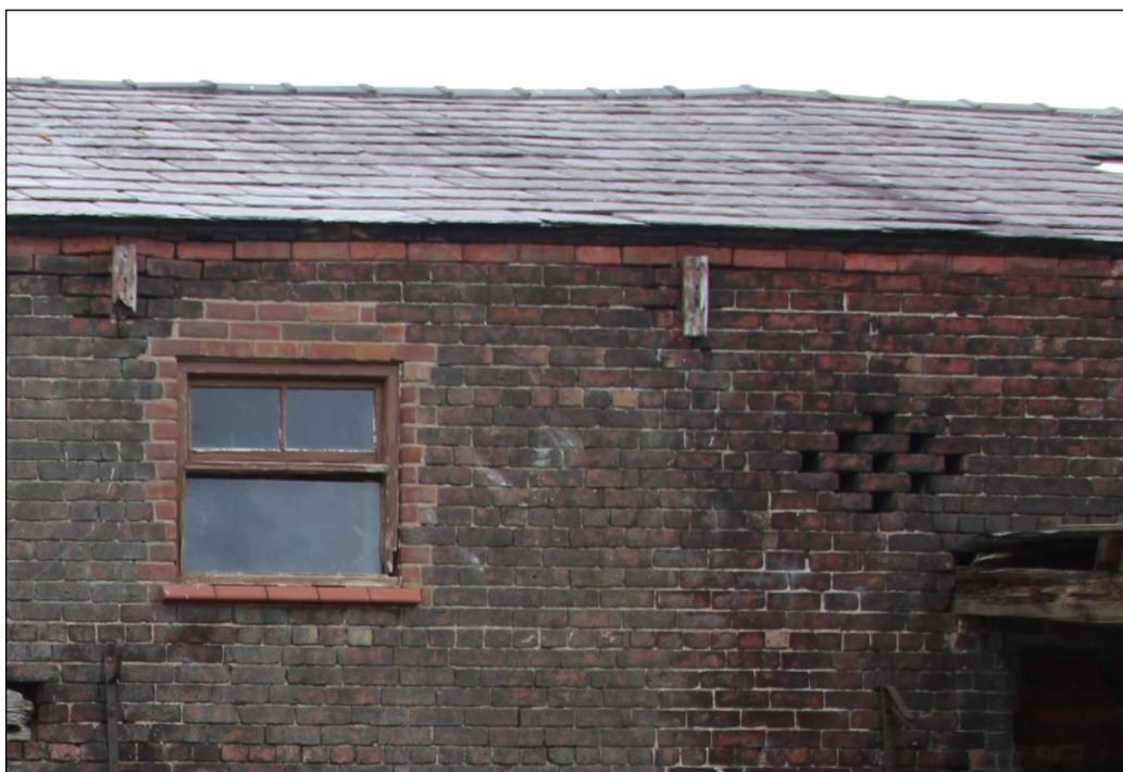
*Plate 24: Inserted first-floor window on western elevation, with ventilation loop to right, facing east*
