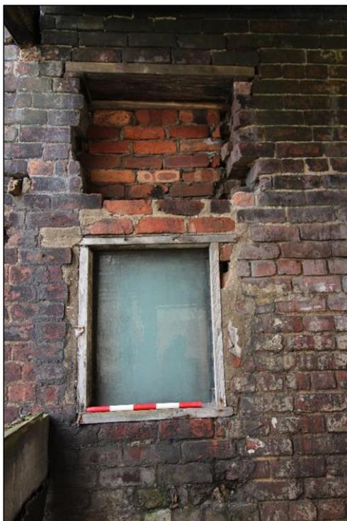
*Plate 23: Crudely inserted window towards southern end of western elevation, facing east with 0.5m scale*
