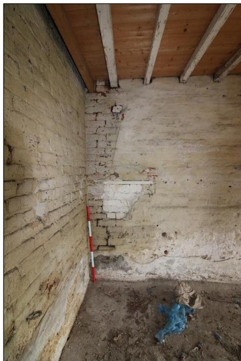
*Plate 34: Diagonal scar on the northern wall denoting former position of Hayrack, facing north with 1m scale*
