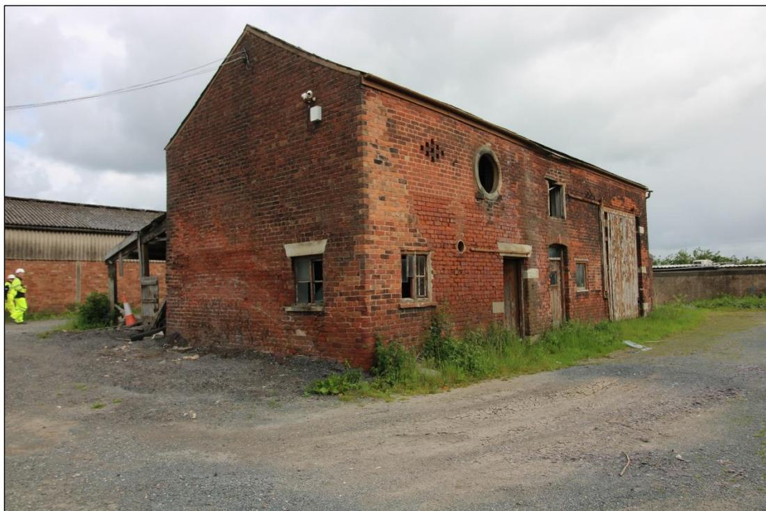
*Plate 8: Exterior of Barn, facing north-west, note rebuilding of south-eastern corner*
