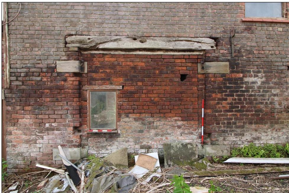
*Plate 21: Blocked double width entrance on western elevation, facing east with 1m scale*
