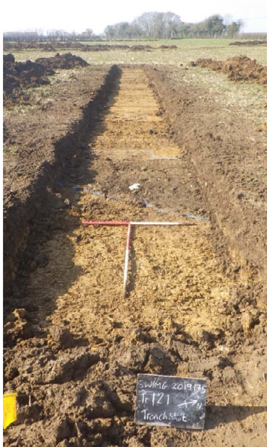
Plate 7: Trench 121 looking northwest (2x 1m scale)
