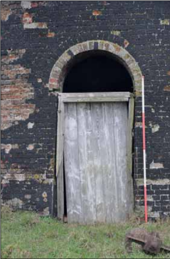
Plate 19: South-east side door, from the south-east
