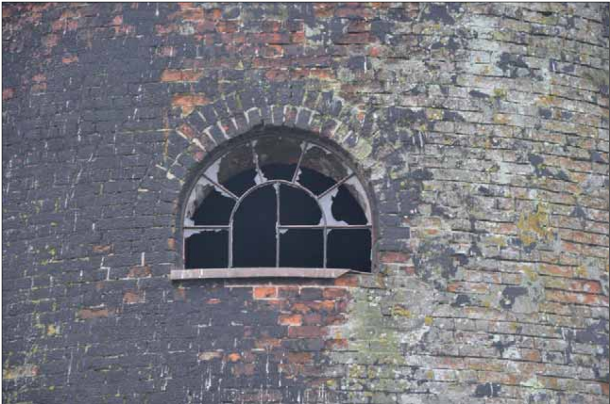
Plate 21: South-west side window to the second floor, from the south-west
