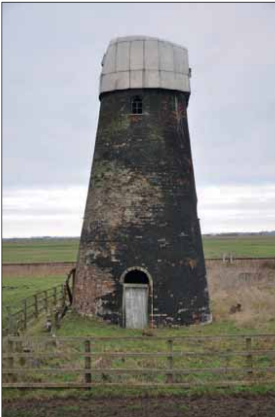
Plate 18: Lockgate Mill, from the south-east
