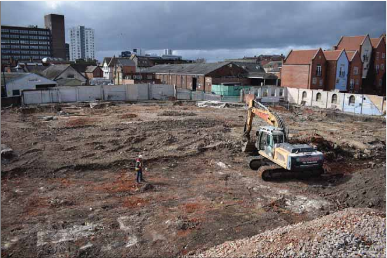
Plate 1: North-western extent of the development site, looking north-west
