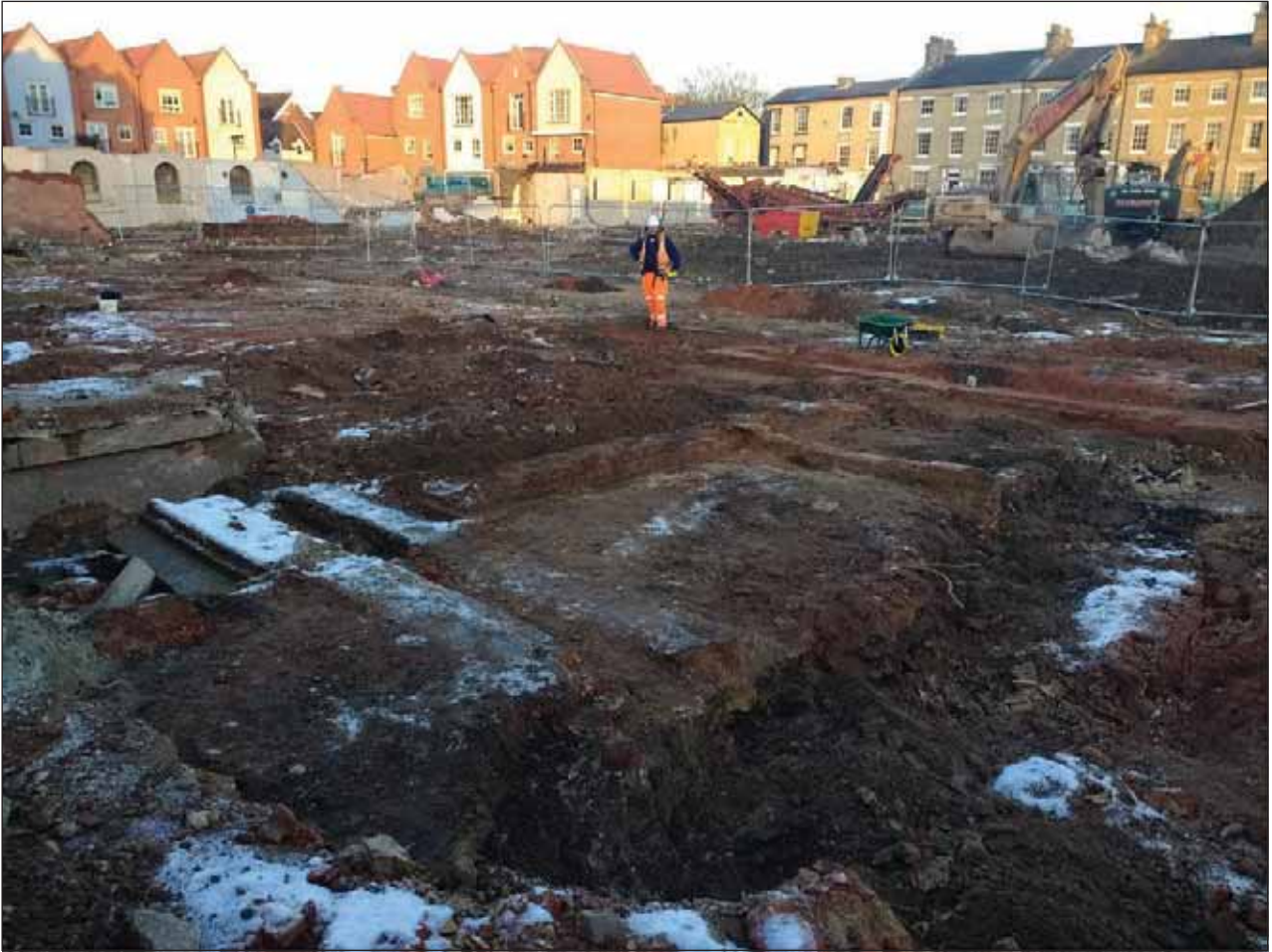
Plate 17: Area 10: Period 4.2 walls 1245=1261, etc, looking north-east
