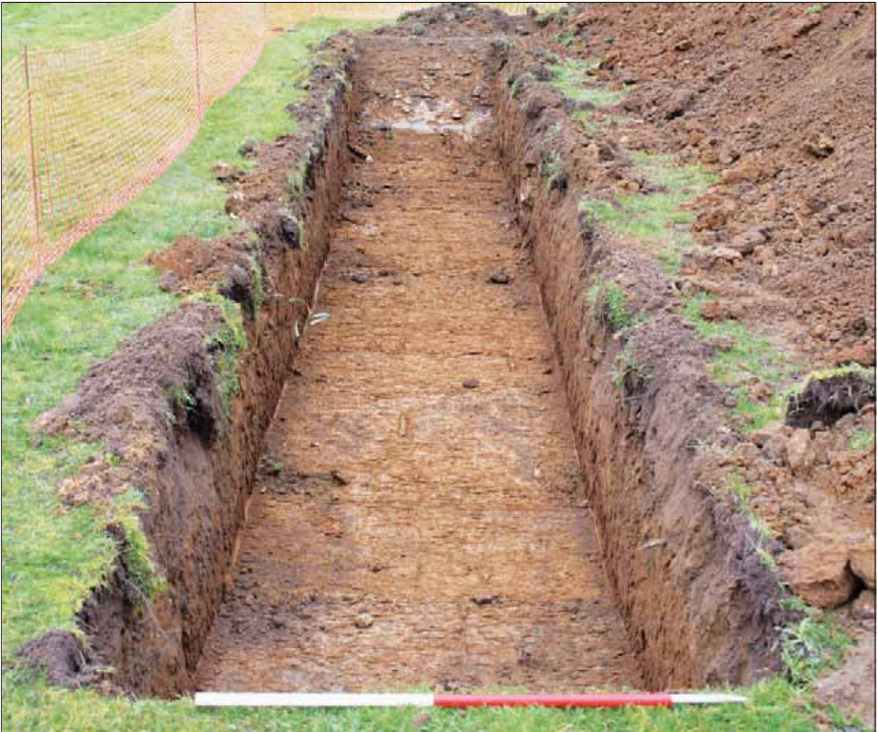
Plate 1: Trench 2, looking north-west
