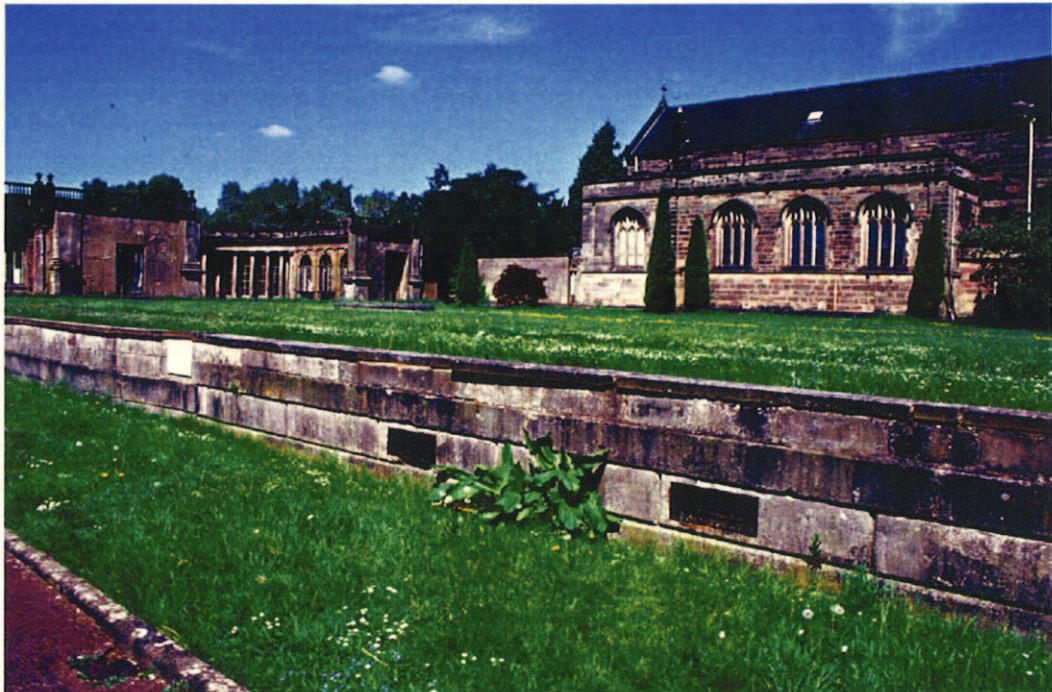
Plate 14: Vents in retaining wall at southern limit of the ground floor/basement
