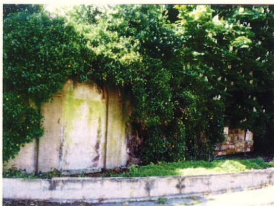
Plate 9: Arch in eastern retaining wall
