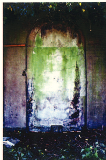
Plate 10: Close up of arch showing
