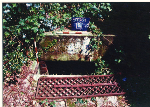
Plate 1: Access to Site A; possible light well / shute
