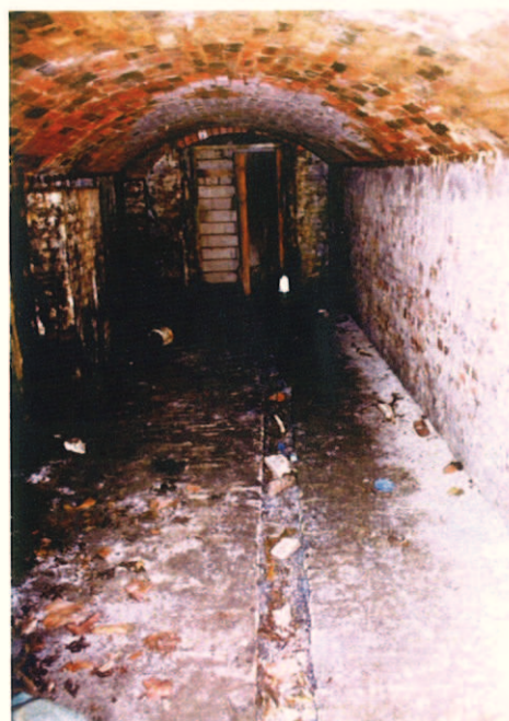
Plate 2: Northern limit of main passage, with blocked doorway
