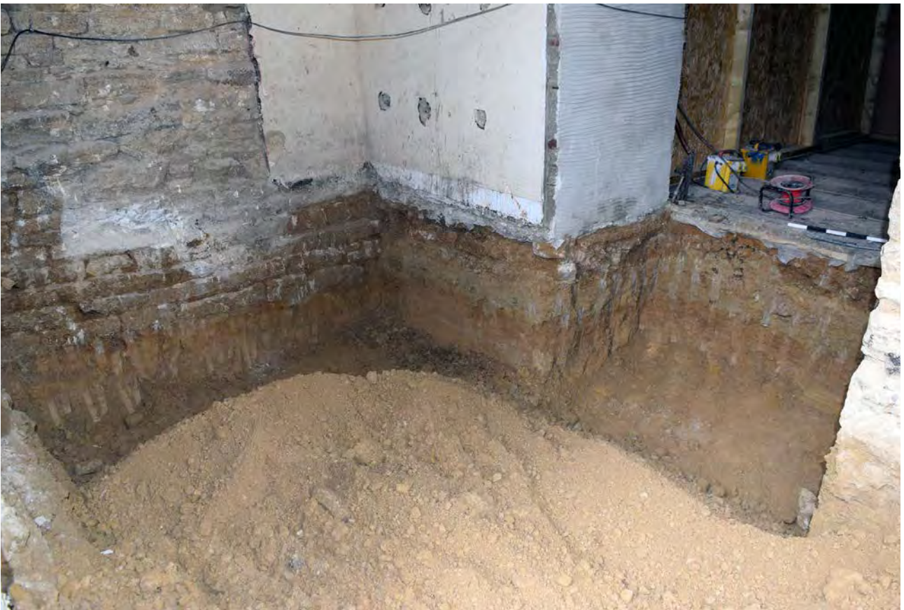
Plate 8: General view, sections 2, 3 4 and 5
