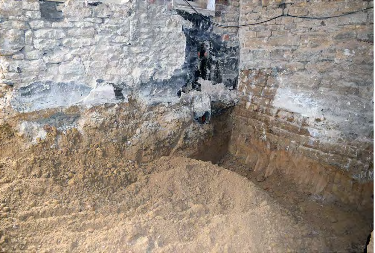
Plate 7: General view, sections 1 and 2
