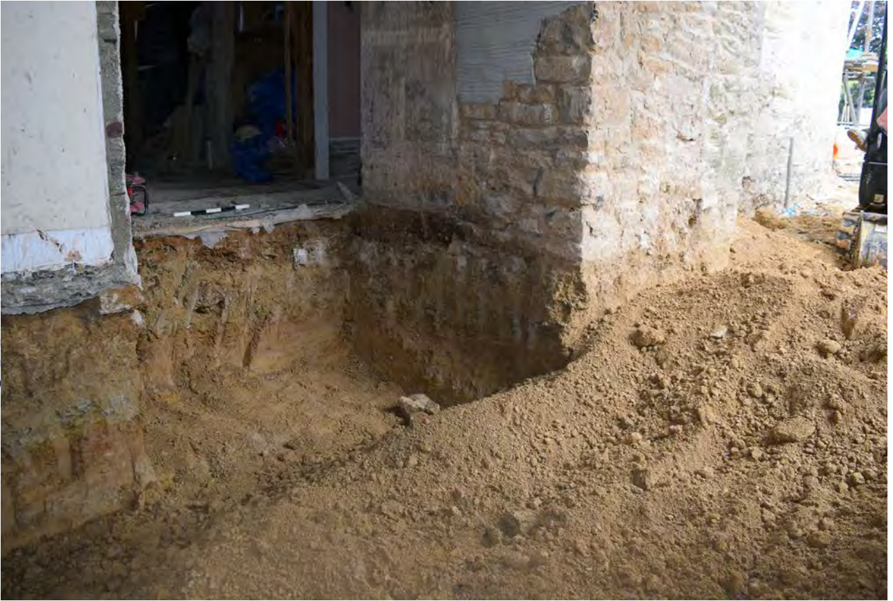
Plate 9: General view, sections 3, 5 and 6
