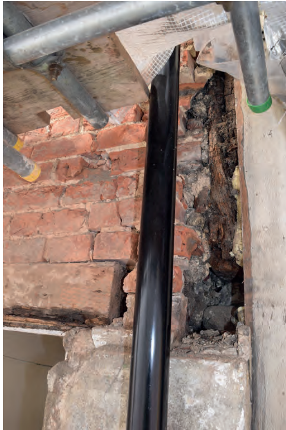
Plate 49: Remains of northern corner post of Nos. 5-6
