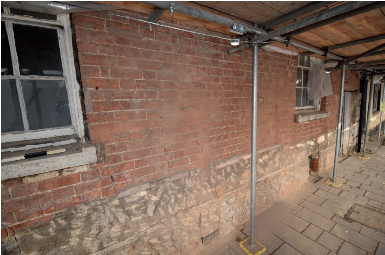
Plate 48: Ground floor of Nos. 5-6
