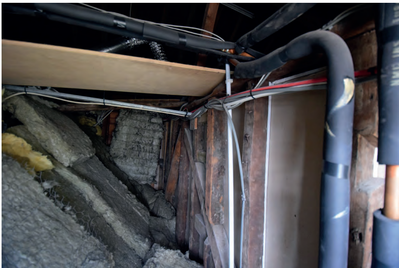
Plate 32: Wall of No. 3 overlying the roof structure of Nos. 1-2
