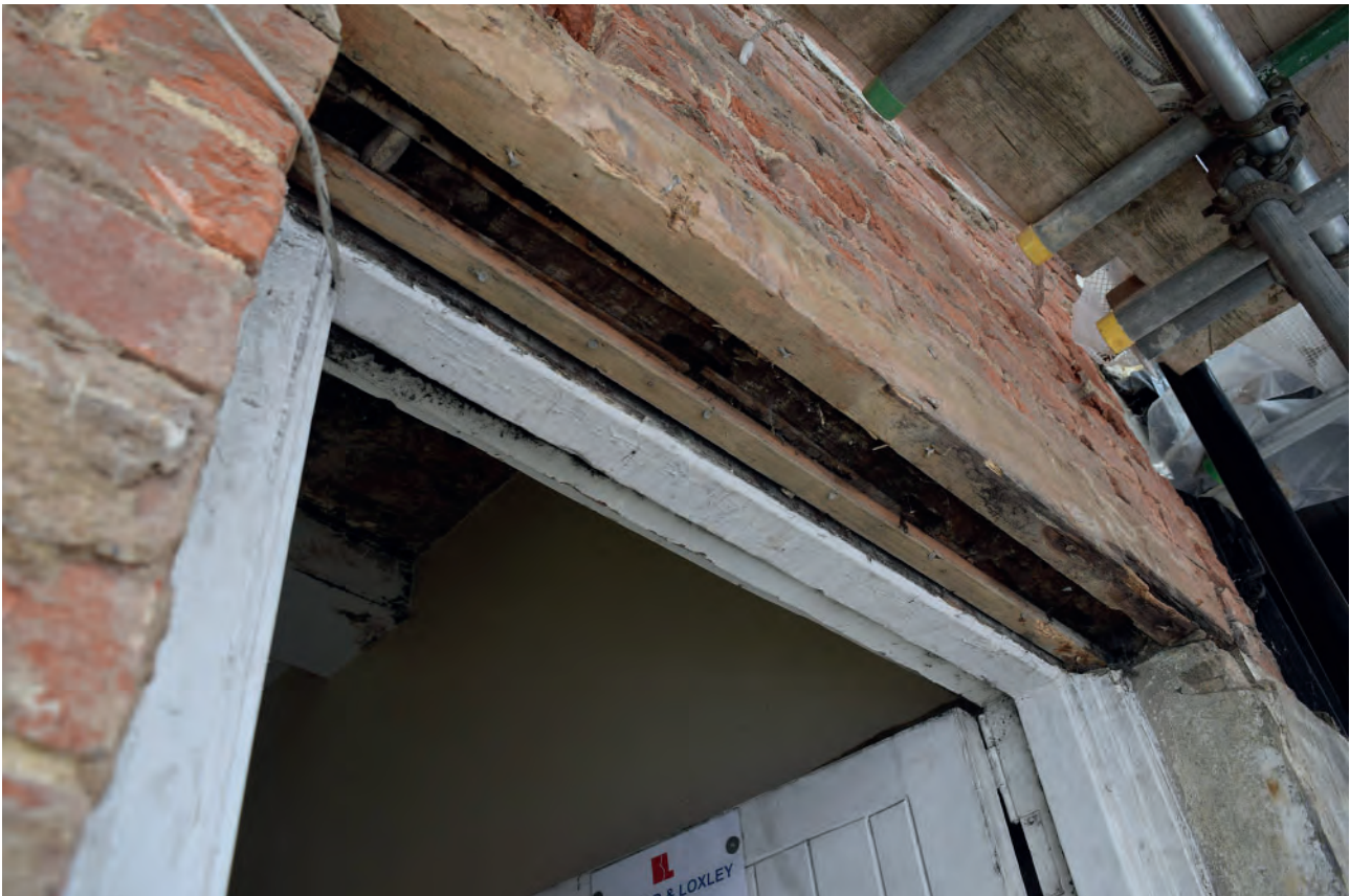
Plate 50: Original passage lintel between newer timbers on Nos. 5-6
