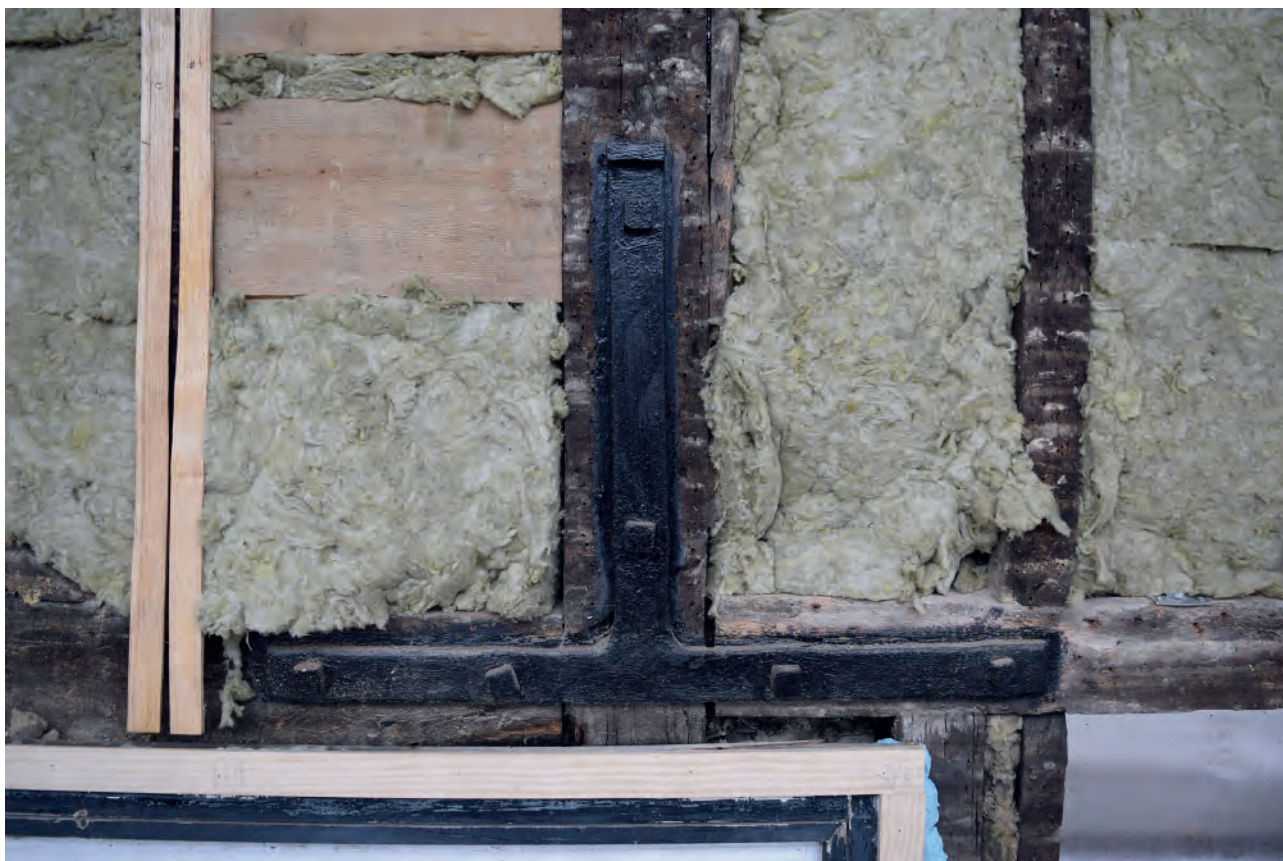
Plate 11: Strap above the northern first floor window of Nos. 1-2
