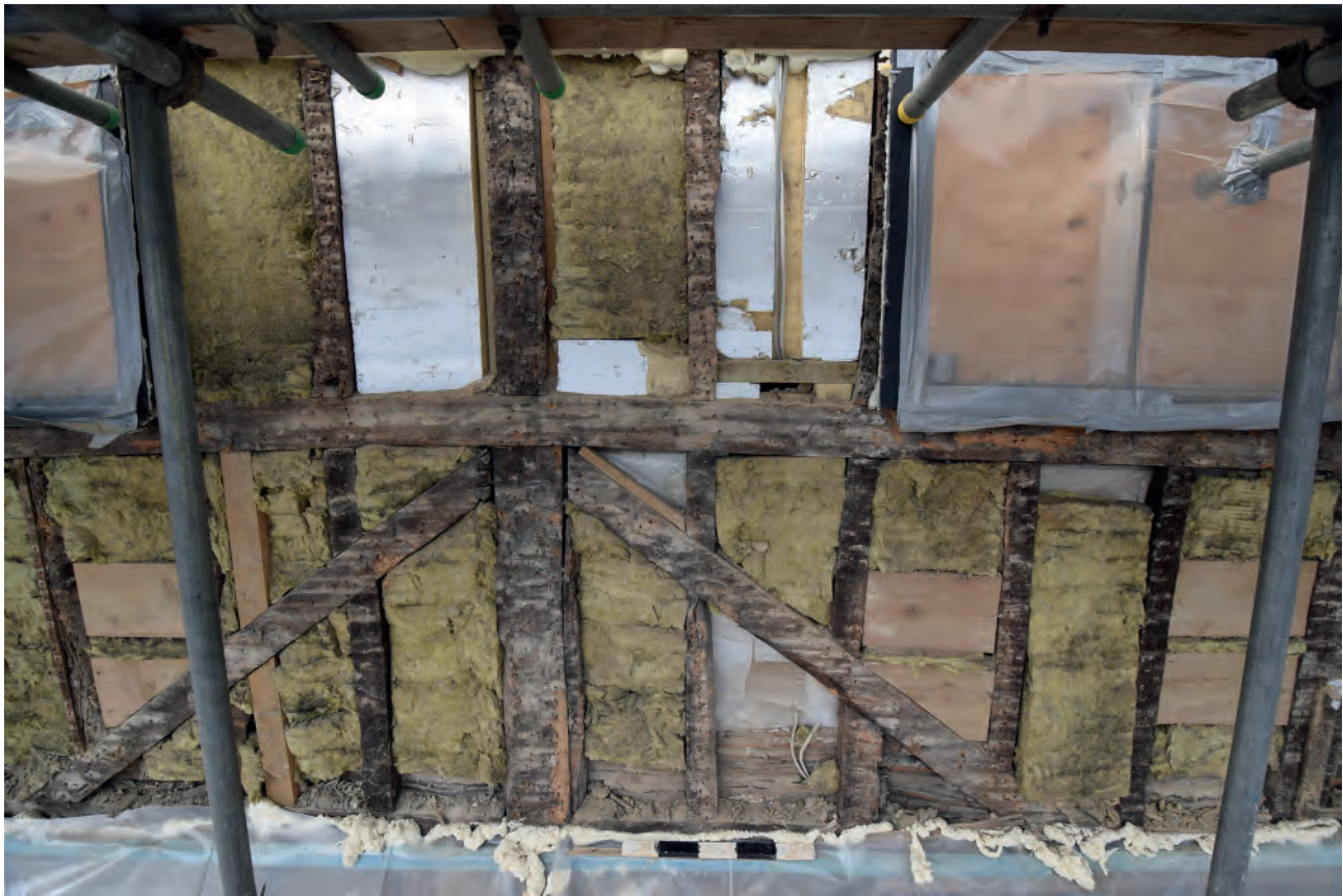
Plate 9: Braces on the east elevation of Nos. 1-2 at second floor level
