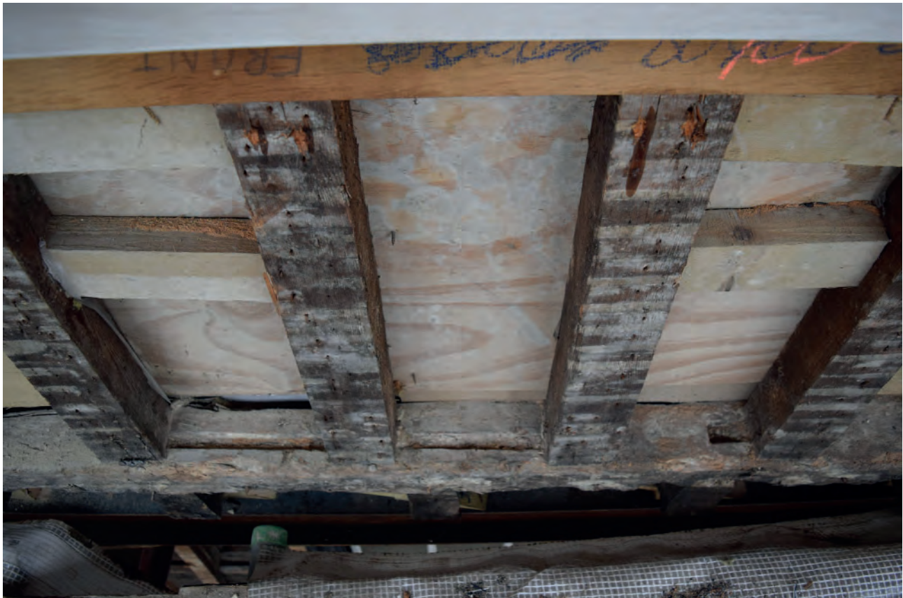
Plate 2: Studs fixed into a groove at first floor level of Nos. 1-2
