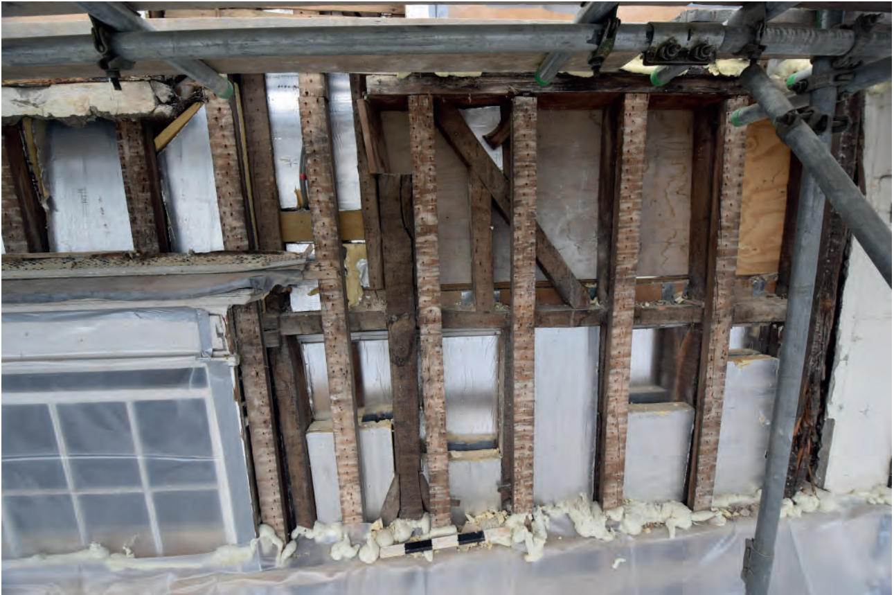
Plate 45: Refacing on the first floor of Nos. 5-6
