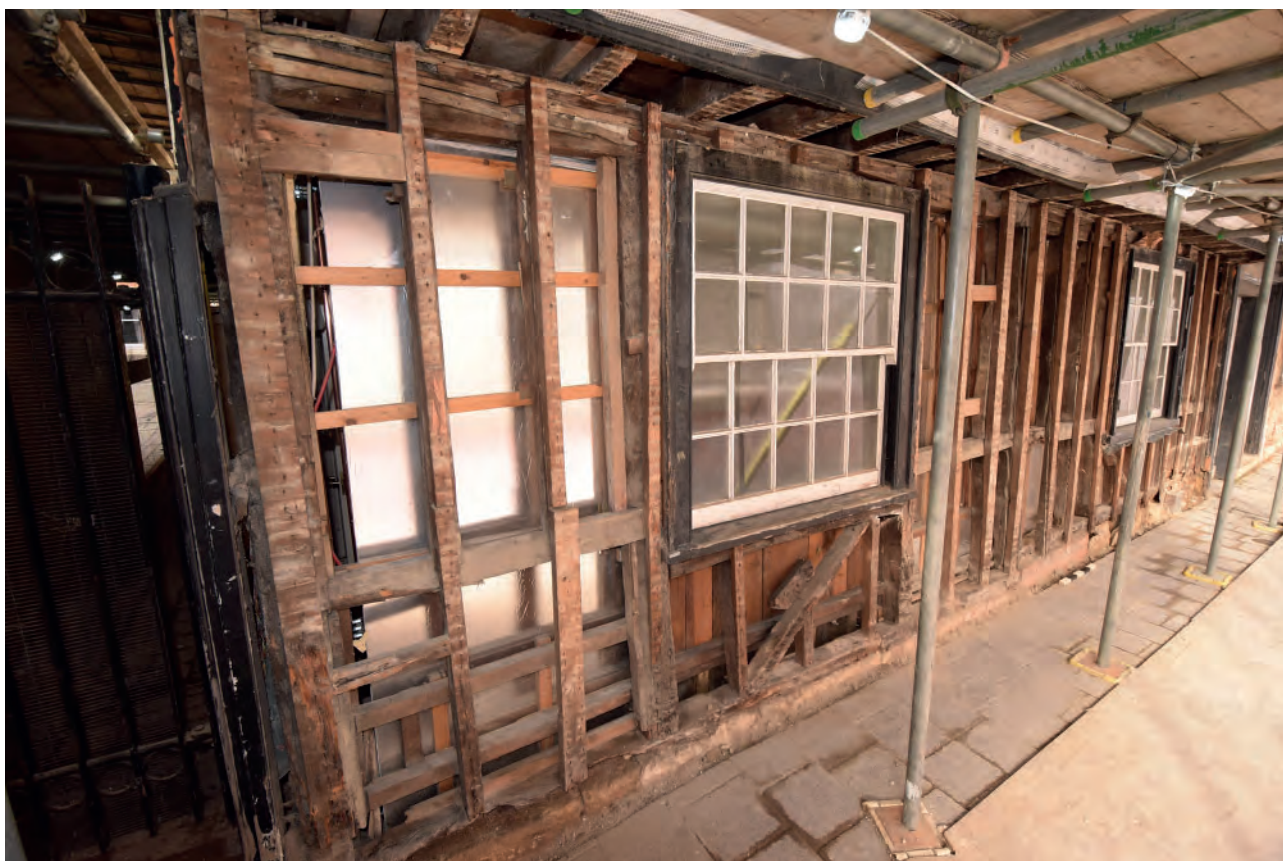
Plate 12: The refaced ground floor of Nos. 1-2
