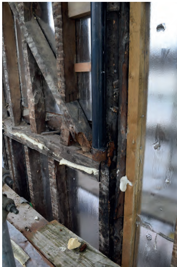
Plate 28: Change from No. 3 to Nos. 4-6 with laths in between
