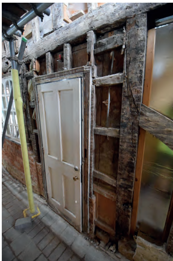
Plate 17: Entrance to Nos. 1-2 on the south elevation
