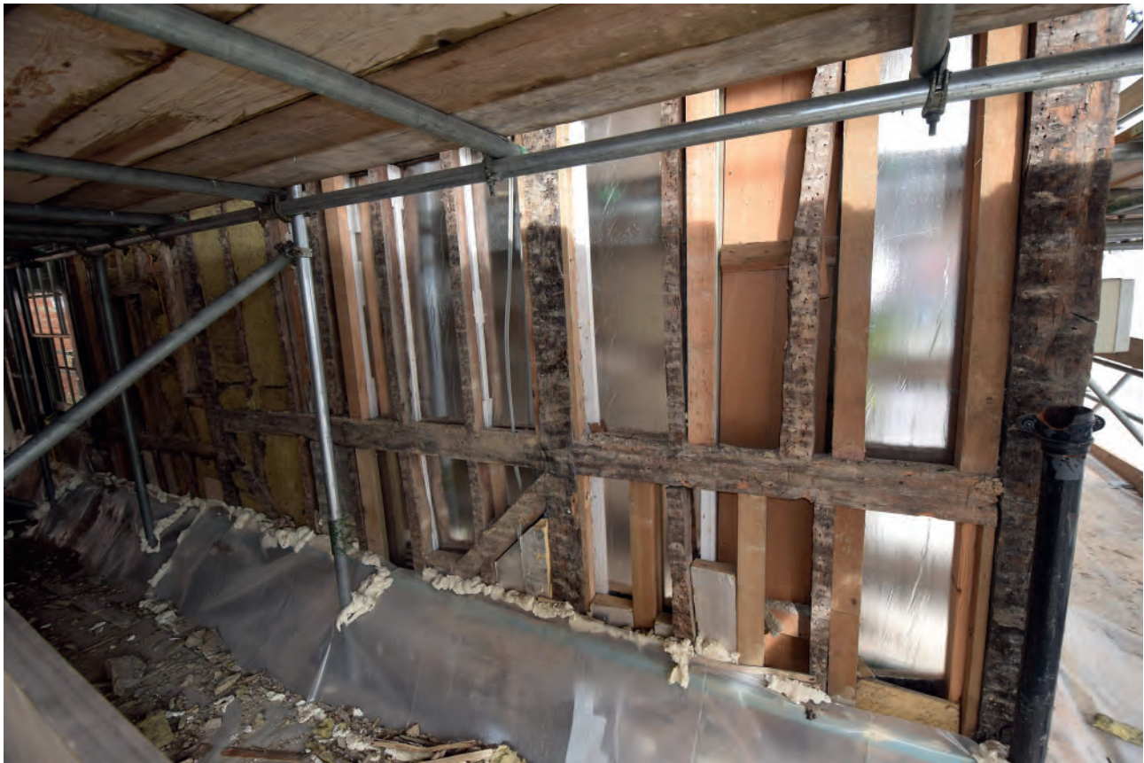
Plate 19: East elevation of Nos. 1-2 at first floor level
