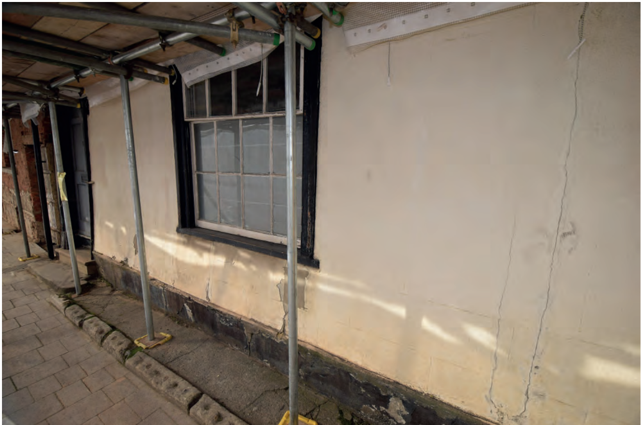
Plate 60: Stone settings for lost rails of No. 7
