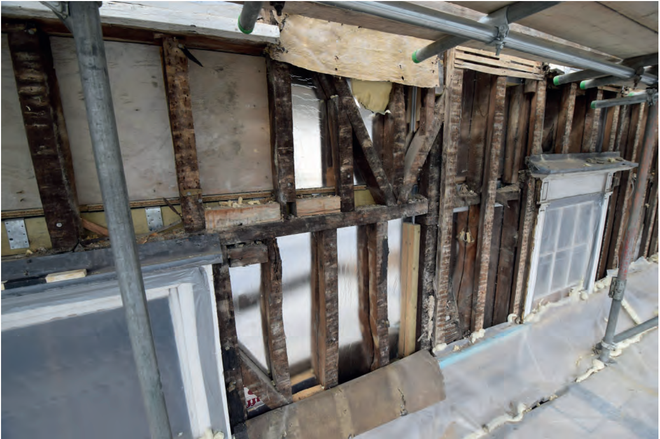
Plate 35: Primary framing of No. 4 and refacing of Nos. 5-6
