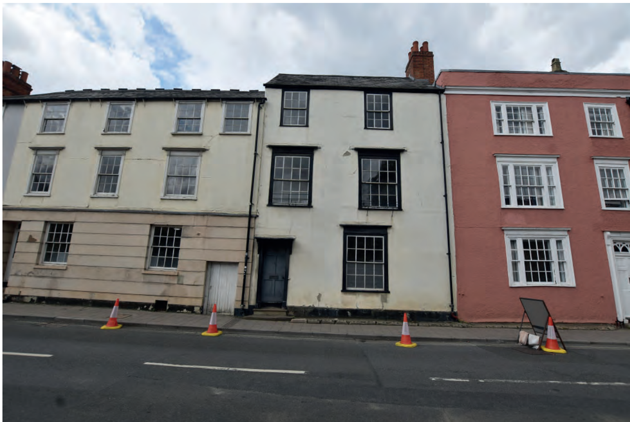
Plate 53: East elevation of No. 7 Longwall Street before work commencing
