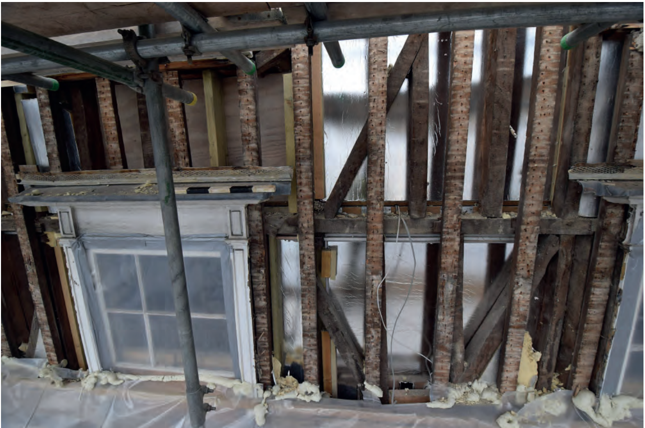
Plate 46: Refacing on the second floor of Nos. 5-6
