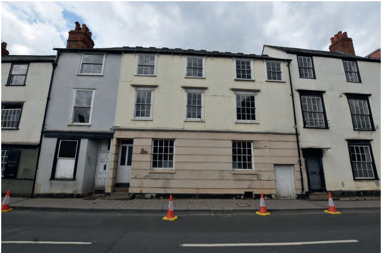
Plate 34: East elevation of Nos. 4-6 Longwall Street before work commencing
