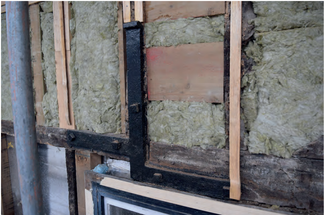
Plate 10: Strap above the southern first floor window of Nos. 1-2
