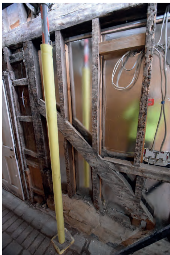
Plate 21: Brace on east elevation of Nos. 1-2
