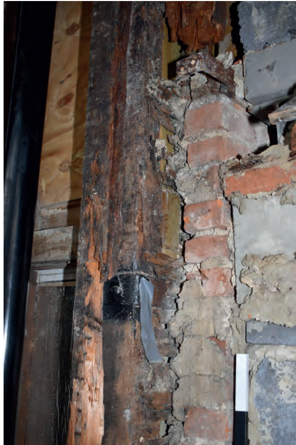
Plate 39: Iron brace and laths between Nos. 5-6 and No. 7
