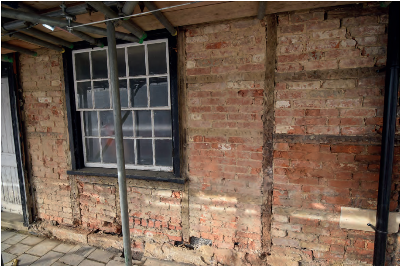
Plate 33: Brick reface on the ground floor of No. 3
