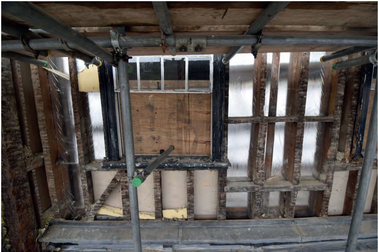
Plate 29: Southern half of the first floor of No. 3
