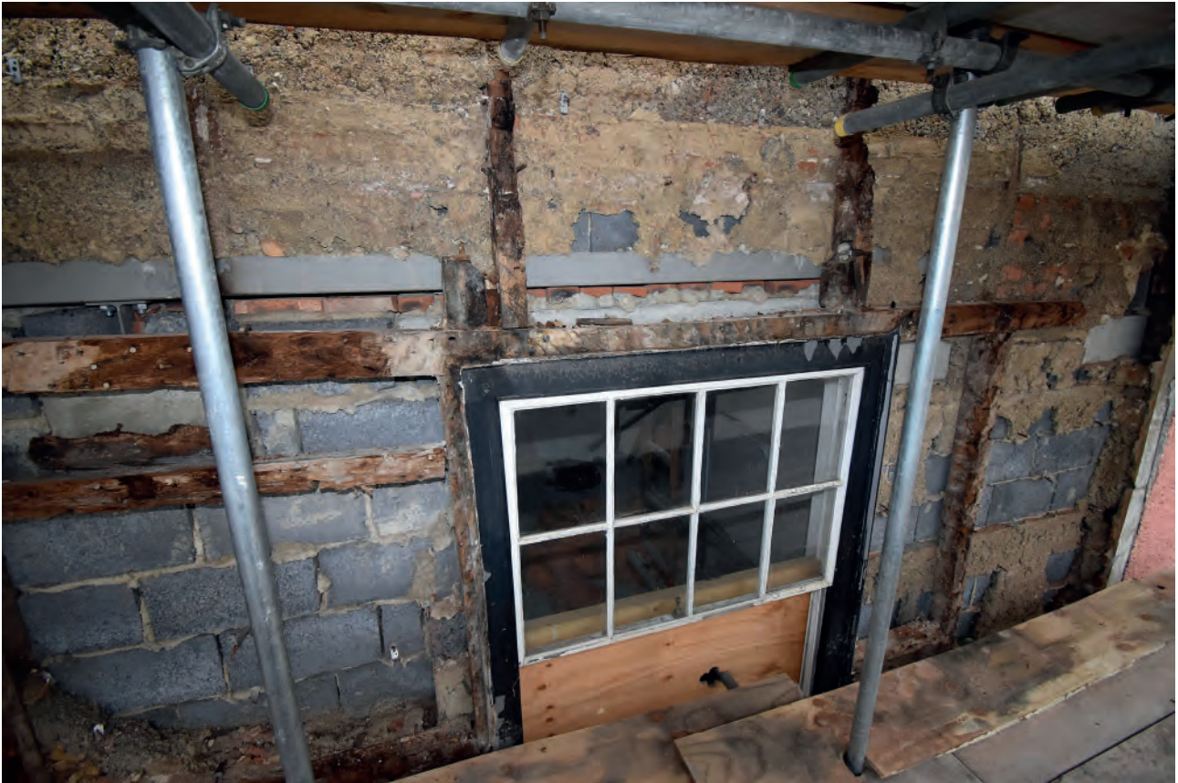
Plate 55: First floor of No. 7
