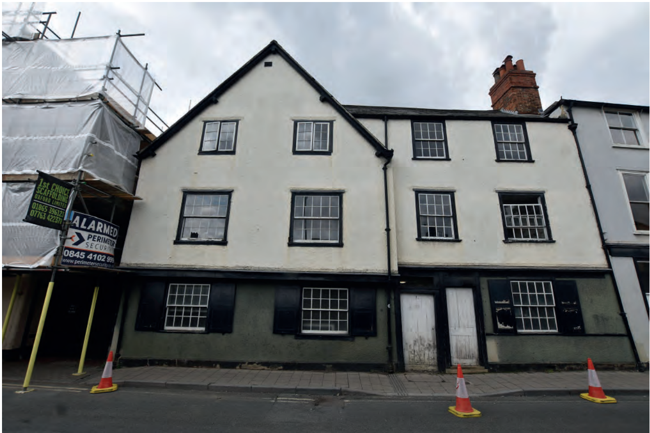
Plate 1: East elevation of Nos. 1-3 Longwall Street before work commencing
