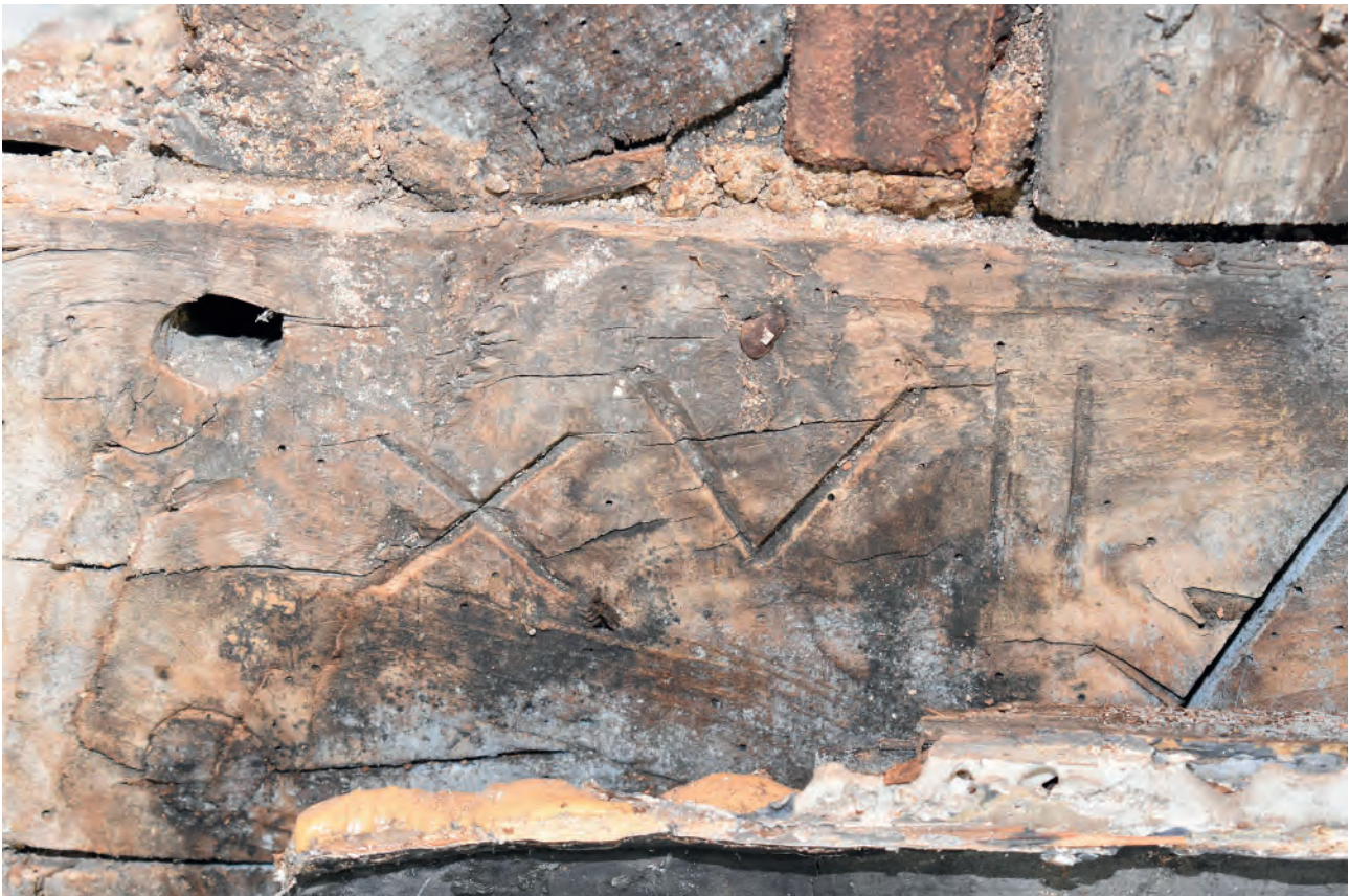
Plate 58: Carpenters' mark on the first floor of No. 7
