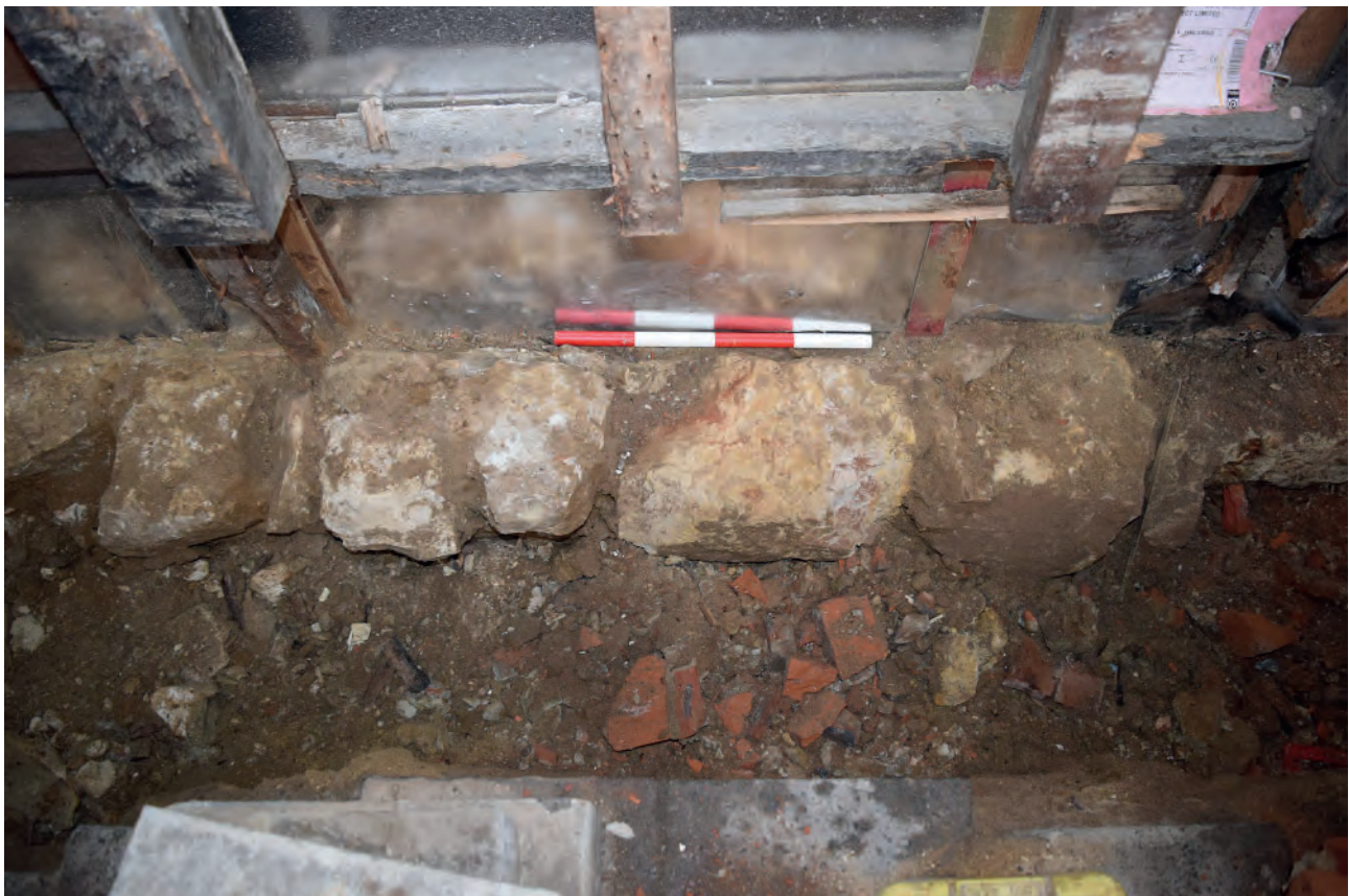
Plate 14: Stone plinth of Nos. 1-2
