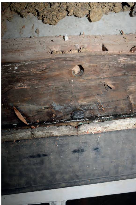
Plate 61: Peg hole and mortise above first floor south window of No. 7
