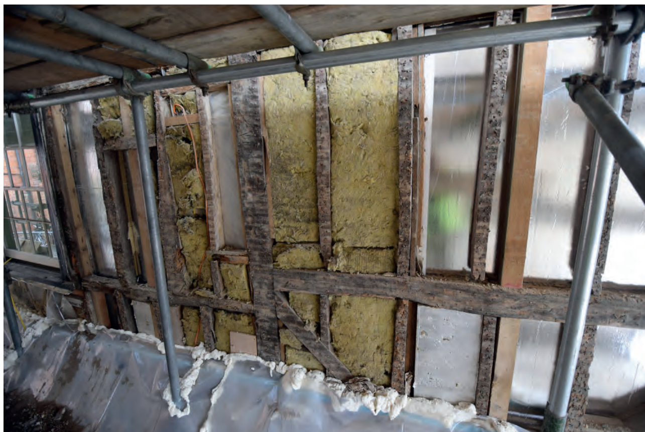
Plate 22: East elevation of Nos. 1-2 at first floor level
