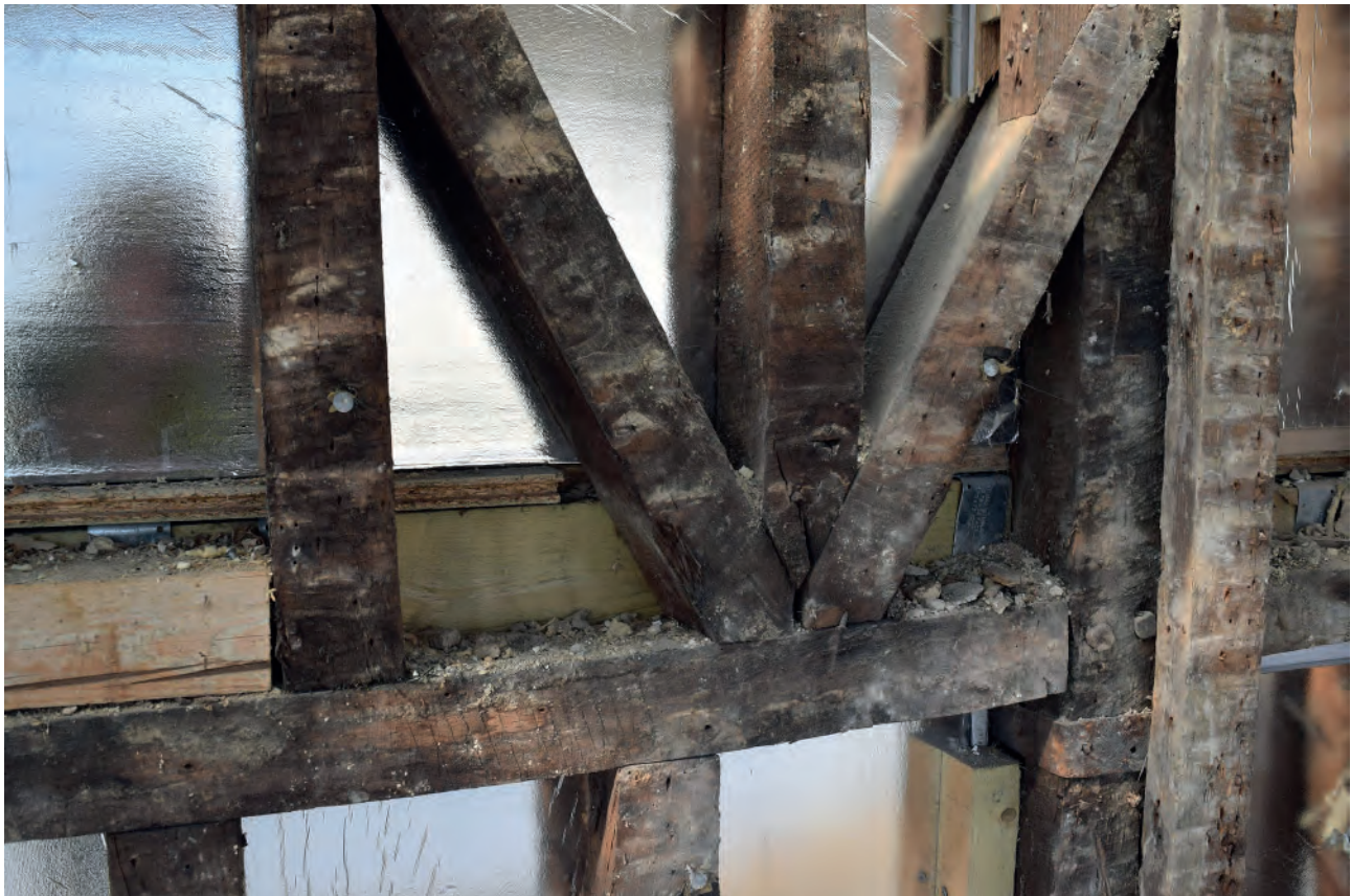
Plate 38: Bracing on the first floor of No. 4
