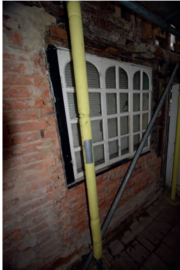
Plate 23: Brickwork on the western half of the ground floor on Nos. 1-2
