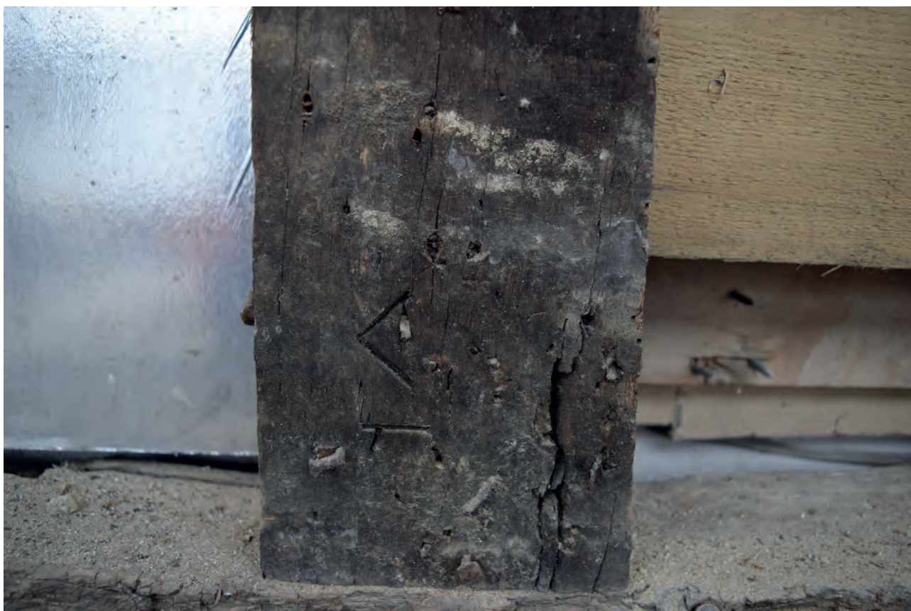
Plate 4: Carpenters' mark on the east elevation of Nos. 1-2 at first floor level
