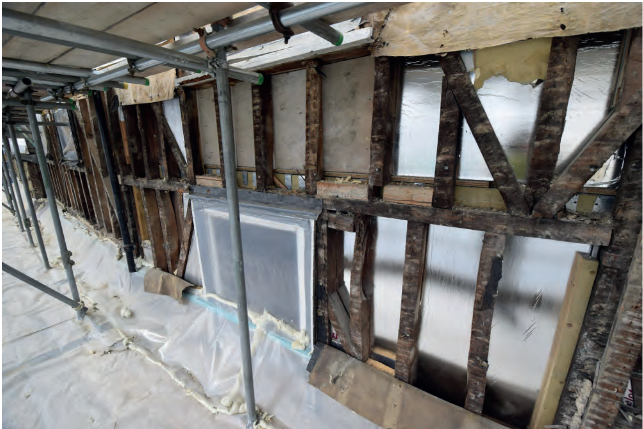
Plate 37: First floor of No. 4
