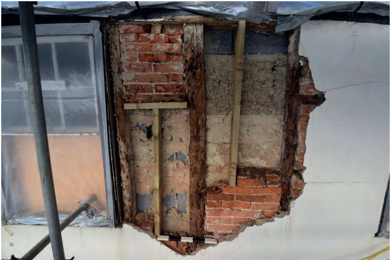
Plate 59: Brick panels on the second floor of No. 7
