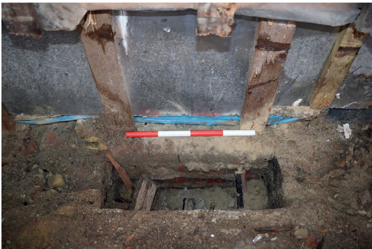
Plate 16: Blocked probable coal chute of Nos. 1-2
