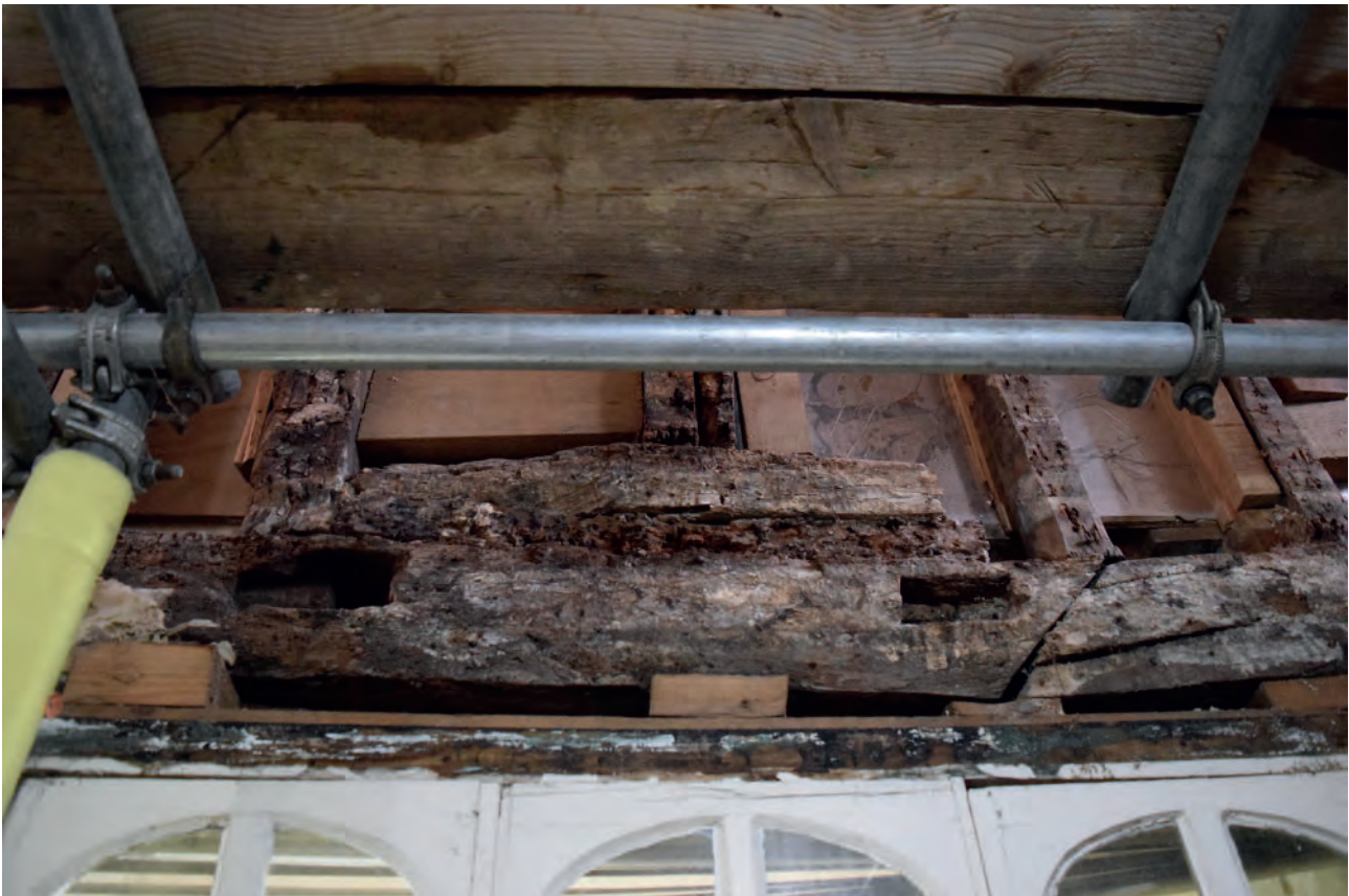
Plate 24: Scarf joint and mortices above ground floor window of Nos 1-2
