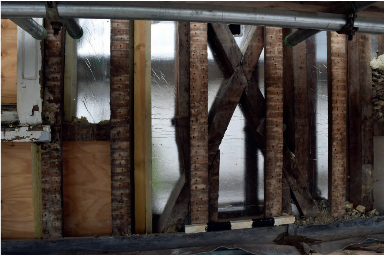
Plate 36: Cross brace on first floor of Nos. 5-6
