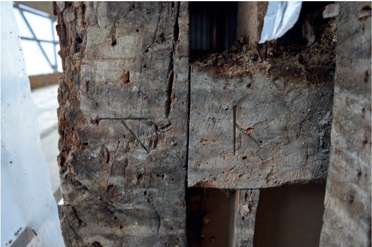
Plate 6: Pair of carpenters' marks on the north elevation of Nos. 1-2 at first floor level
