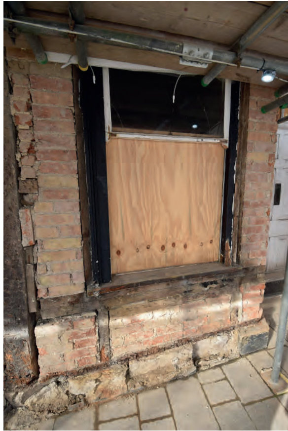
Plate 41: Brick nogging on the ground floor of No. 4
