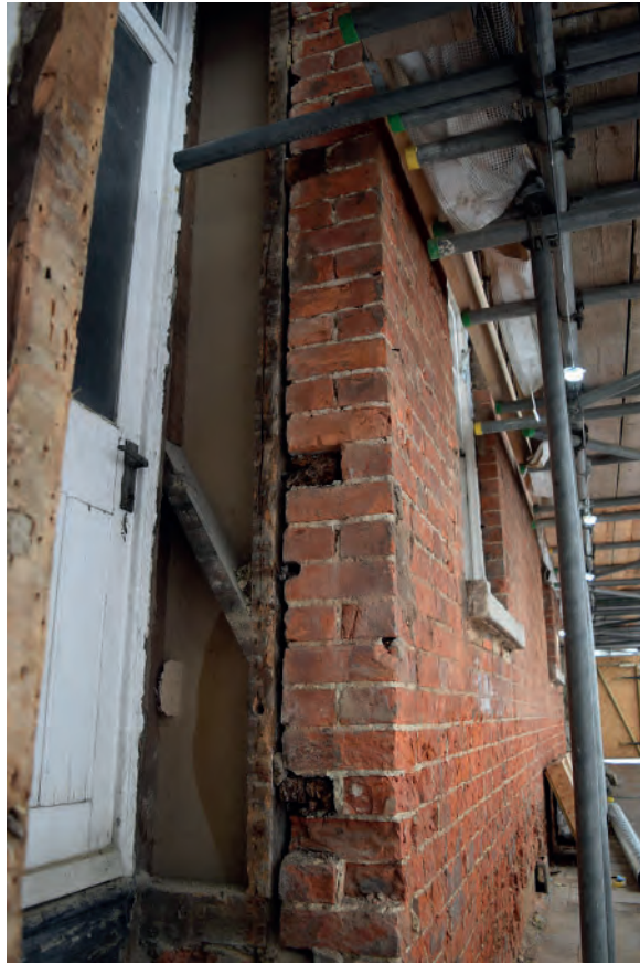
Plate 51: Framing behind the brick reface of Nos. 5-6
