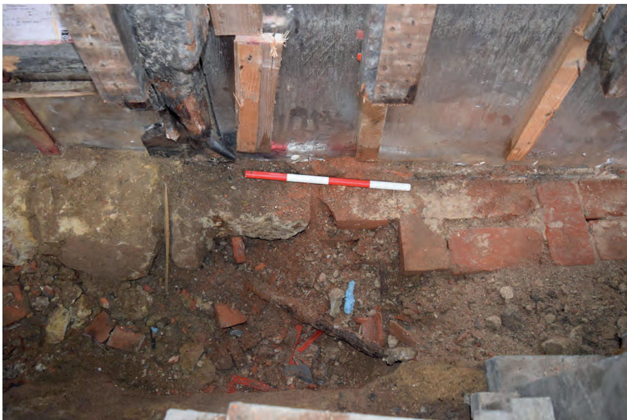
Plate 15: Secondary brick plinth on the northern side of Nos. 1-2
