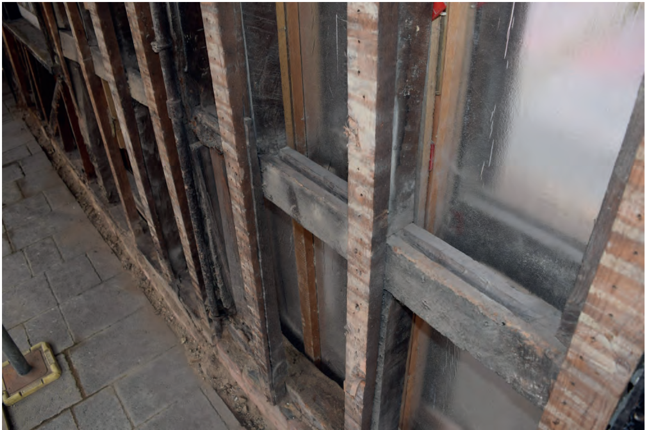
Plate 13: Refacing on the ground floor of Nos. 1-2
