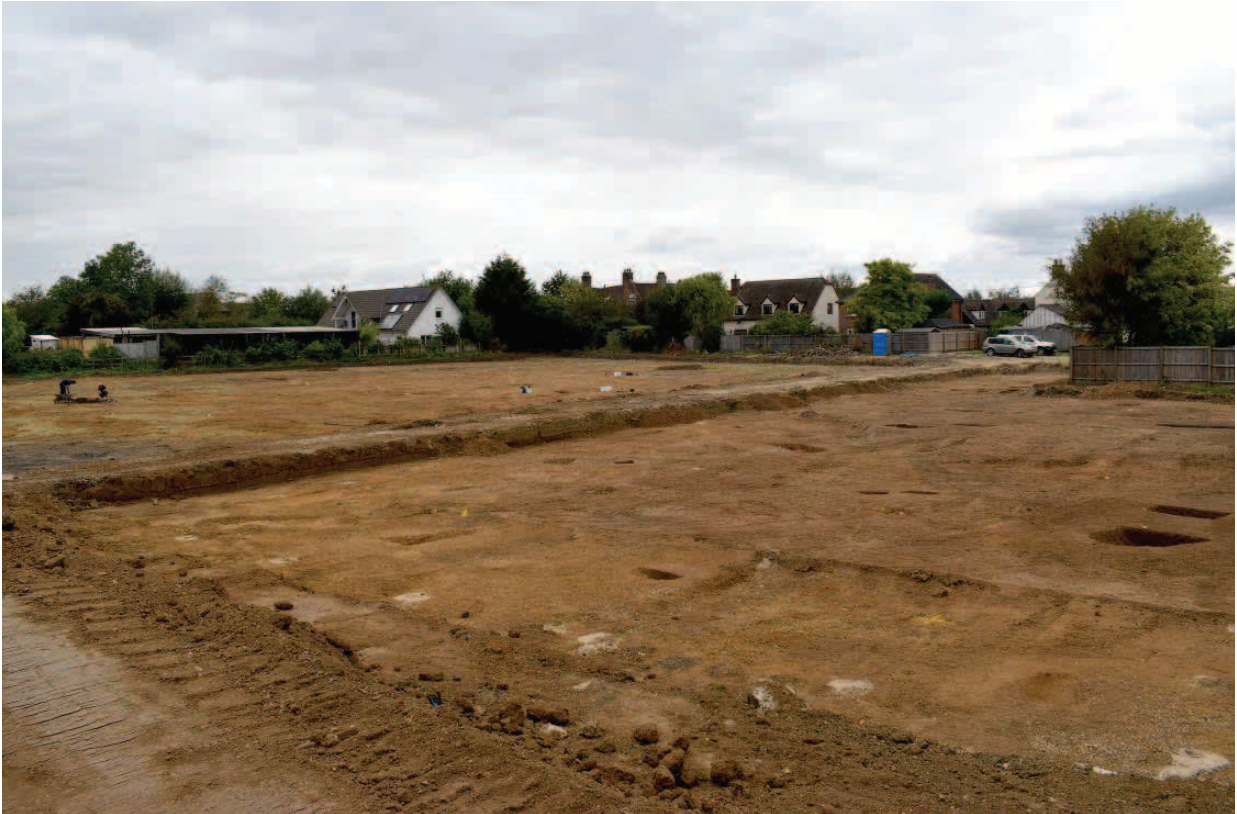
Plate 2: View of the site from the north-east
