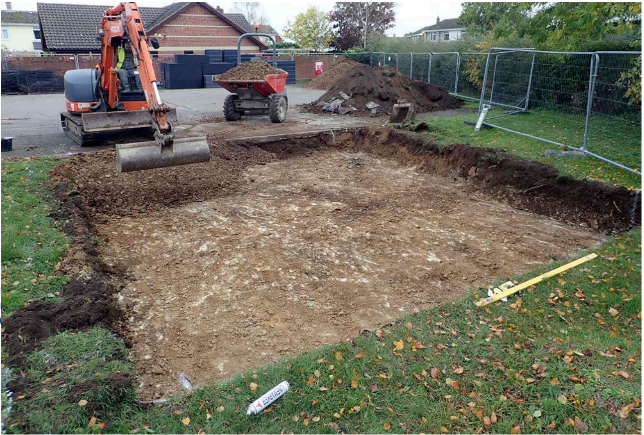
Plate 1: Area strip for soak-away
