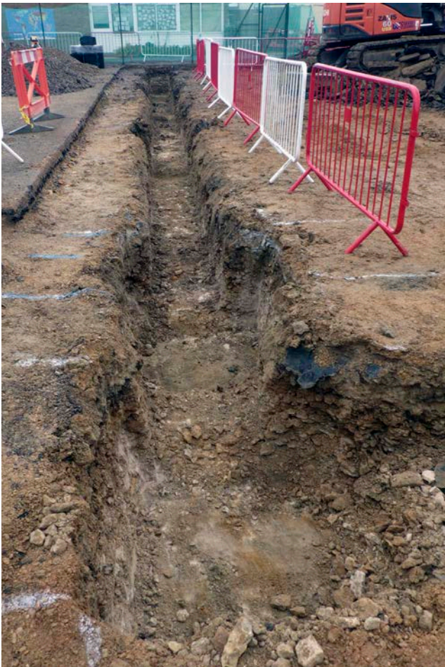
Plate 2: Foundation trench
