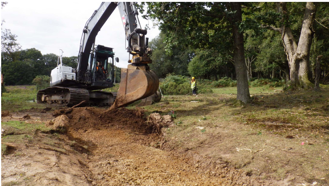
Plate 1: OA 27, work near possible mound, looking south-west
