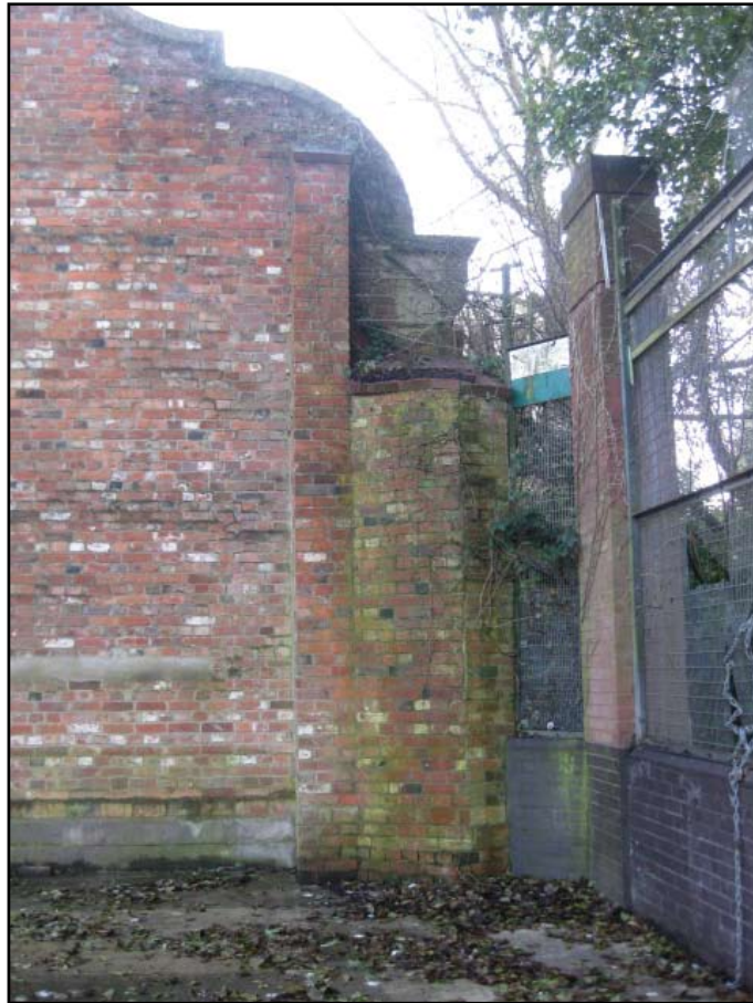
Plate 6: Buttress and corner pier on north face of gable wall
