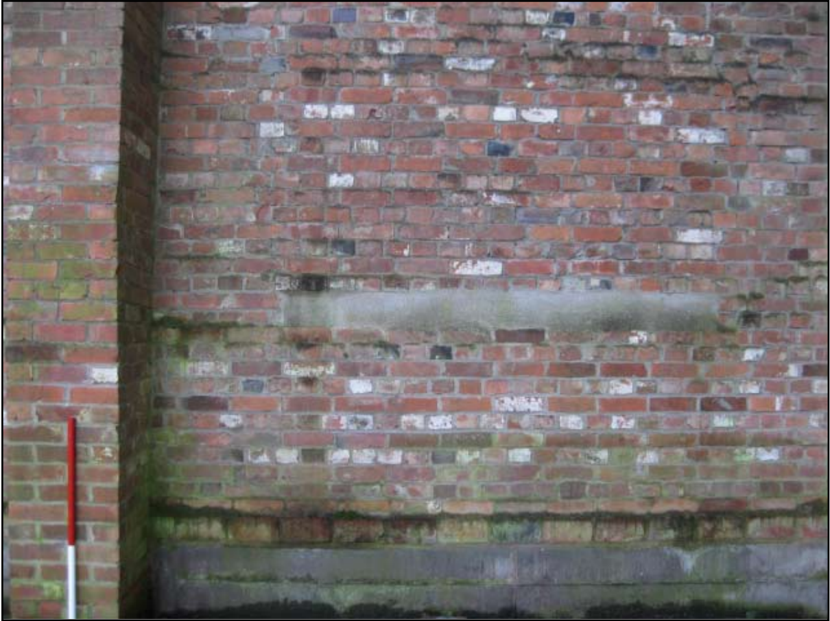
Plate 5: Buttress and plinth on north face of gable wall
