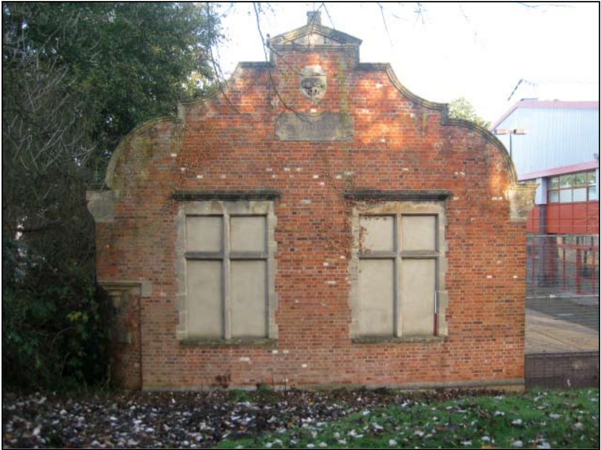
Plate 1: South face of gable wall
