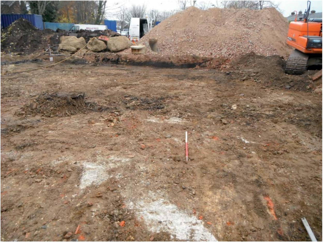
Plate 3: General view of ground reduction
