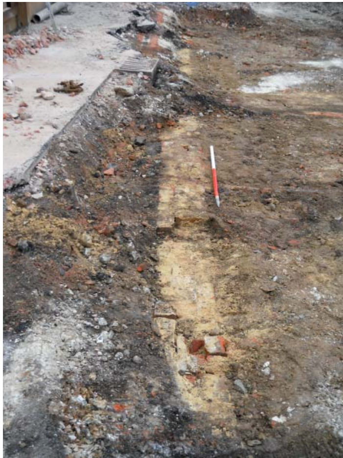
Plate 2: Eastern edge of site: Wall footing 107
