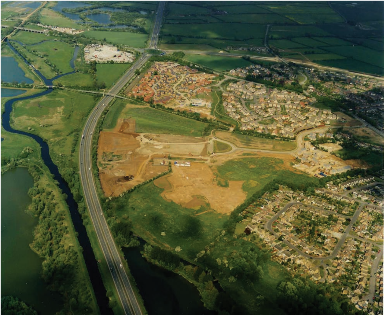
Plate 5.8 Aerial view of development area after the Saxon and medieval excavations, looking north-west (Duchy of Lancaster copyright)
