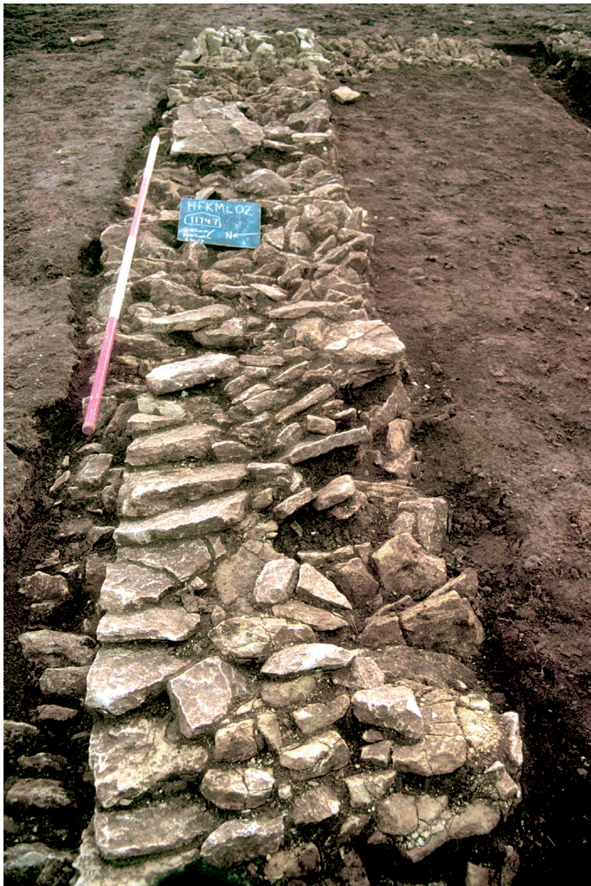
Plate 4.6 Building 11620, north wall 11747, facing east. Note the manner in which the outer face of the wall is set back from the outer face of the foundation. Scale: 2 m
