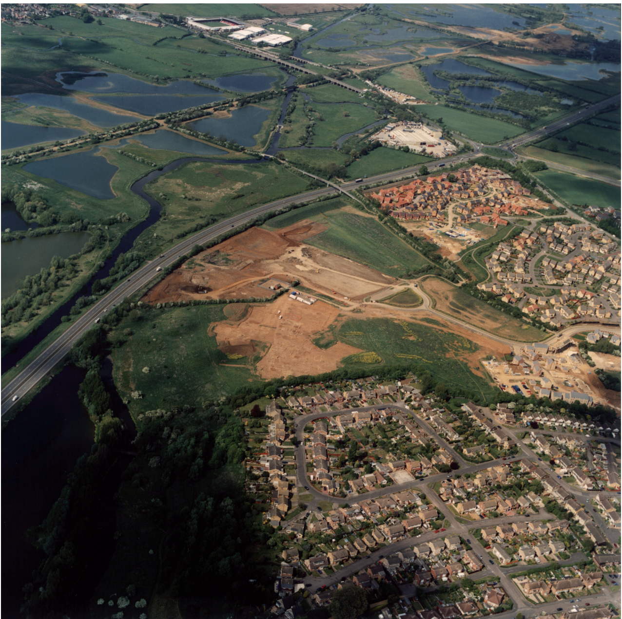
Plate 1.2 Aerial photograph of Higham Ferrers site during 2002/3 excavations on the Roman settlement (© Duchy of Lancaster)
