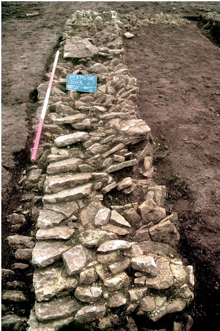
Plate 4.6 Building 11620, north wall 11747, facing east. Note the manner in which the outer face of the wall is set back from the outer face of the foundation. Scale: 2 m
